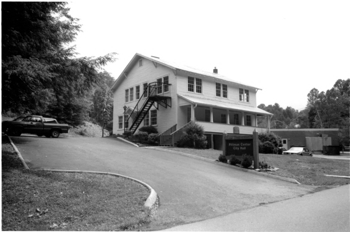
Pittman Community Center Home Economics Building Sevier Co. TN
