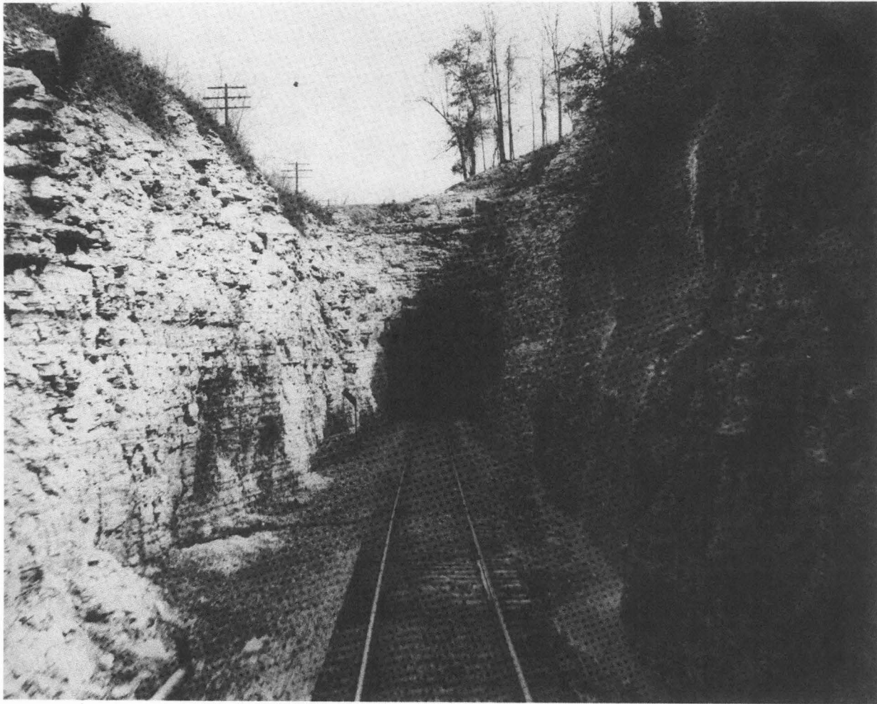
Cotter Tunnel Northwest Portal (c.1943)
