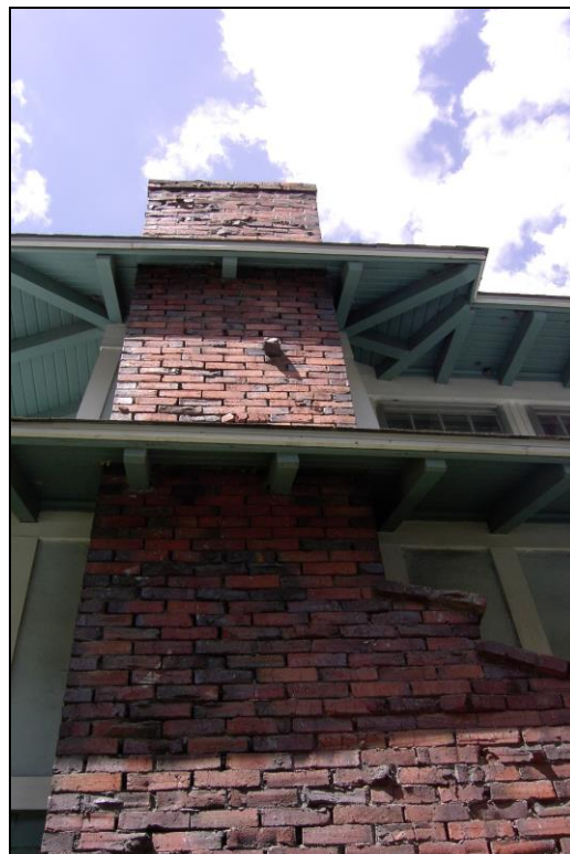
WA_Spokane County_Seligman House_0005.tiff Clinker brick chimney on south face of Seligman House
