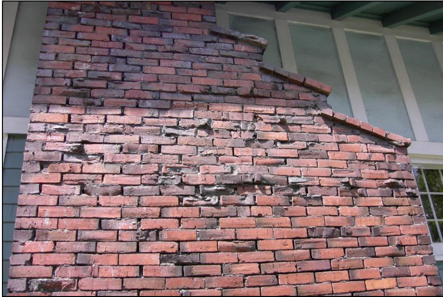
WA_Spokane County_Seligman House_0006.tiff Clinker brick chimney detail on south face of Seligman House
