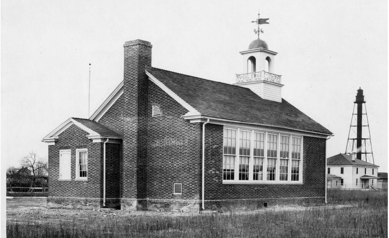
Figure 8: Taylor's Bridge School, rear elevation, circa 1925. (Image courtesy of the Hagley Museum: Delaware School Auxiliary Association)
