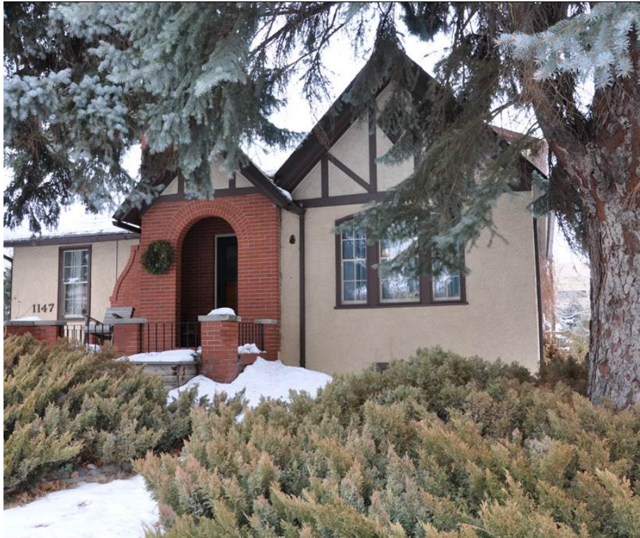
MT_Yellowstone County_North ElevationHD_0032: 1147 N. 31 st Street, view to the northeast.
