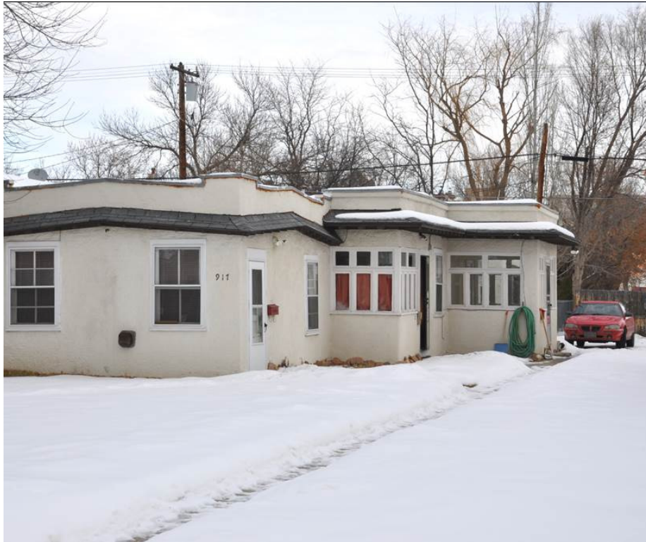
MT_Yellowstone County_North ElevationHD_0031: 917 N. 31 st Street, view to the northeast.
