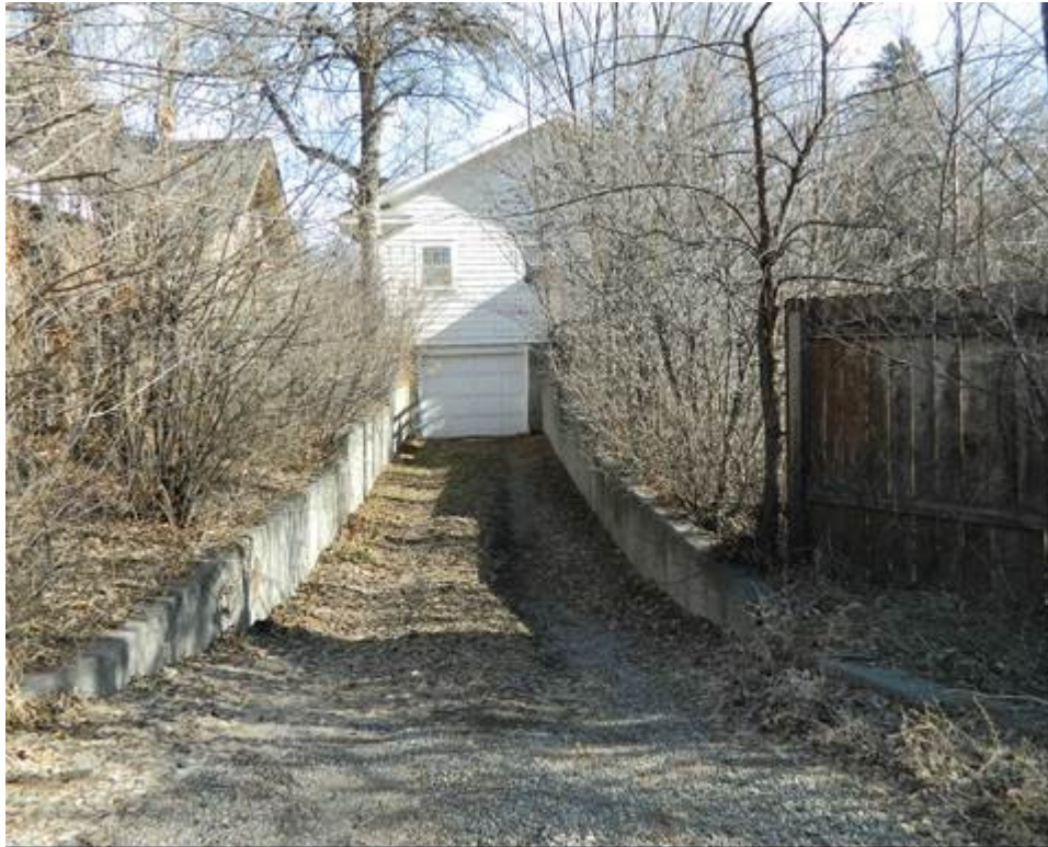
MT_Yellowstone County_North ElevationHD_0044: 1130 N. 31st Street, showing garage as part of principle structure, view to the east.
