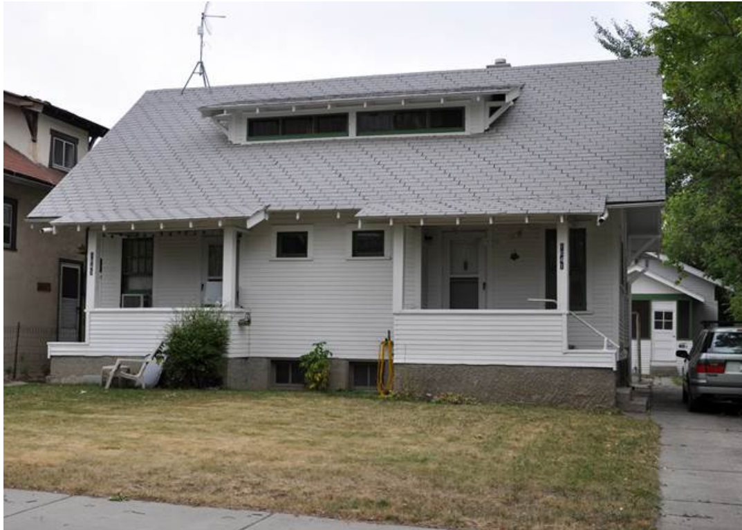
MT_Yellowstone County_North ElevationHD_0004: 1041 and 1043 N. 31 st Street, view to the northeast.
