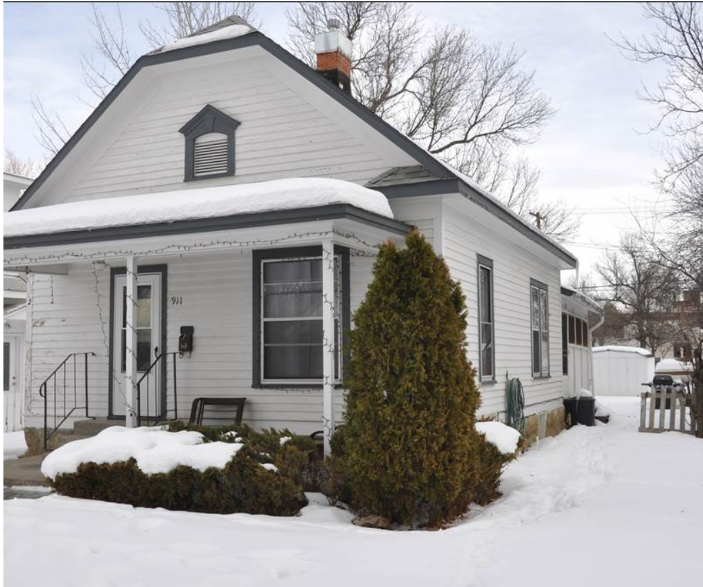
MT_Yellowstone County_North ElevationHD_0020: 911 N. 31 st Street, view to the east.
