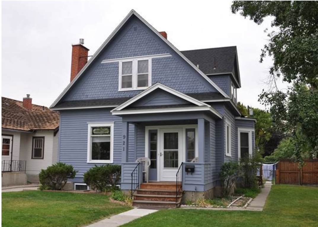
MT_Yellowstone County_North ElevationHD_0030: 921 N. 31 st Street, view to the east.
