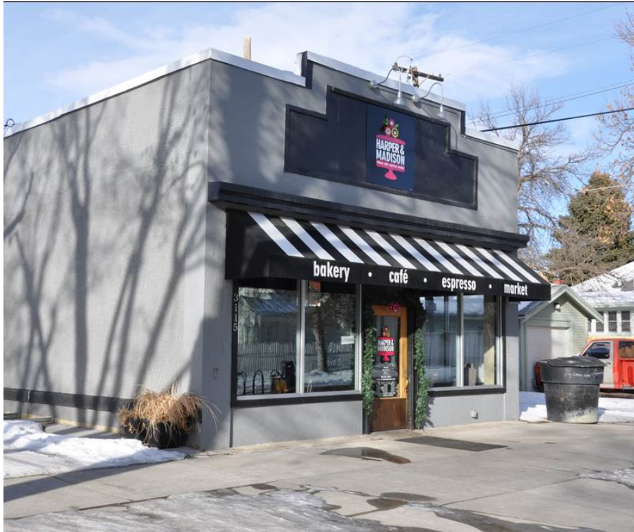
MT_Yellowstone County_North ElevationHD_0034: 3115 10th Ave. North, view to the northeast.
