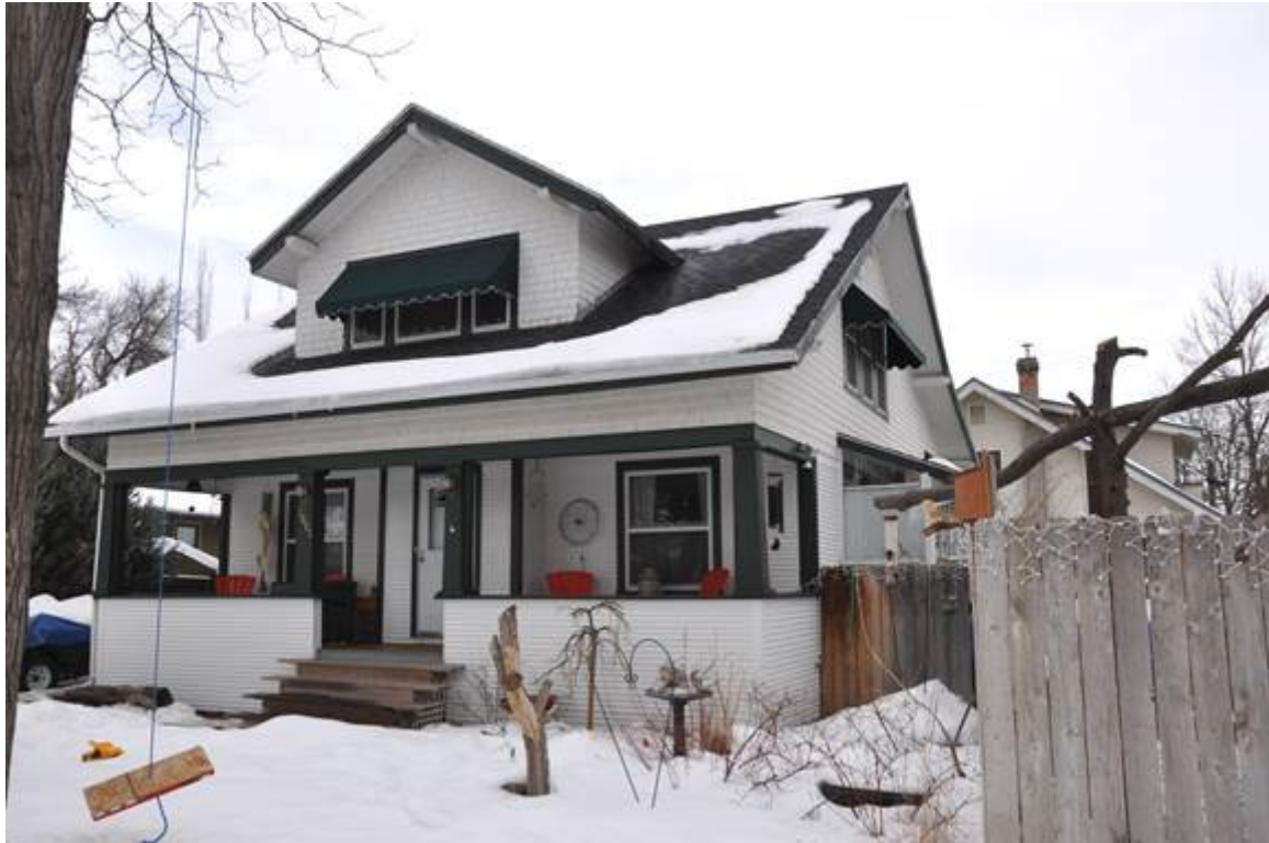
MT_Yellowstone County_North ElevationHD_0003: 1001 N. 31 st Street, view to the northeast.
