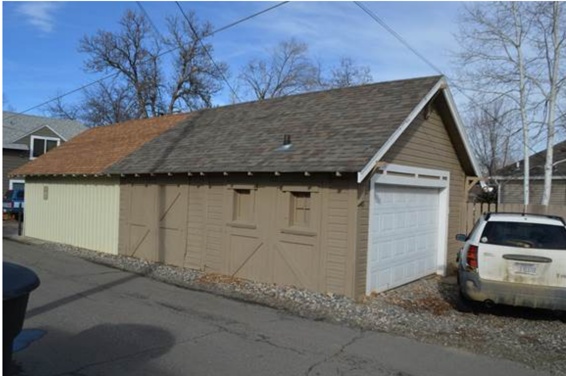
MT_Yellowstone County_North ElevationHD_0046: 910 N. 31st Street, garage, view to the northeast.
