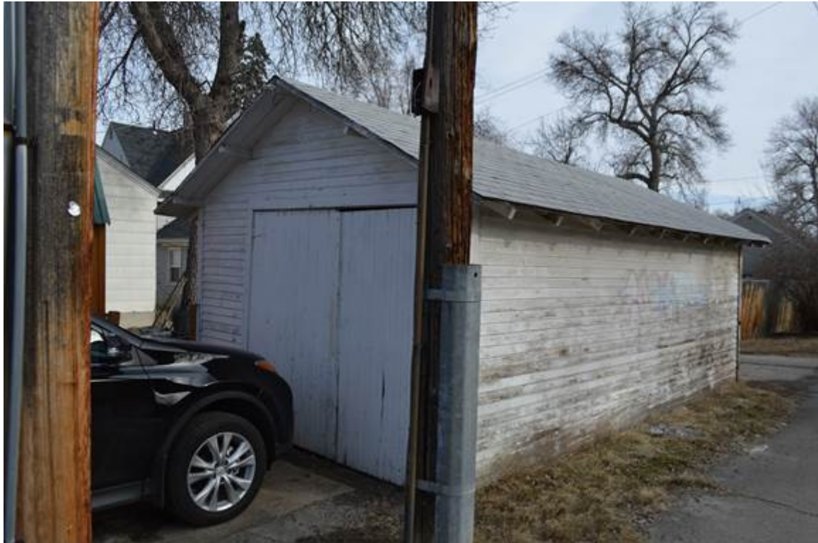
MT_Yellowstone County_North ElevationHD_0045: 946 N. 31st Street, garage, view to the southeast.
