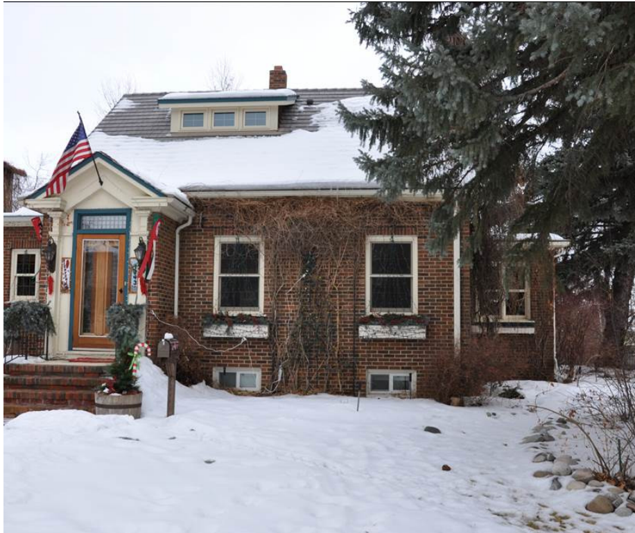
MT_Yellowstone County_North ElevationHD_0023: 1143 N. 31 st Street, view to the east.
