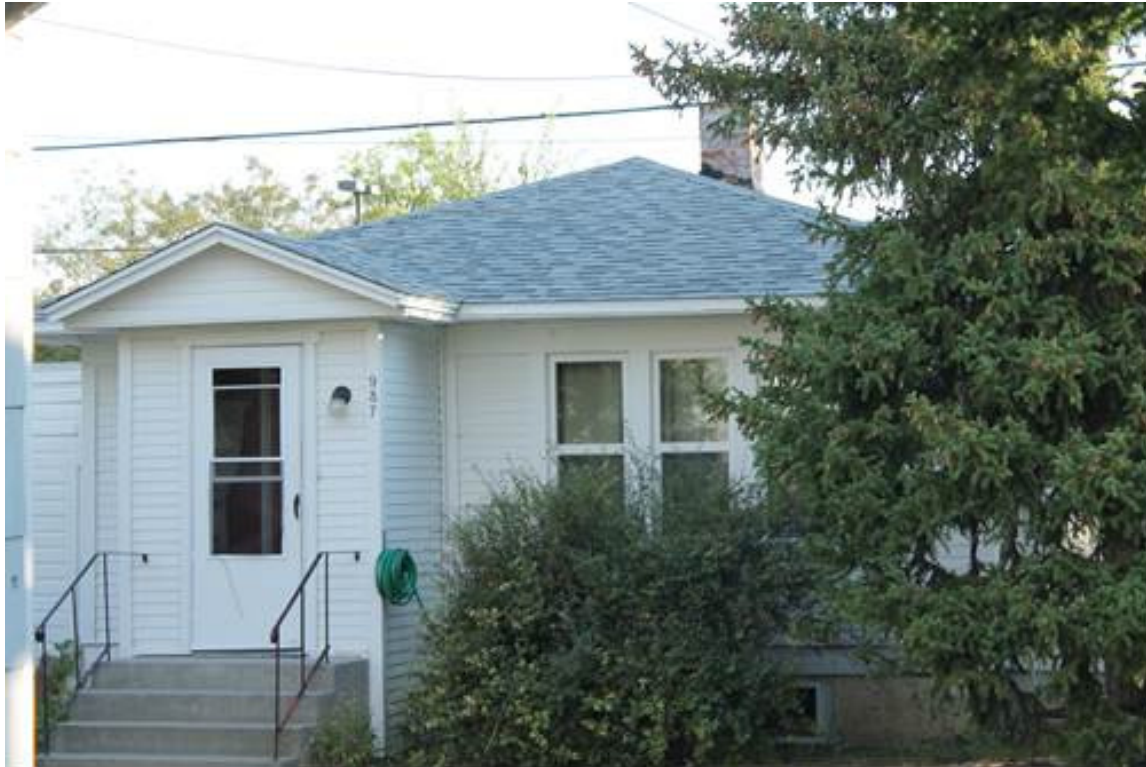
MT_Yellowstone County_North ElevationHD_0015: 937 N. 31 st Street, view to the northeast.
