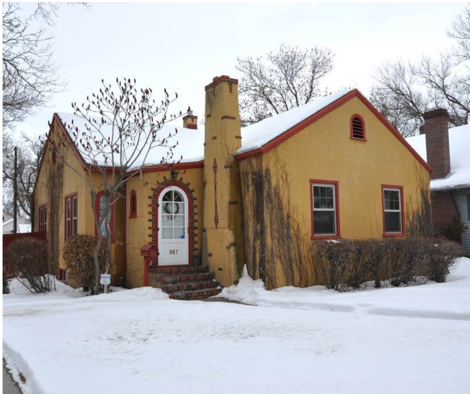
MT_Yellowstone County_North ElevationHD_0010: 947 N. 32 nd Street, view to the northeast.
