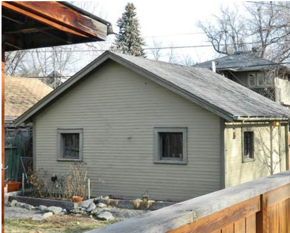
MT_Yellowstone County_North ElevationHD_0041: 1105 N. 32nd Street, showing garage, view to the east.
