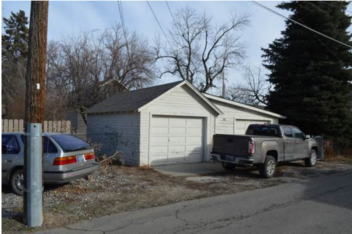
MT_Yellowstone County_North ElevationHD_0047: 906 N. 31st Street, garage, view to the southeast.
