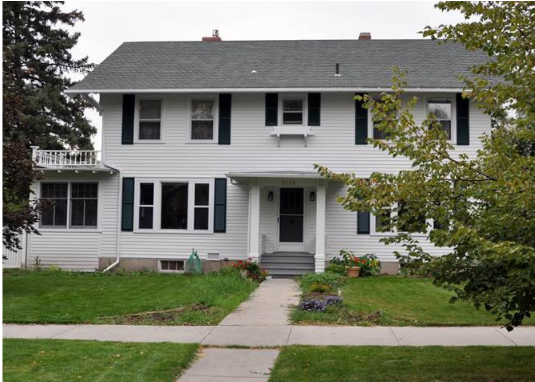
MT_Yellowstone County_North ElevationHD_0026: 1024 N. 31 st Street, view to the southeast.
