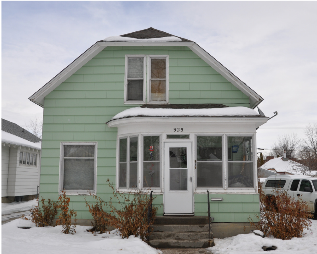
MT_Yellowstone County_North ElevationHD_0019: 925 N. 31 st Street, view to the east.
