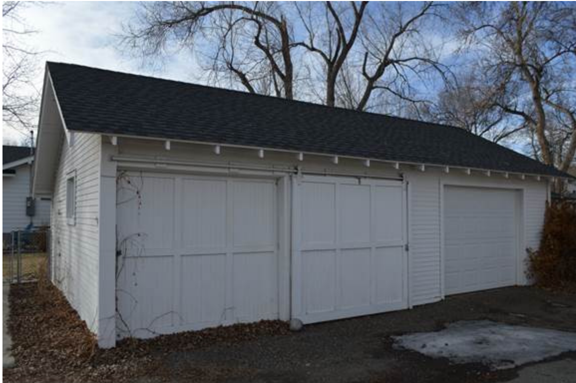
MT_Yellowstone County_North ElevationHD_0042: 931 N. 32nd Street, garage, view to the northwest.
