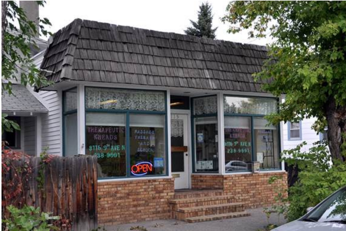
MT_Yellowstone County_North ElevationHD_0035: 3115 9 th Ave. North, view to the northeast.
