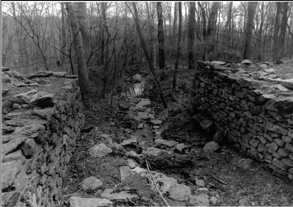
Photo 6 of 40 Waste Weir-Spillway (NR#39), view E
