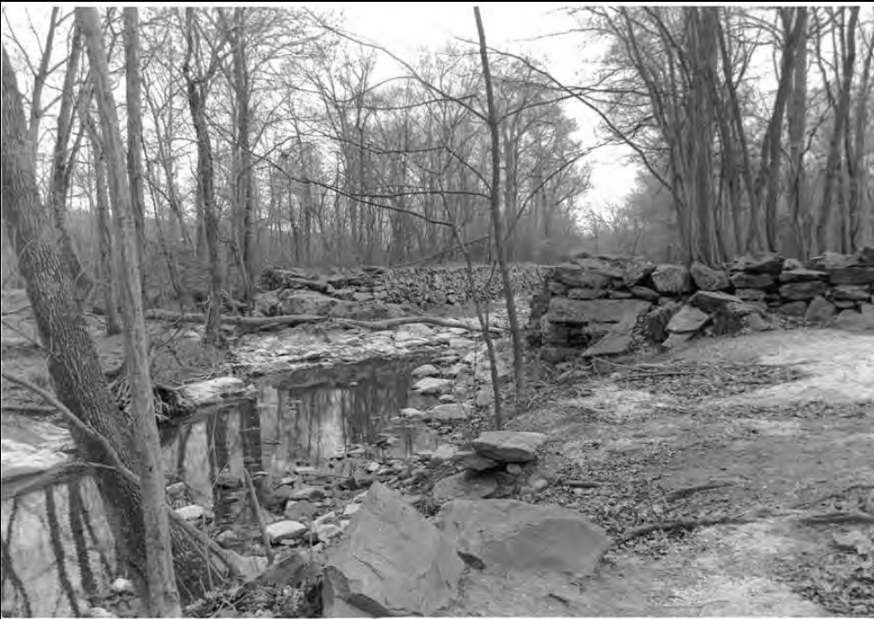
Photo 4 of 40 Upper Canal Wall and Bed of Canal (NR#31), view SE at Upper Guard Gate
