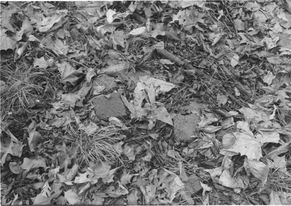
Photo 30 of 40 Detail of Worker's Barracks brick fall (NR#22)
