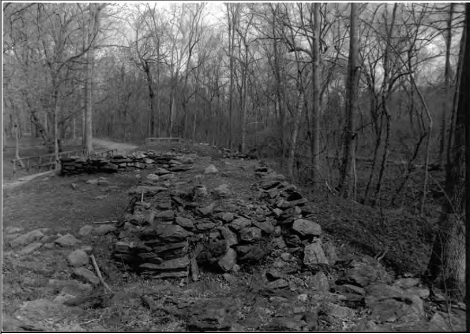
Photo 9 of 40 Collecting Basin Wall SE corner (NR#37), Sawmill Foundation, view N
