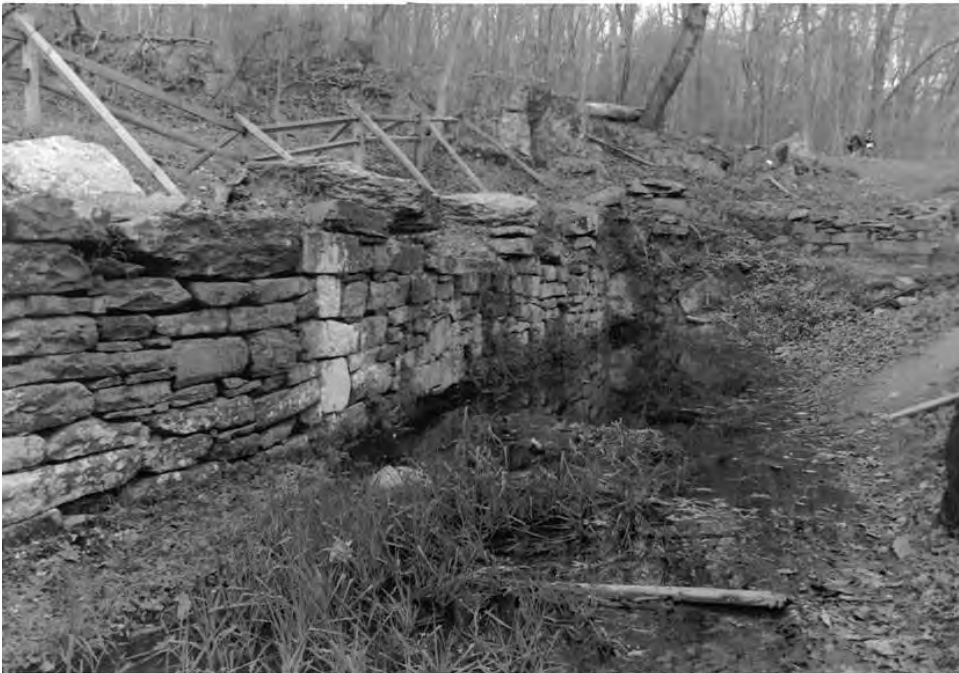
Photo 20 of 40 East Wall Detail, Middle Canal Long Wall (NR#32)
