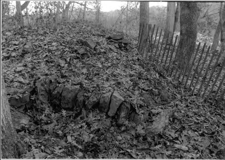
Photo 15 of 40 Canal Works (NR#46), East of Locks 2 & 3, Stone Ramp, View E
