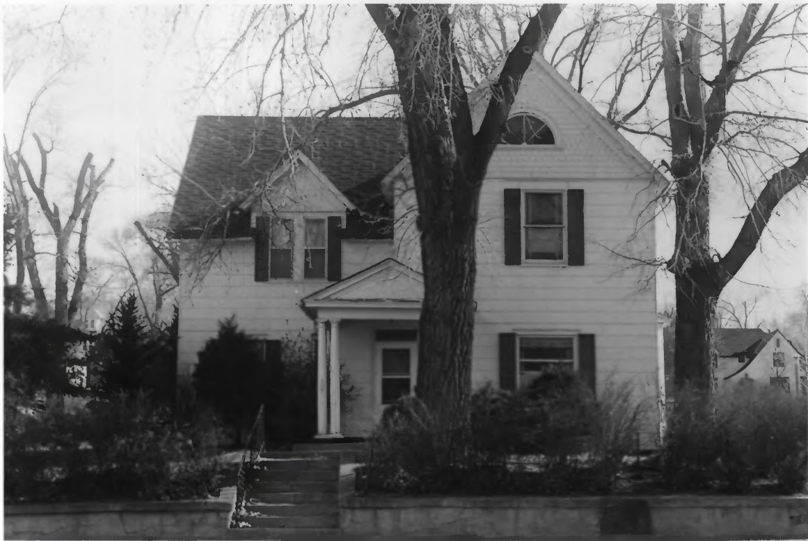
Horner/Hyde House , Hughes County, South Dakota, No. 1
