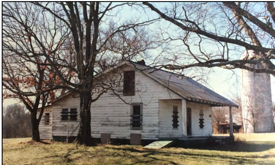
Figure 17: Tenant House in 1990. Photo from Clover Bottom File, Tennessee Historical Commission.
