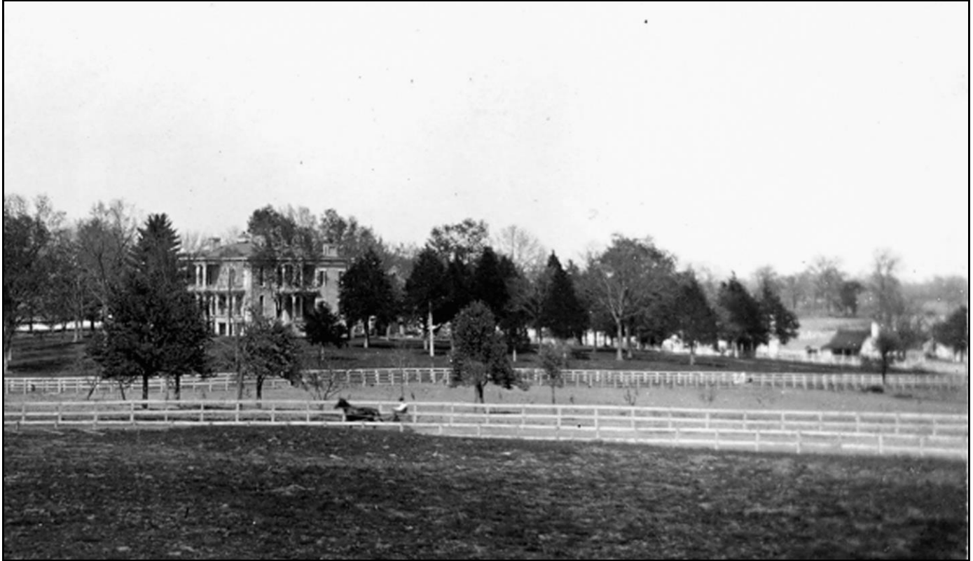
Figure 25: Clover Bottom Horse Track with Mansion and Slave/Tenant Dwellings visible at rear, ca. 1900. Digital File in Clover Bottom File, Tennessee Historical Commission.
