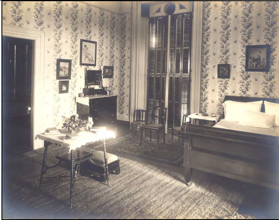
Figure 14: Bedroom at Northeast Corner of Second Level. View to the northwest, ca. 1917. Photo from Clover Bottom File, Tennessee Historical Commission.
