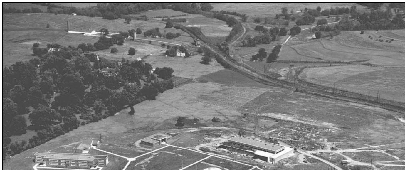
Figure 34: Aerial Photo of the Tennessee School for the Blind under construction in 1952 with Clover Bottom Farm behind. Image #15279 from Tennessee State Library and Archives.
