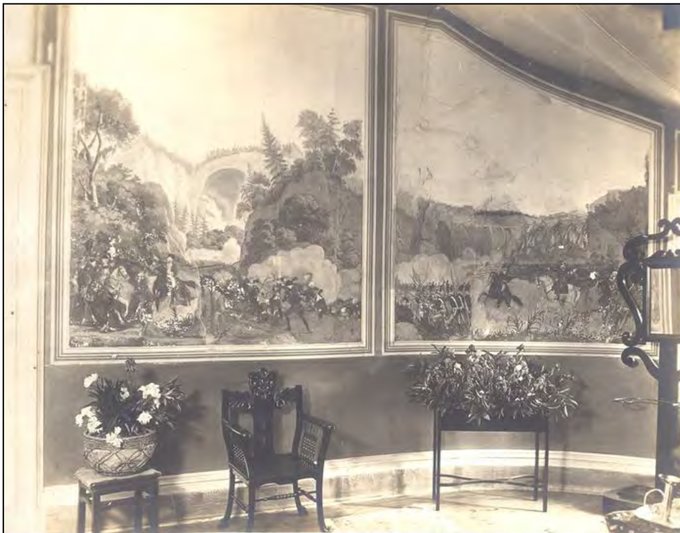
Figure 5: Close-up of Wallpaper below Stairs in First Level Hall, ca. 1917. Photo from Clover Bottom File, Tennessee Historical Commission.
