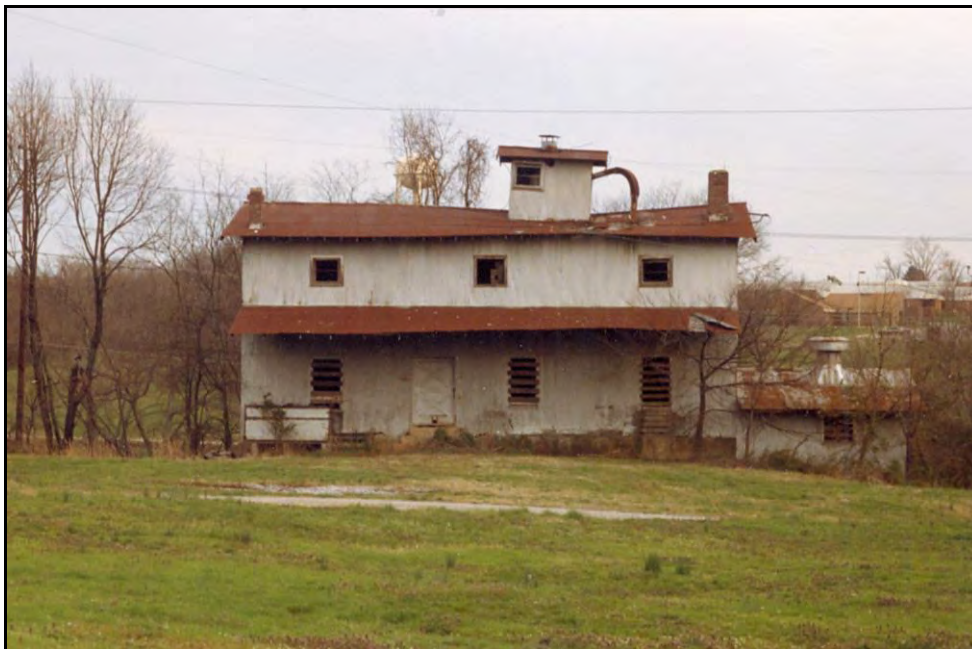
Figure 18: Feed Mill in 1990. Photo from Clover Bottom File, Tennessee Historical Commission.
