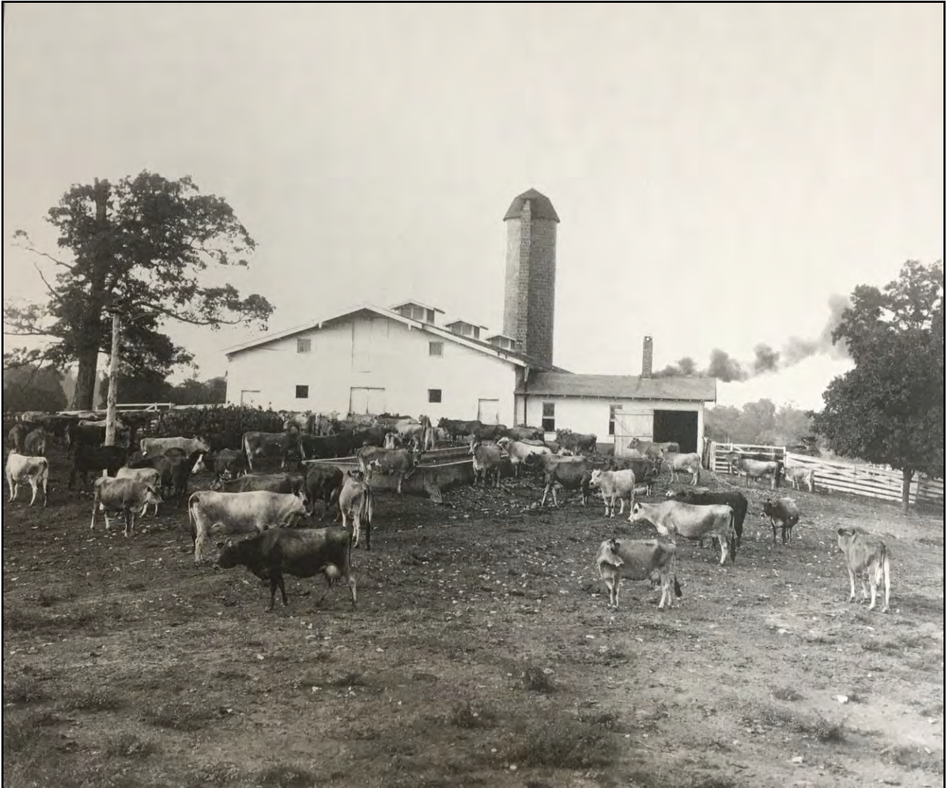
Figure 31: Dairy Barn and Silo constructed by the Stanfords, ca. 1930. Clover Bottom File, Tennessee Historical Commission.
