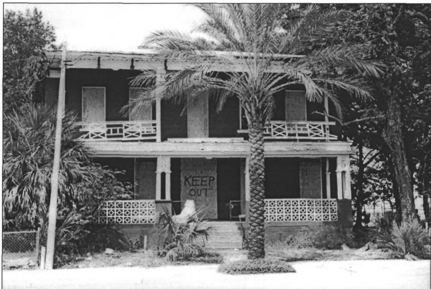
PHOTO #1, Brewster Hospital—Front, Existing Condition at Original Site
