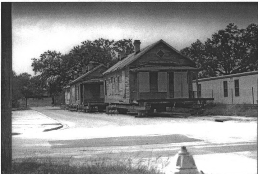
PHOTO #13, Shotgun Houses, Houses Ready to Be Moved to La Villa Experience Site.
