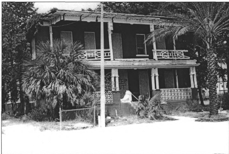
PHOTO #2, Brewster Hospital—Angle Shot, Existing Condition at Original Site
