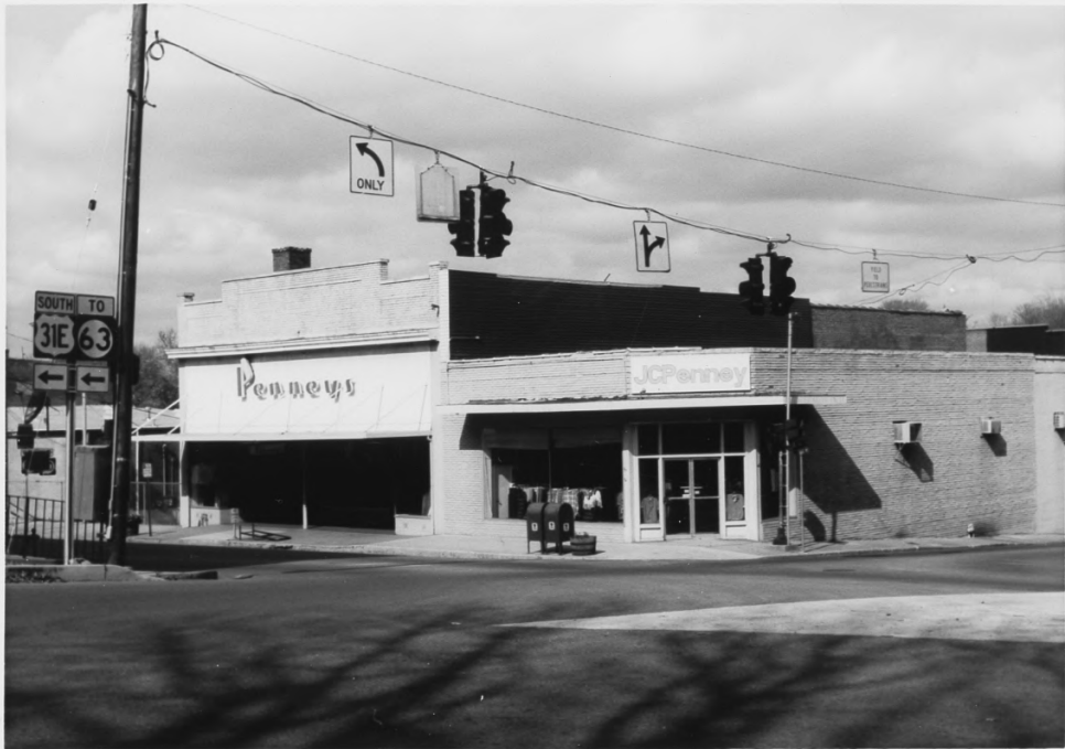
207 West Main Glasgow Central Business District Barren County, Kentucky
