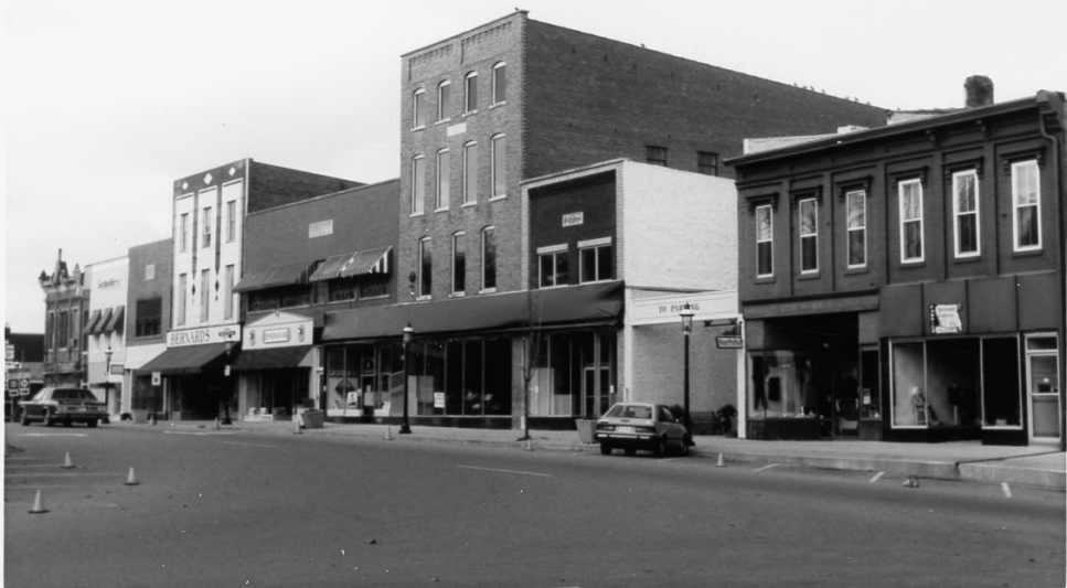
107-143 West Main Glasgow Central Business District Barren County, Kentucky #4
