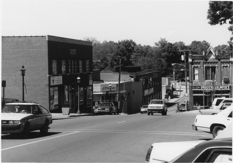
207 W. Main, 109 N. Race, 143 W. Main Glasgow Central Business District Barren County, Kentucky #3
