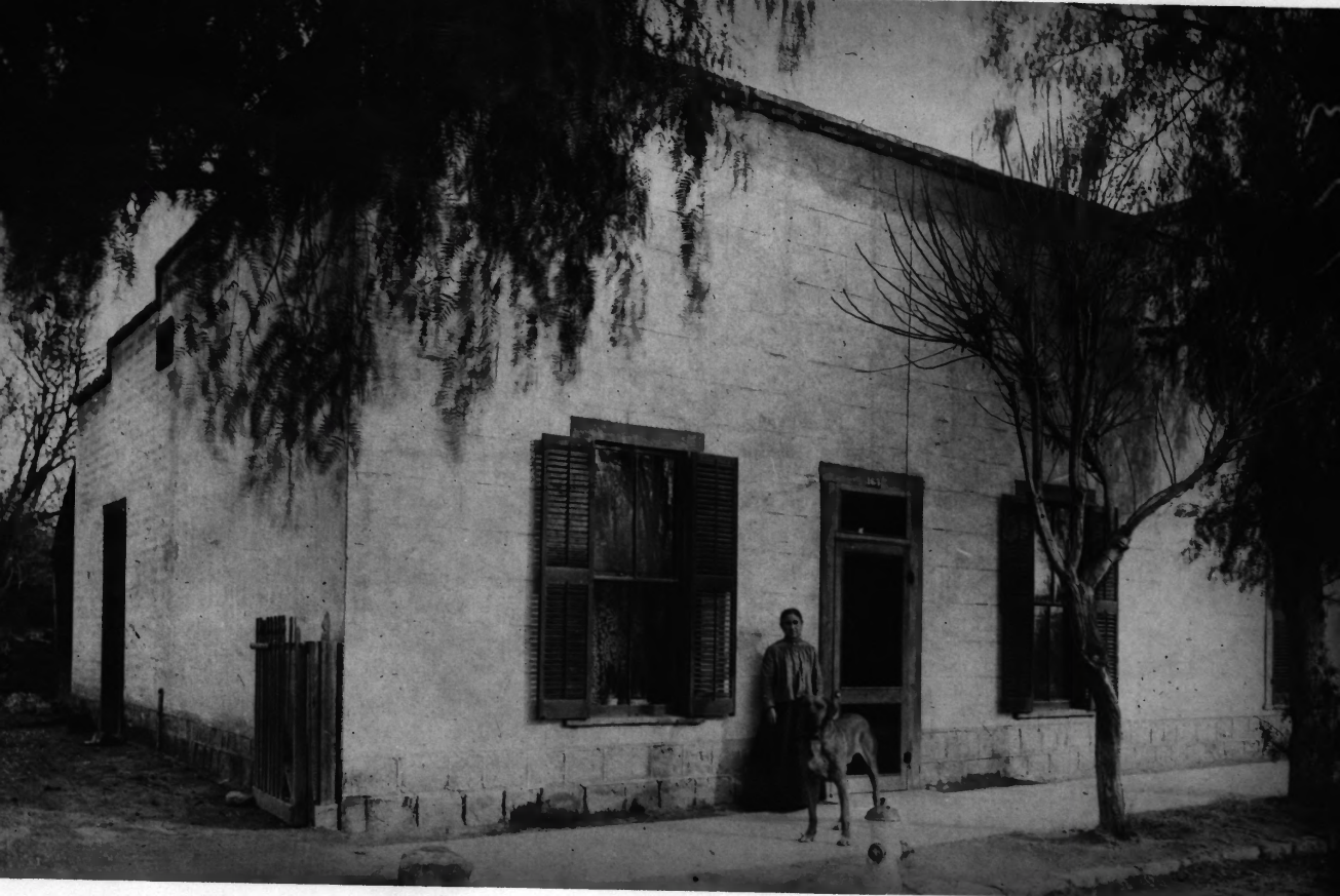
Note: Just the front portion of the house is stuccoed and that is meant to resemble stone, or perhaps for the effect. Wood trim o ver the door and windows.
