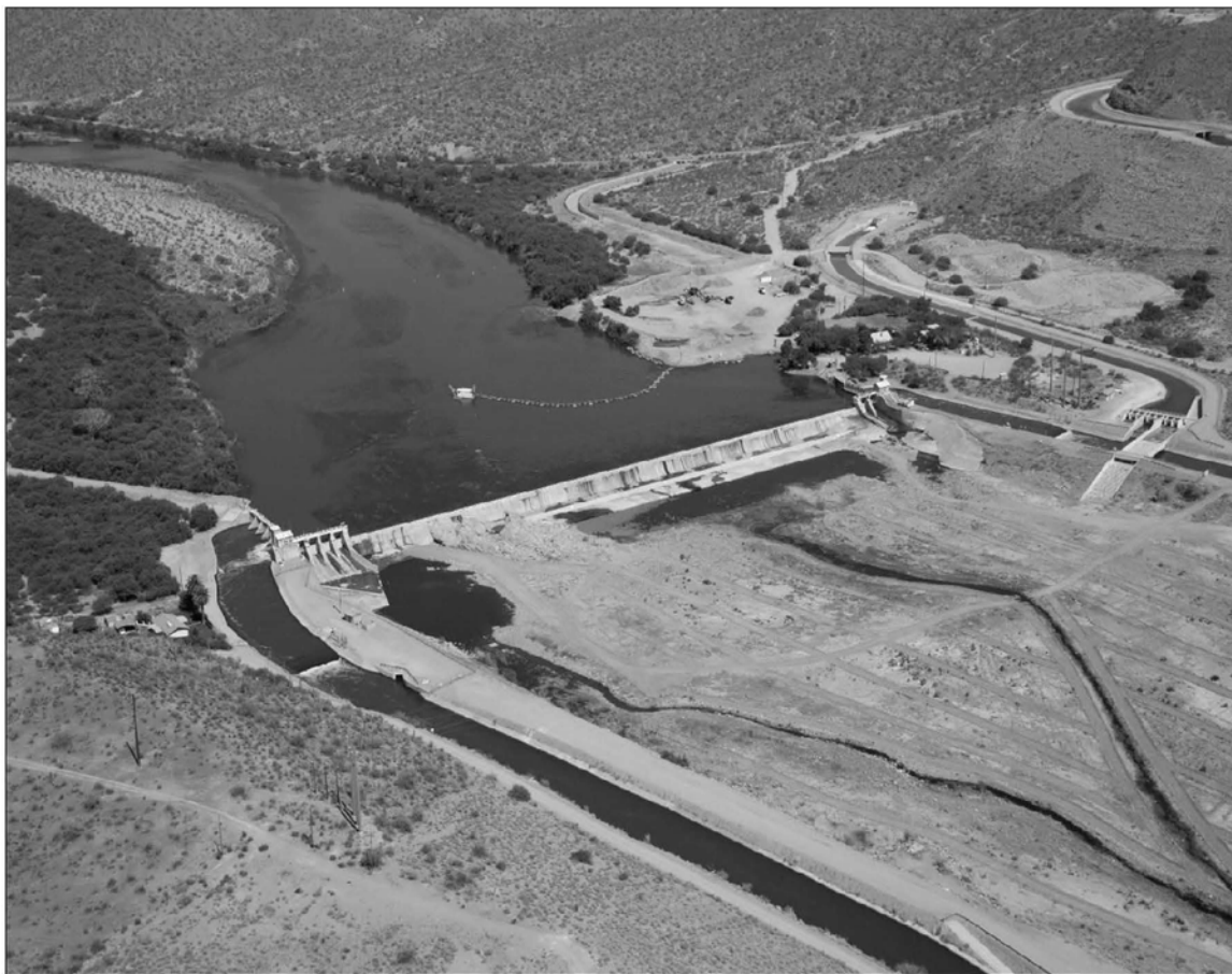
Photo J7: Aerial photo of Granite Reef Diversion Dam. Arizona Canal headworks at center left; South Canal headworks at center right; Southside Gatekeeper's House at center right near South Canal heading. Photo courtesy SRP.
