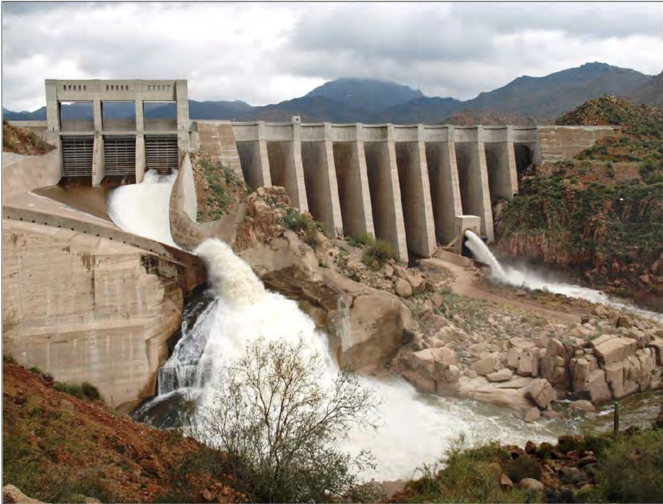
Photo J4: Bartlett Dam on the Verde River, spring 2010. The lighter grey areas atop each of the curved buttresses indicate where the dam was raised 21.5 feet in the 1990s. Photo courtesy of the Bureau of Reclamation, Jim Bailey, photographer
