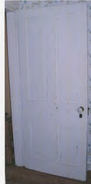
four-paneled, second floor interior door with porcelain knob, electroplated hardware - c. 1850s section
