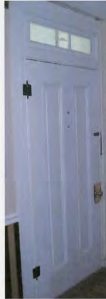
original interior door with flat elongated panels and a three-light transom - c1850s section
