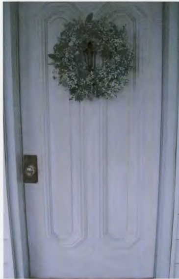
original exterior door with heavily-molded elongated panels - c. 1850s section
