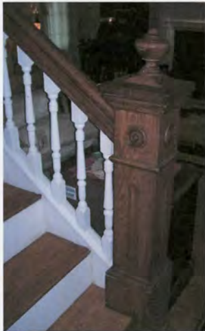
closed-string staircase, molded Handrail, turned balusters, and decorative square newel post - c. 1850s section
