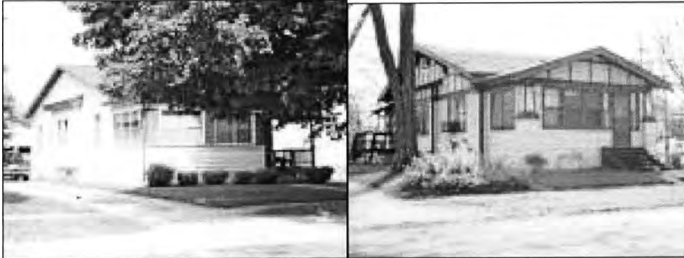
Figure 16: 123 West Washington, 1912 (left), 126 West Adair Street, 1916 (right) (Butler County Assessor)
