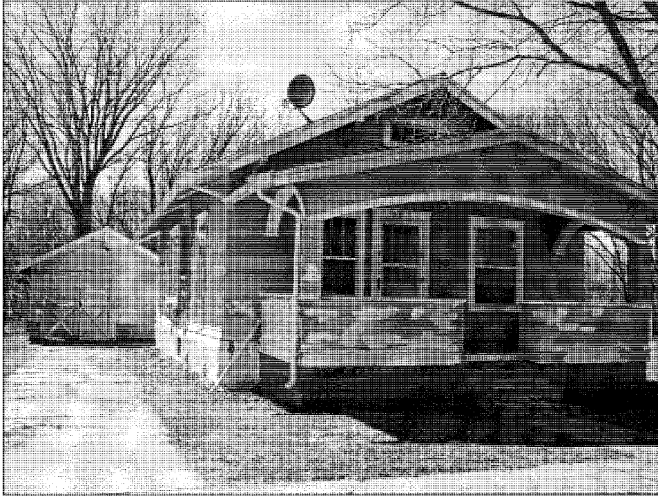
Figure 3: Original location, view west, note garage relationship (photo by Linda McCann, 2006)
