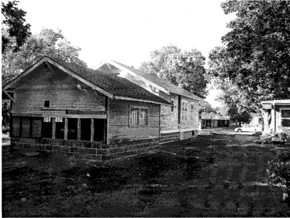
Figure 13: Garage and bungalow on new site, view southeast (photo by Linda McCann, 2006)
