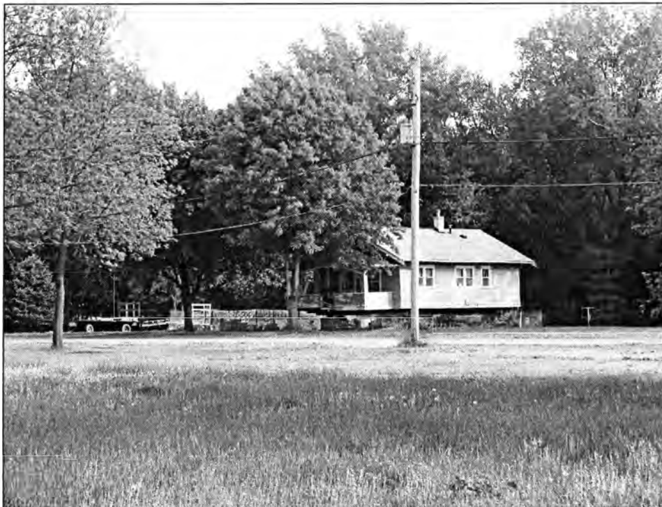
Figure 8: Original site, house suspended alongside foundation, view southwest, overview (photo by Linda McCann, 2006)
