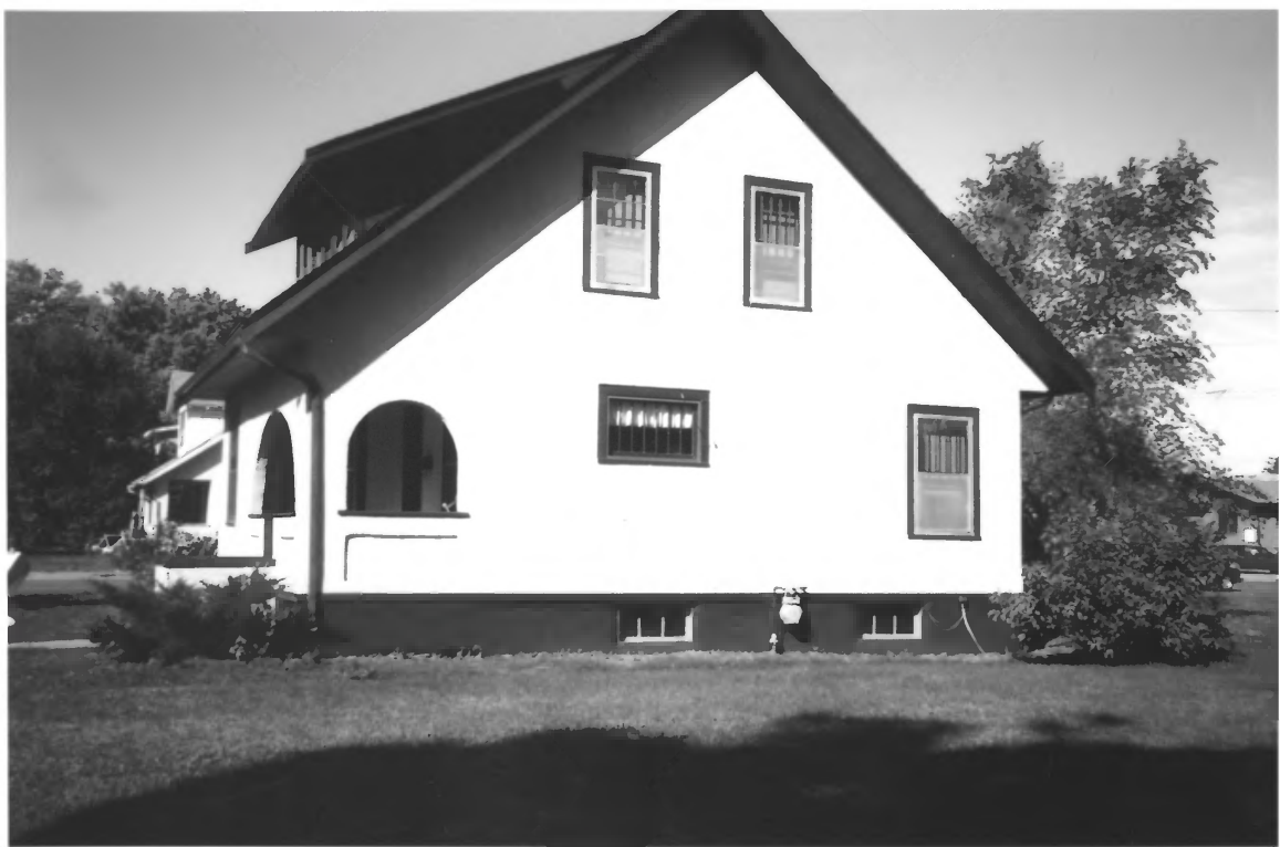
C.E. Chambers House, Davison County, So. Dak., No 3
