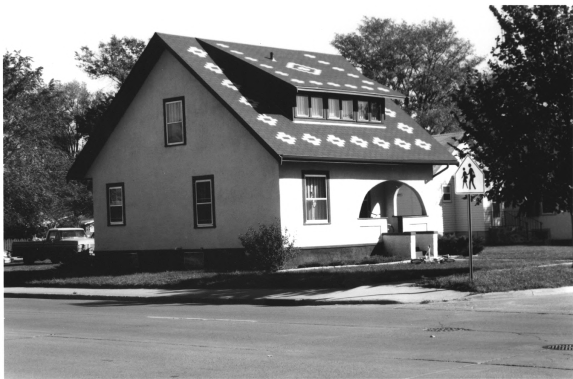
C. E. Chambers House, Davison County, So. Dak., No. 1
