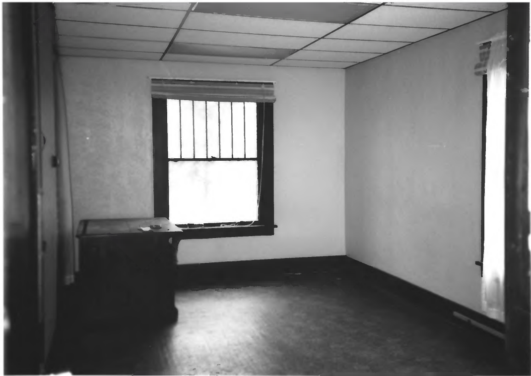
C. E. Chambers House, Davison County, So. Dak., No. 6
