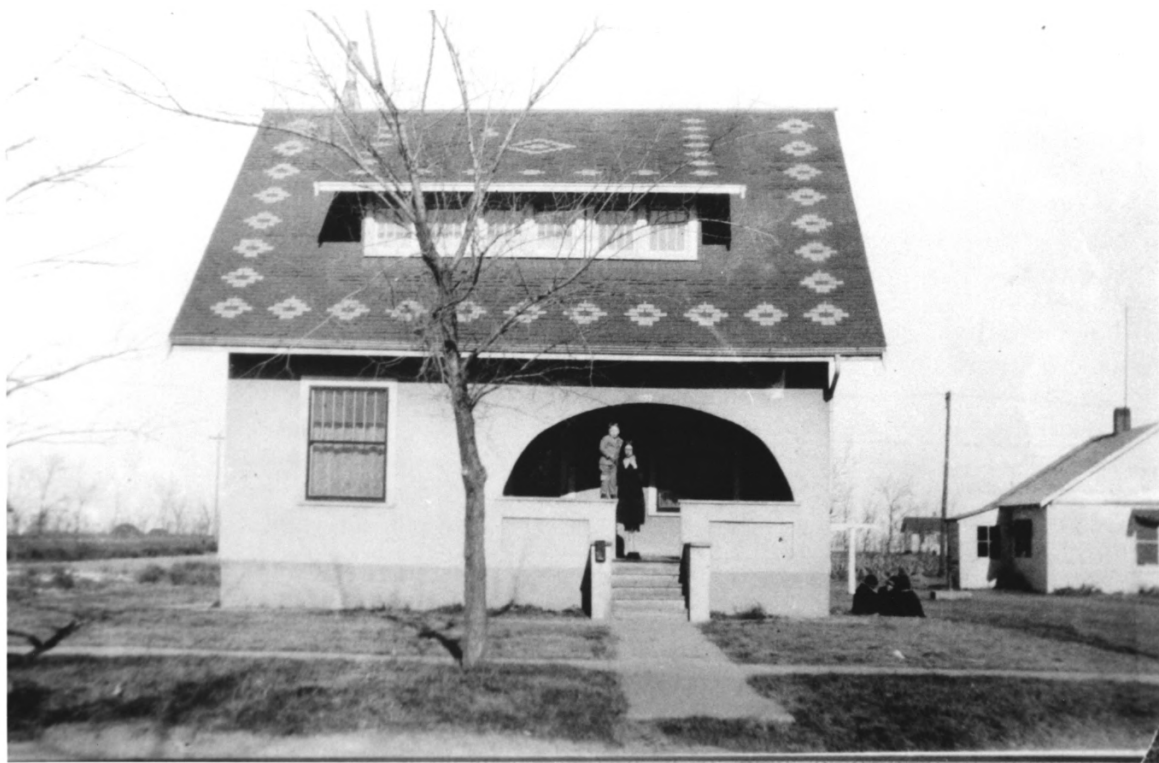
C. E. Chambers House, Davison County, So. Dak., No. 2
