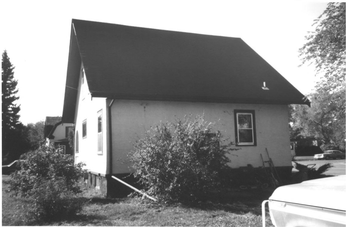
C. E. Chambers House, Davison County, So. Dak., No. 4
