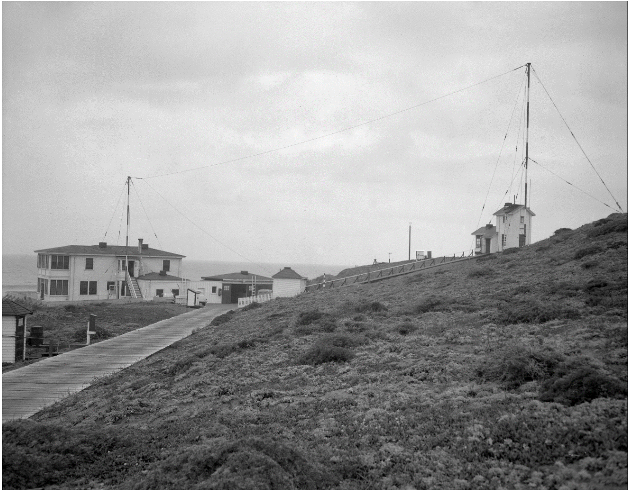
Figure 7. Photograph of the Point Reyes Naval Radio Compass Station, ca. 1943. The radio compass station is on the left, and the dormitory and ancillary buildings are on the right. (Point Reyes National Seashore Archives, HPRC 47710)
