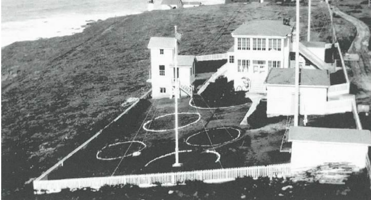
Figure 14. Photograph of the Point Montara Naval Radio Compass Station, ca. 1920s. The radio compass building is located on the left. (J.P. Ruschmeyer)
