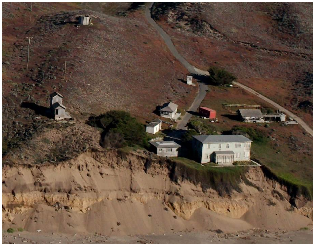
Figure 12. Aerial photograph of the Point Reyes Naval Radio Compass Station, September 2013. The shoreline has eroded such that the dormitory on the right is located at the cliff edge. (Kenneth and Gabrielle Adelman, California Coastal Records Project)
