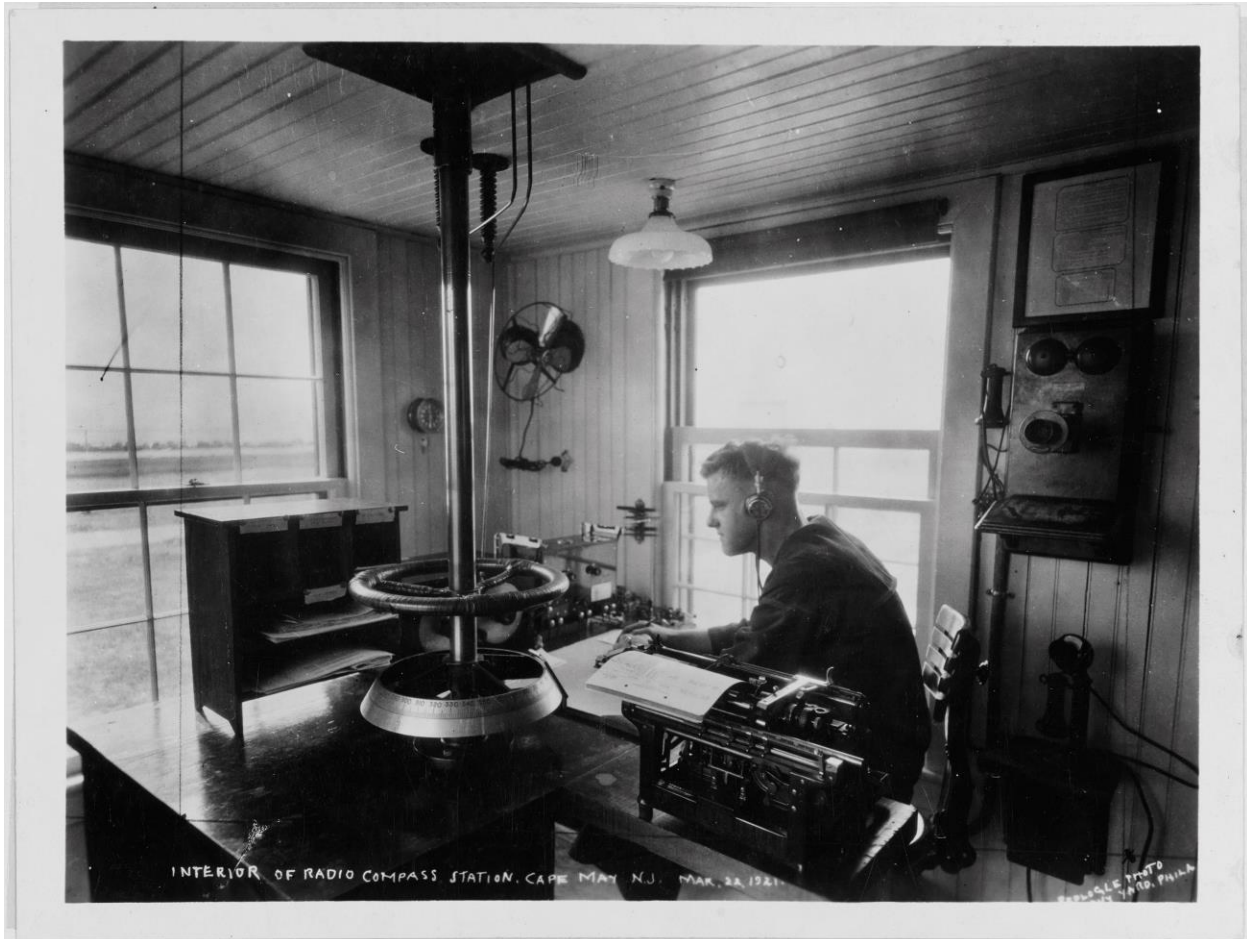
Figure 18. Interior photograph of the radio compass station at Cape May, New Jersey, 1921. The Point Reyes Naval Radio Compass Station would have had a similar setup. The radio compass is controlled by turning the metal ring on the left. (Naval History and Heritage Command, Photograph No. NH 122667)
