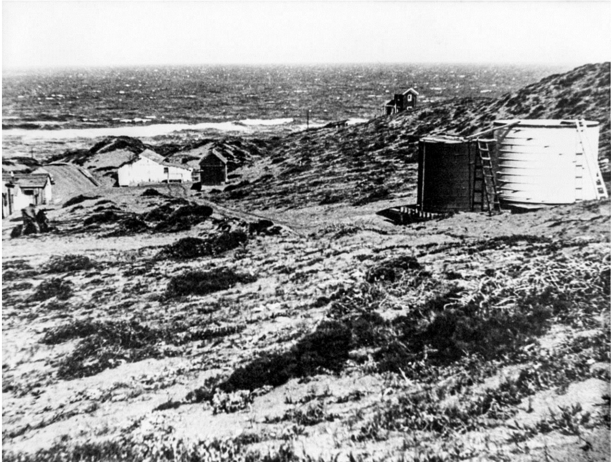
Figure 3. Photograph of the Point Reyes Naval Radio Compass Station, ca. 1920-1923. The radio compass station building is in the background on the right. (Point Reyes National Seashore Archives, HPRC 43050)
