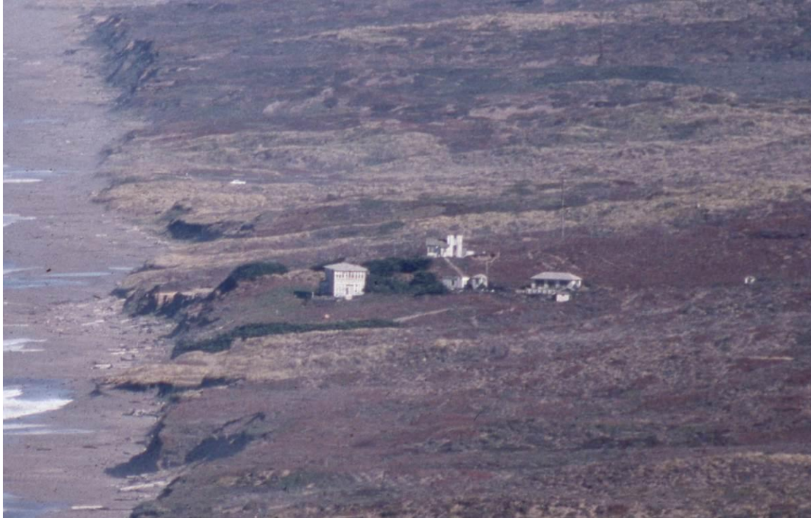
Figure 10. Aerial photograph of the Point Reyes Naval Radio Compass Station, September 1995 (Point Reyes National Seashore Archives, Don Gunn Collection, HPRC 8057.485)
