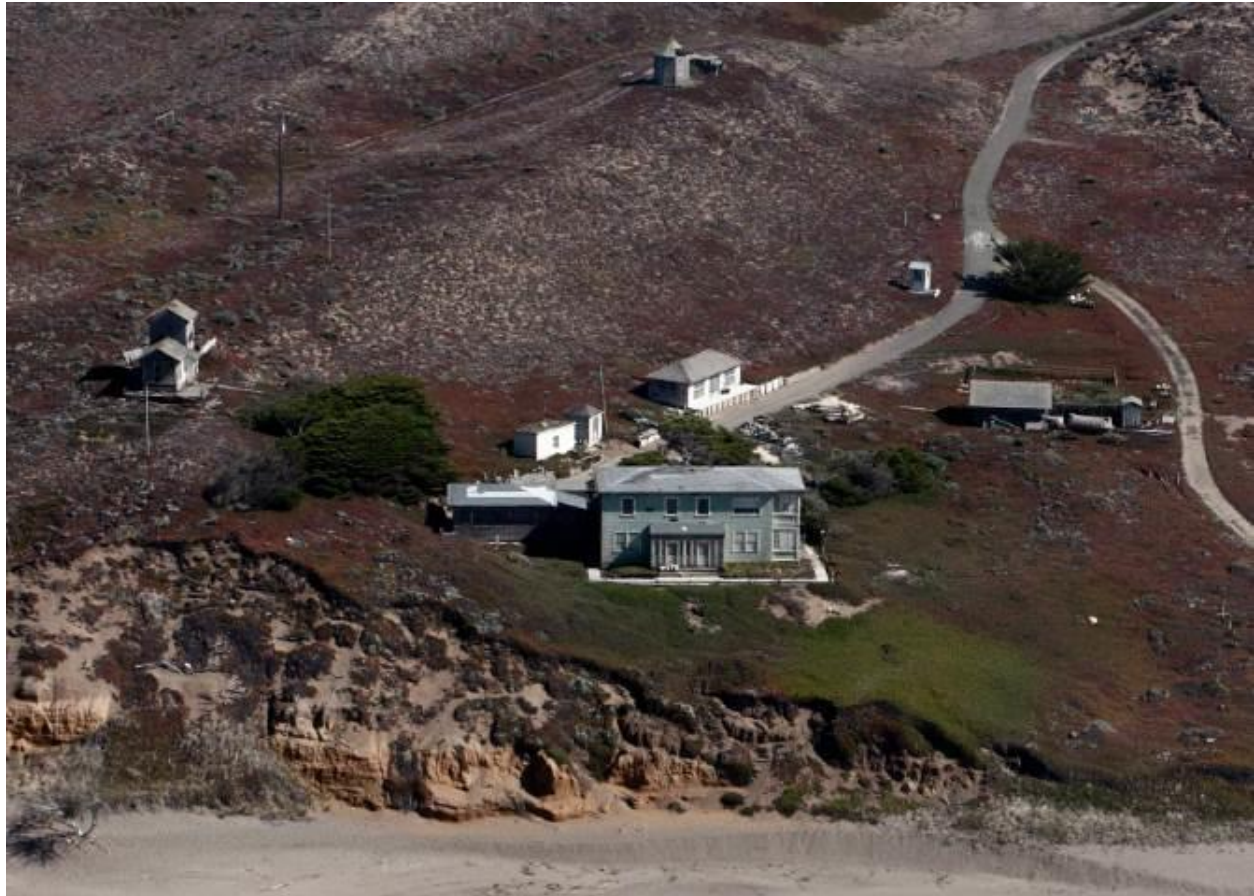
Figure 11. Aerial photograph of the Point Reyes Naval Radio Compass Station, October 2009. The photograph depicts the eroding shoreline. (Kenneth and Gabrielle Adelman, California Coastal Records Project)
