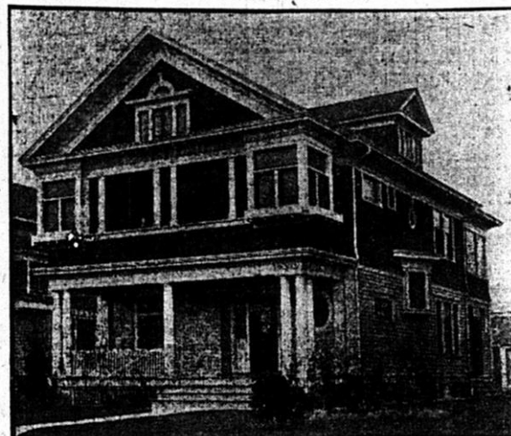
The characteristic feature of the recently remodeled residence of R. L. Vance, at 506 South Sheridan avenue, is to be found in the two large open-air sleeping porches. Both are on the second floor, one being in the front and the other in the rear of the house. Besides the sleeping porches there are eight large rooms and full cement basement. The house is heated by a hot air furnace. Potter & Merrill were the designing architects.
