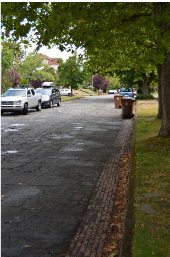
7 of 20 – Streetscape showing brick gutters, S Sheridan Ave. looking north.
