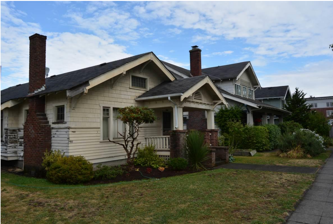
2 of 20 – Streetscape, S “M” St. looking north, west side of street.
