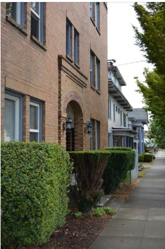
15 of 20 – Various apartments NE corner of S 6 th Ave & S Sheridan.
