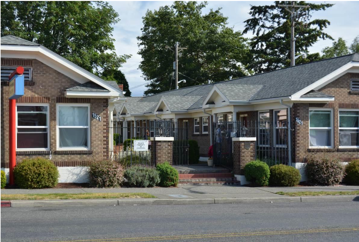
18 of 20 – 1521 S 6 th Ave., former Creso Court Apartments.
