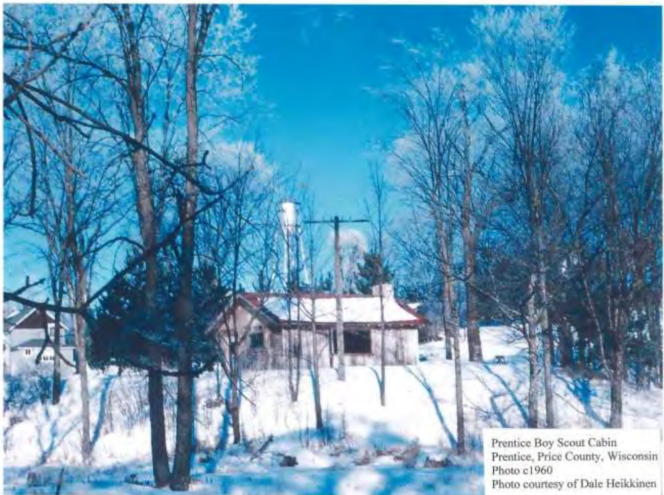
Figure 3: Historic Photograph, c1960
