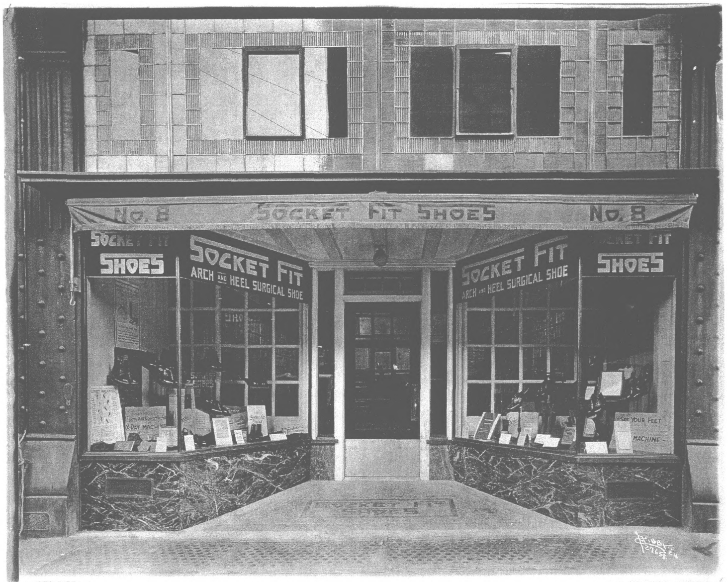
c. 1930s to 1940s. SOCKET FIT SHOES STOREFRONT, NORTH 8 POST STREET, PEYTON BUILDING. SOURCE: NORTHWEST MUSEUM OF ARTS AND CULTURE.
