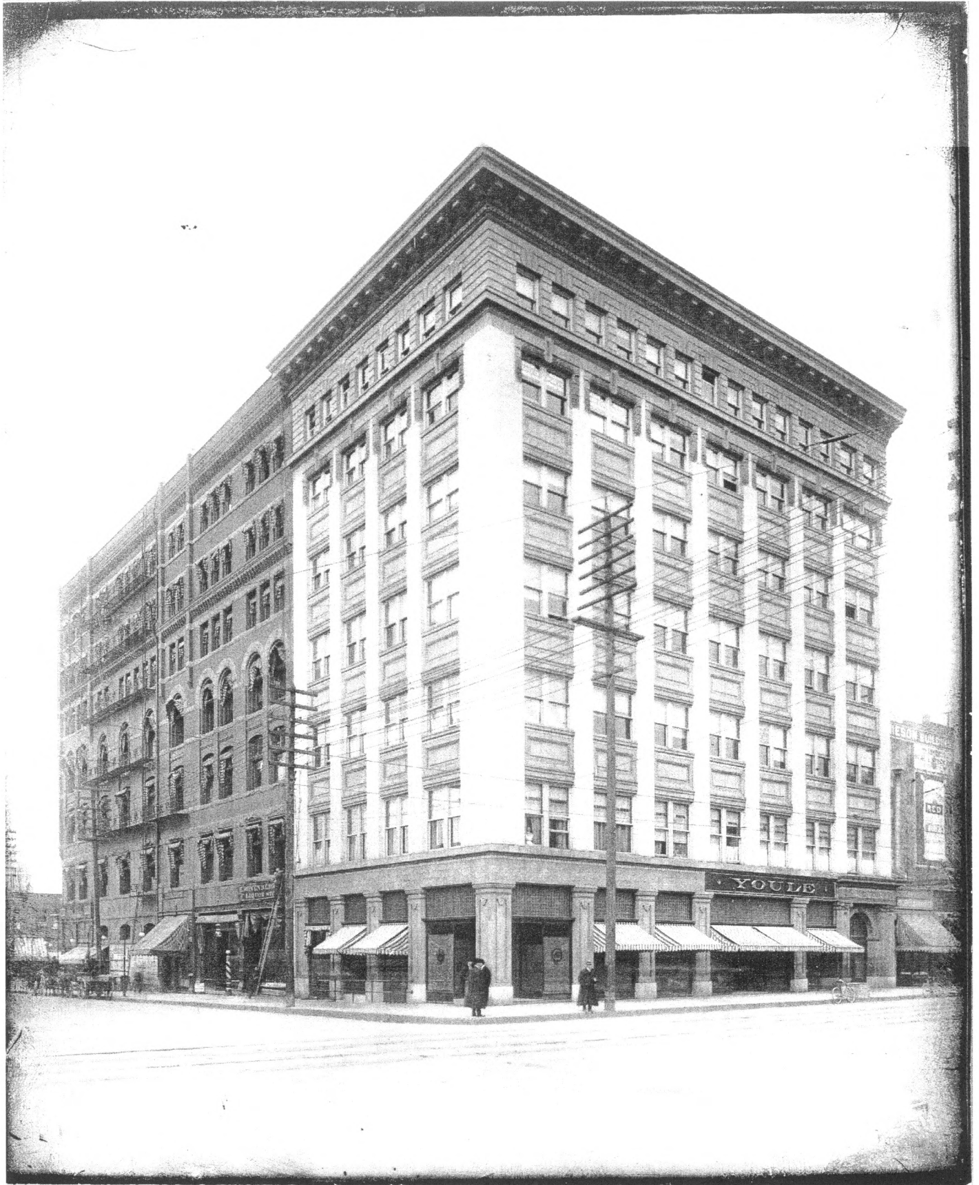
1909. PEYTON BUILDING (LEFT) AND PEYTON ANNEX (RIGHT). VIEW: LOOKING NORTHEAST. SOURCE: NORTHWEST MUSEUM OF ARTS AND CULTURE.
