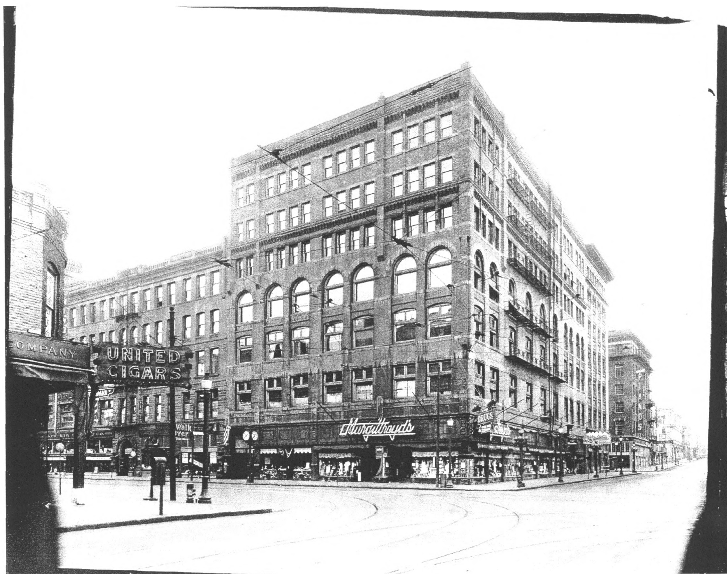
C. 1920. PEYTON BUILDING AND PEYTON ANNEX. VIEW: LOOKING SOUTHEAST. SOURCE: NORTHWEST MUSEUM OF ARTS AND CULTURE.
