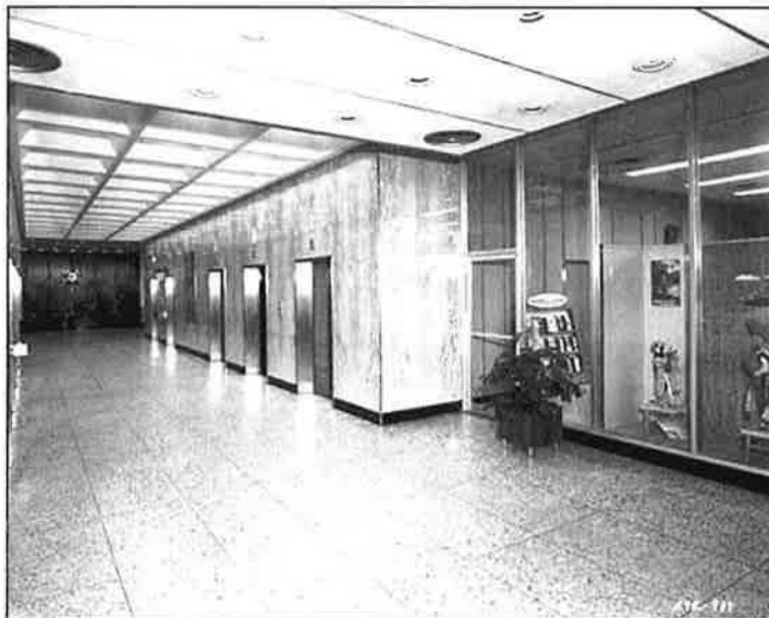
Figure 8: The first-floor elevator lobby of the Cargill Building.
