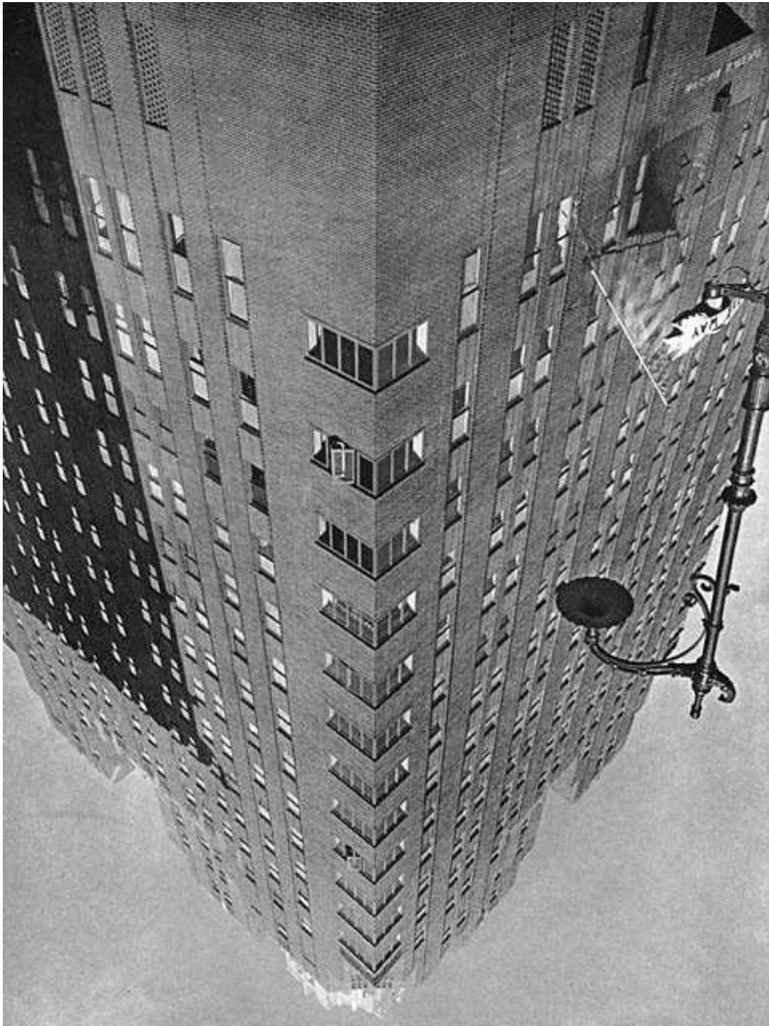
Photograph of corner windows on southwest corner of the Master Building. Source: "The Roerich Museum and Master Apartment Building, New York," Architectural Record , December, 1929.
