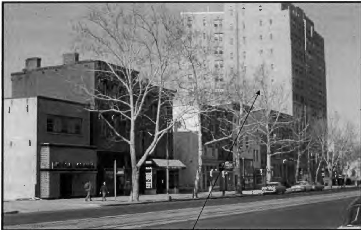
Keystone Apartments/H.B. Burns Memorial Building
