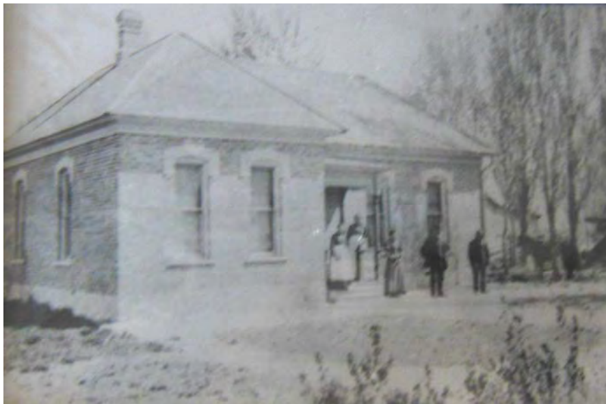
Figure 1 South and west elevations of Amundsen House, photographed circa 1892. (courtesy of Tamra Lee, best available copy)
