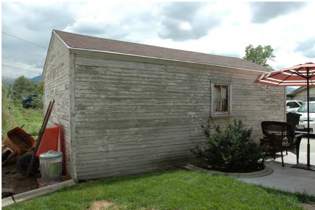
Photograph 6 of 9 West elevation of garage. Camera facing southeast.
