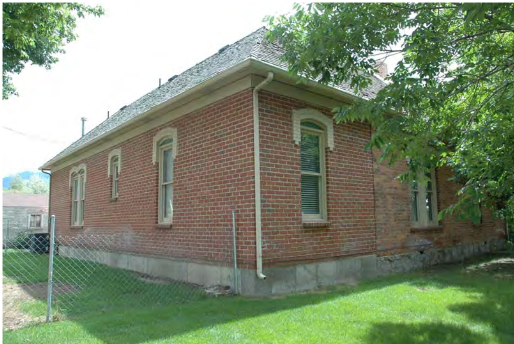
Photograph 4 of 9 North and west elevations of Amundsen House. Camera facing southeast.
