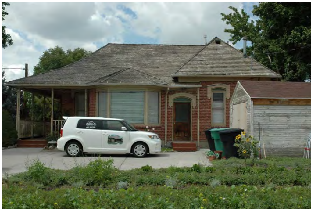
Photograph 5 of 9 East elevations of Amundsen House and garage. Camera facing west.
