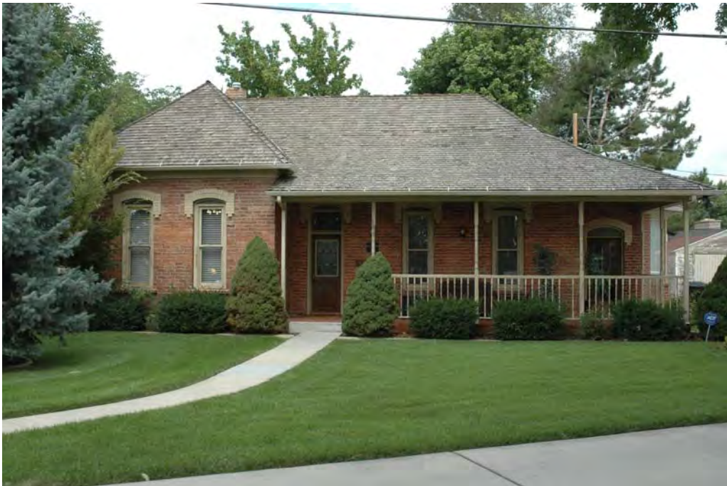
Photograph 1 of 9 South elevation of Amundsen House. Camera facing north.
