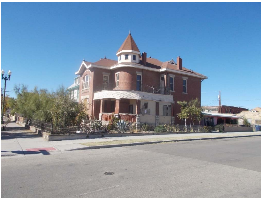
Photo 12 Property #118 1129 Magoffin Avenue, SE oblique looking NW, Apr 2015
