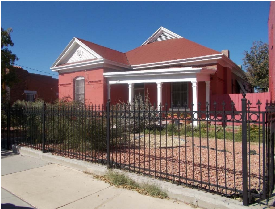
Photo 13 Property #24 1103 East San Antonio, south elevation looking west, May 2014
