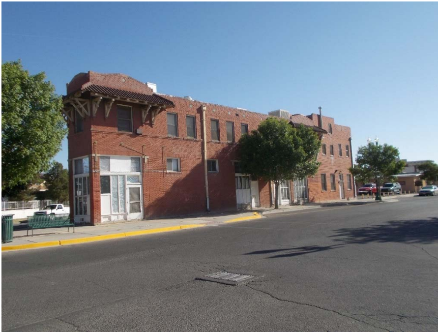
Photo 171 Property #15 1003 E San Antonio, Triangle Building, south elevation looking north, May 2014
