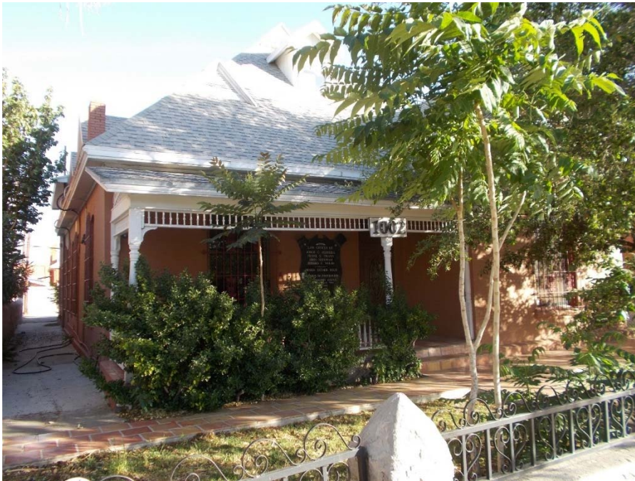
Photo 9 Property #105 1002 Magoffin Avenue, north elevation looking south, May 2014
