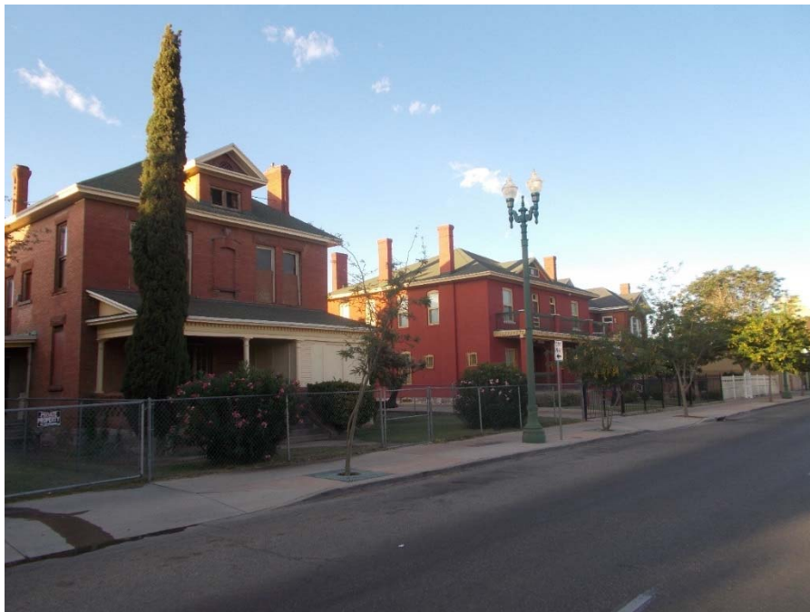
Photo 10 Properties #104, 103, 102 South side 900 block Magoffin Avenue, looking SW, Jun 2014
