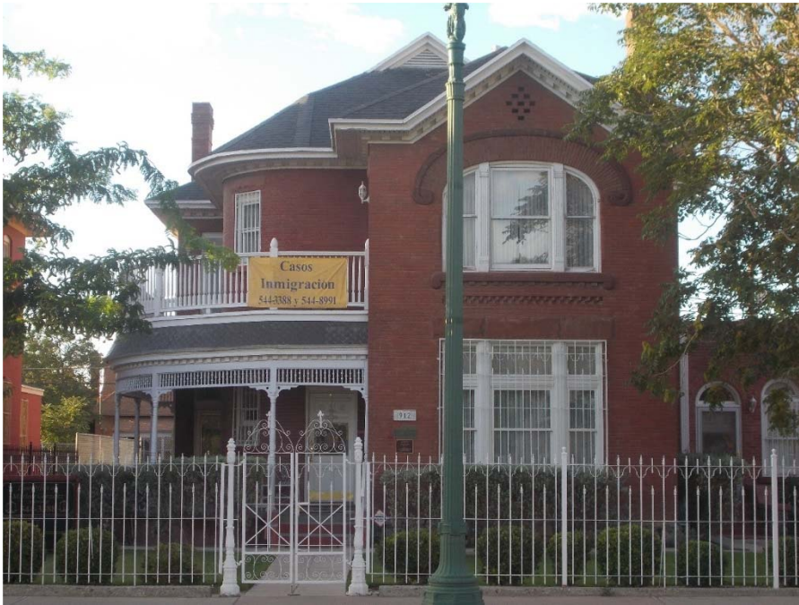
Photo 3 Property #102 912 Magoffin Avenue, north elevation looking south, Jun 2014
