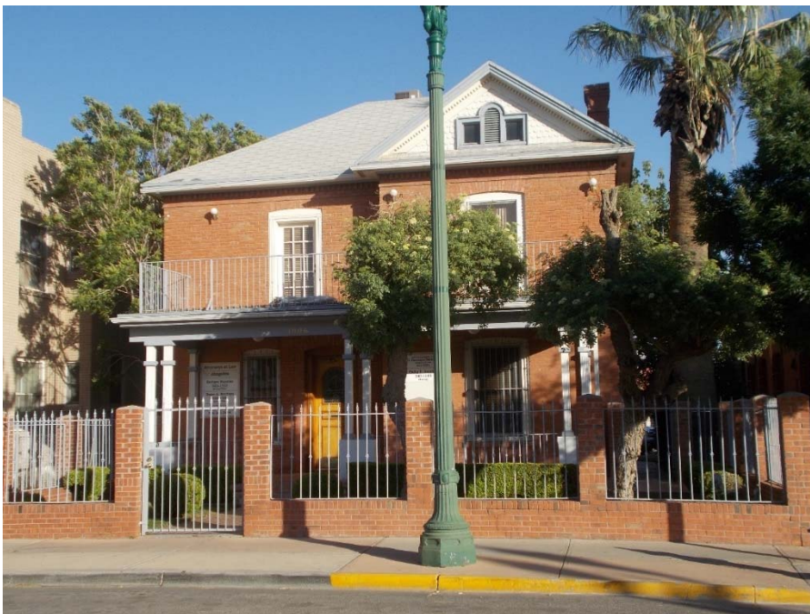
Photo 14 Property #106 1006 Magoffin Avenue, north elevation looking south, May 2014
