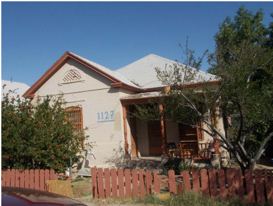
Photo 146 Property #171 1127 Myrtle, south elevation looking NW, May 2014
