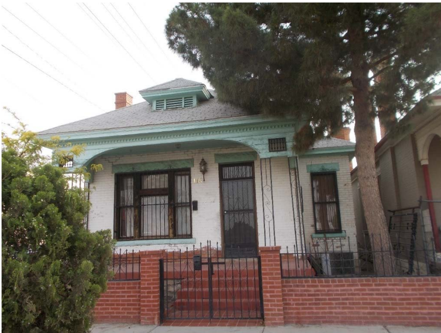
Photo 15 Property #96 115 Hills, east elevation looking west, May 2014
