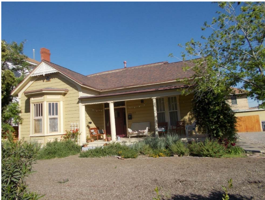
Photo 2 Property #189 817 Olive Avenue (Beall House), south elevation looking NW, May 2014
