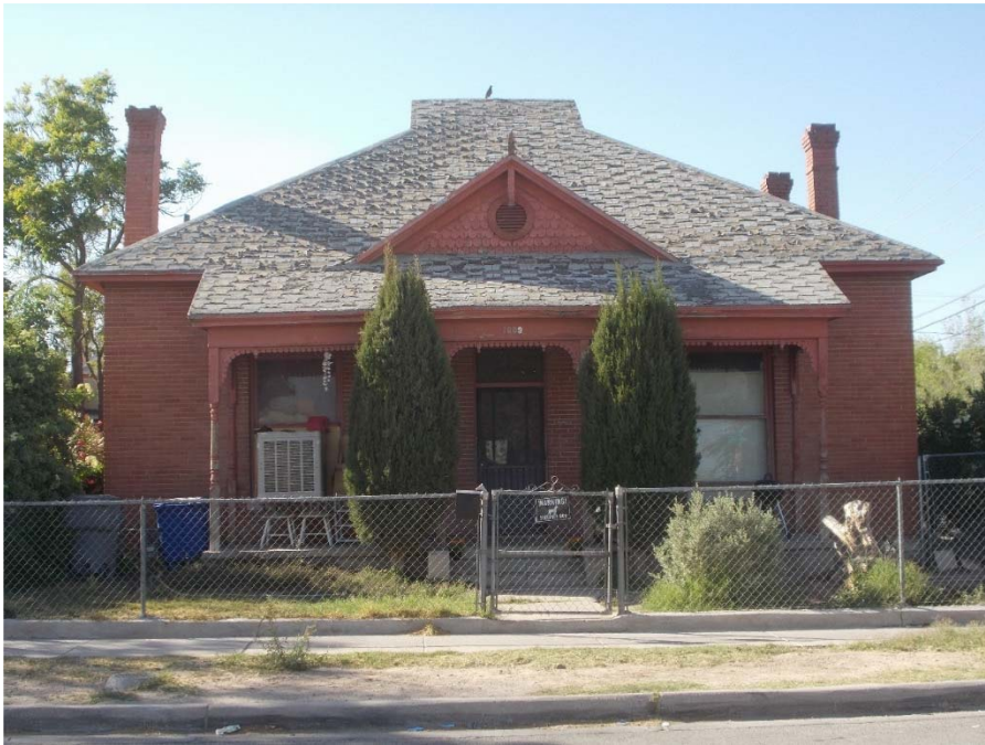
Photo 17 Property #204 1009 Olive, south elevation looking NW, May 2014
