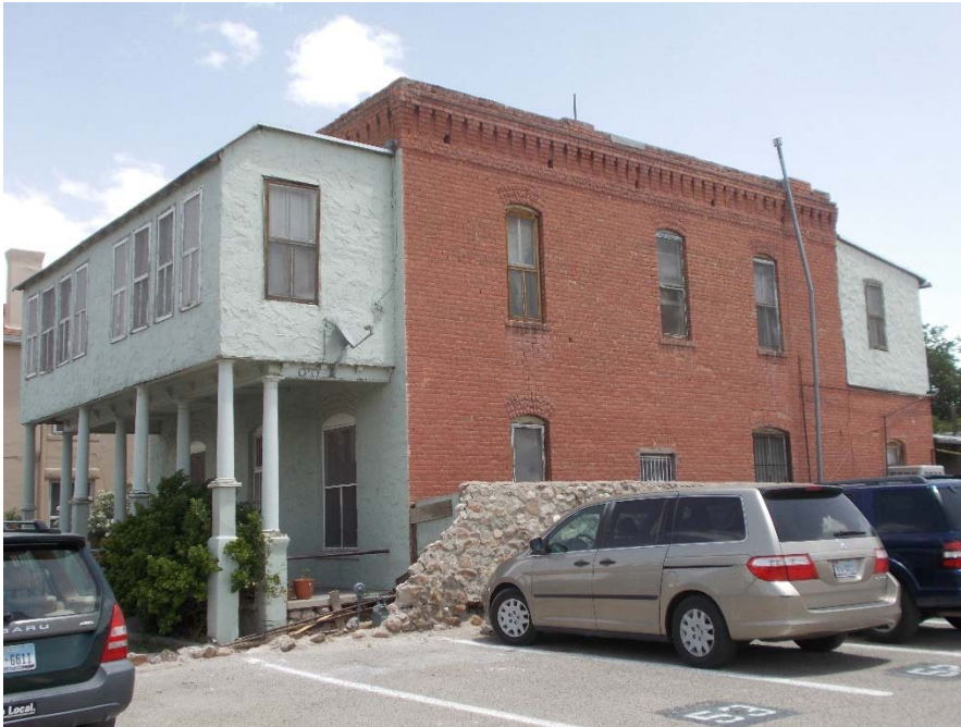
Photo 19 Property #99 812 Magoffin, west elevation looking east, May 2014
