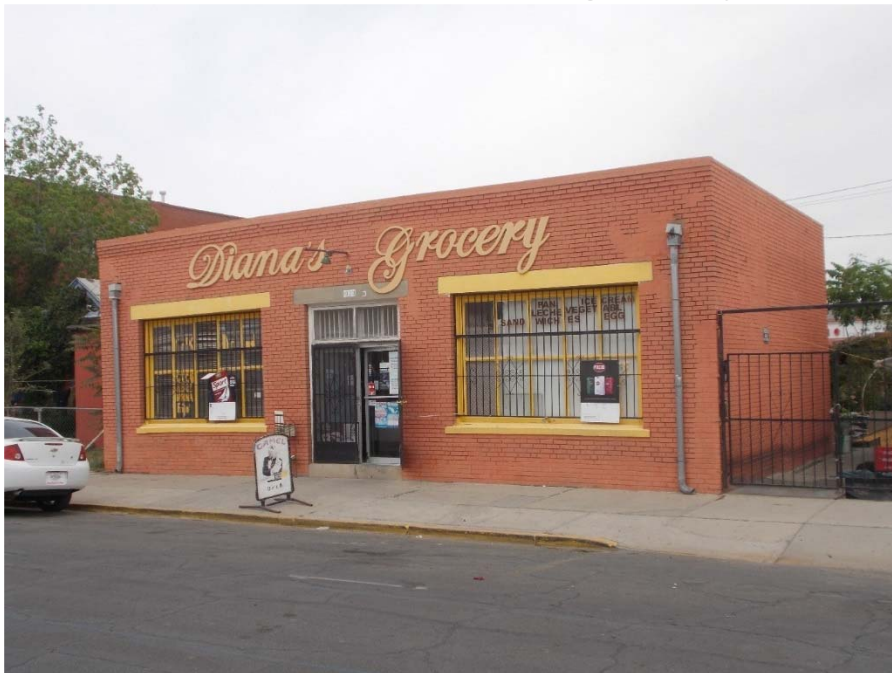
Photo 26 Property #153 1023 Myrtle, south elevation looking west, May 2014
