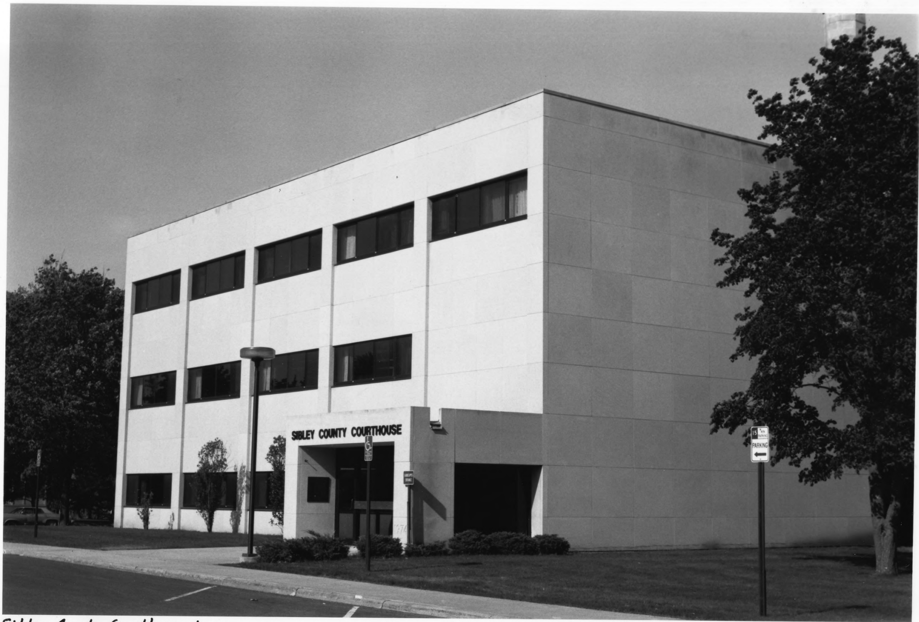
Sibley County Courthouse Annex Grayford, MN 09255-6
