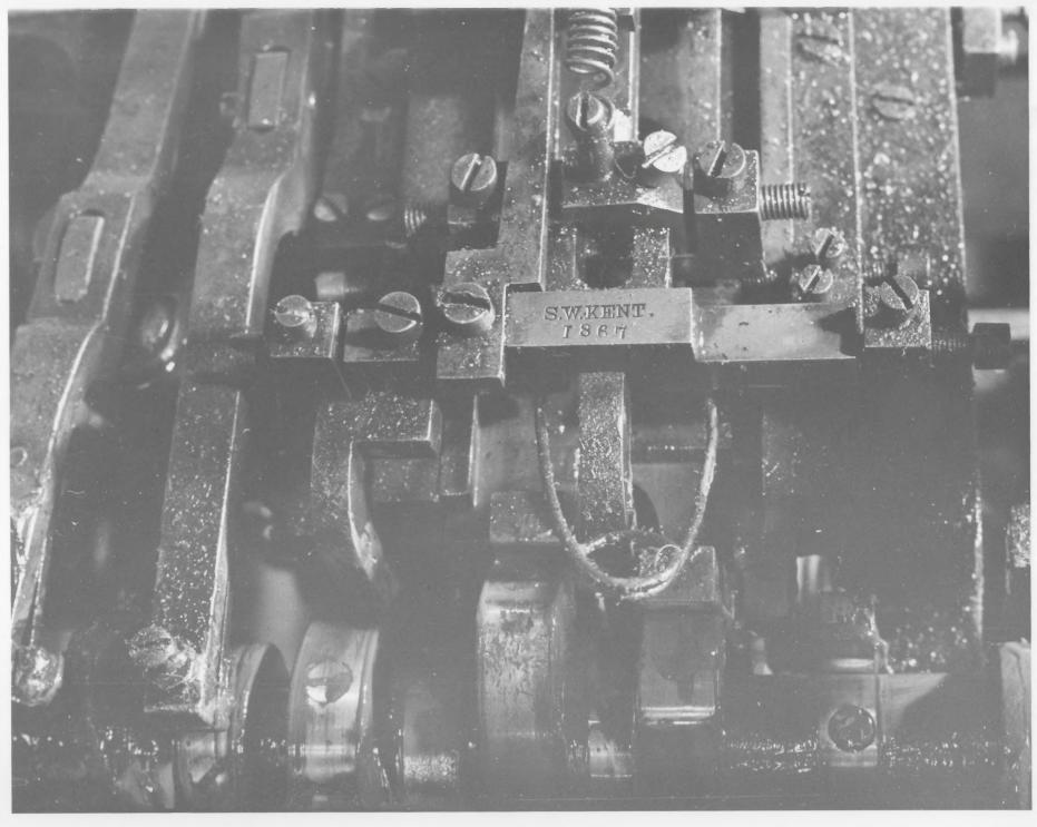
close up of 1867 tooth making and setting machine fax wool hand cards,
