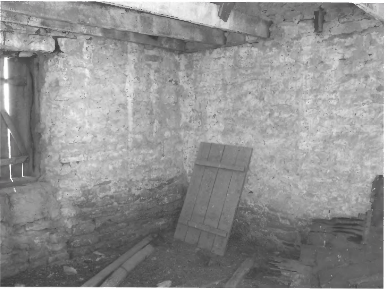
Lockkeeper's House Davis County, IA Photo #0007
