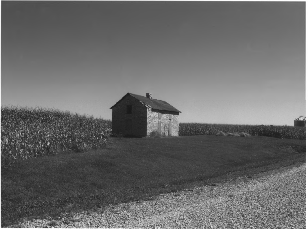
Lockkeeper's House Davis County, IA Photo #0001
