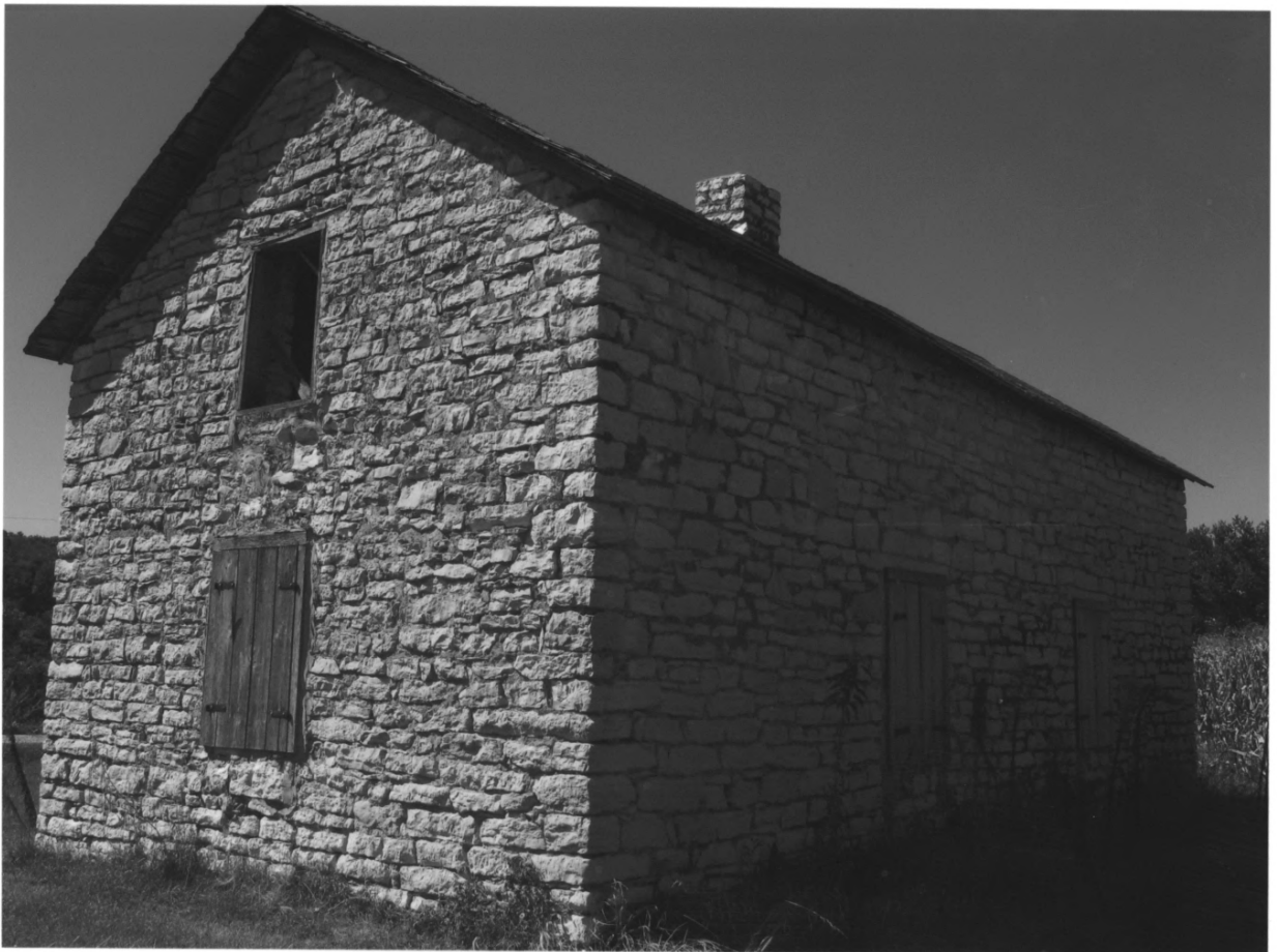
Lockkeeper's House Davis County, IA Photo #0004
