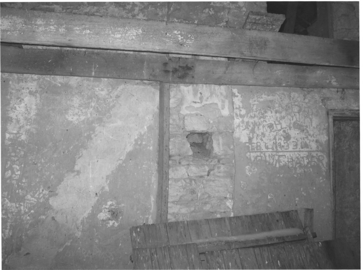
Lockkeeper's House Davis County, IA Photo #0011
