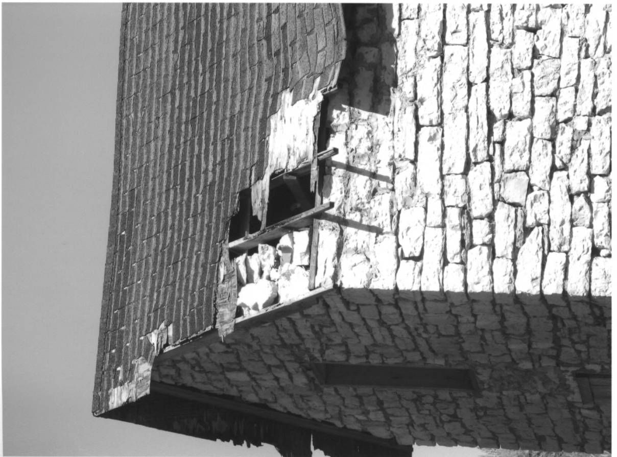
Lockkeeper's House Davis County, IA Photo #0006
