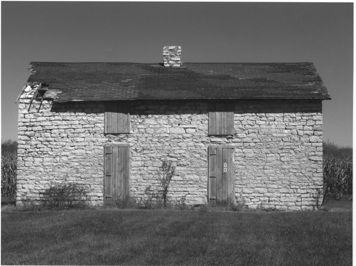
Lockkeeper's House Davis County, IA Photo #002
