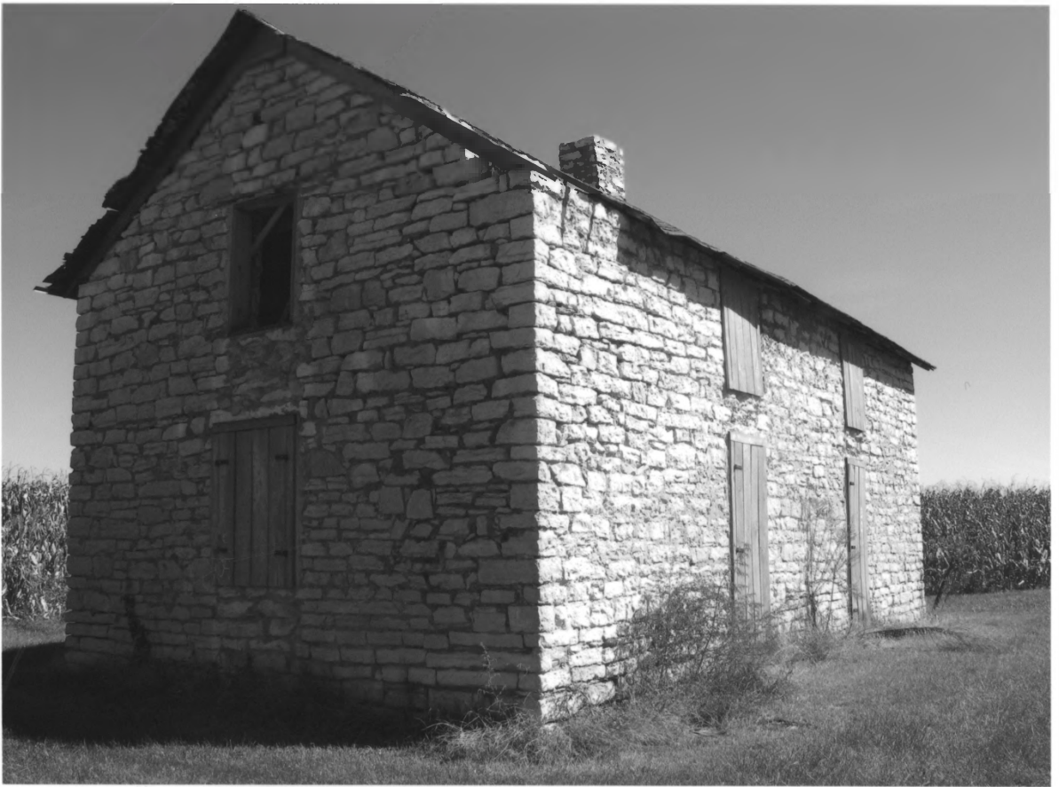
Lockkeeper's House Davis County, IA #0005
