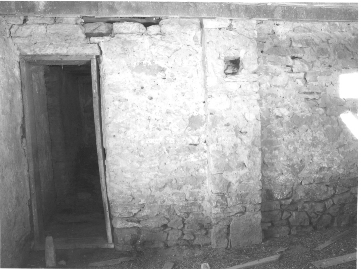
Lockkeeper's House Davis County, IA Photo #0008
