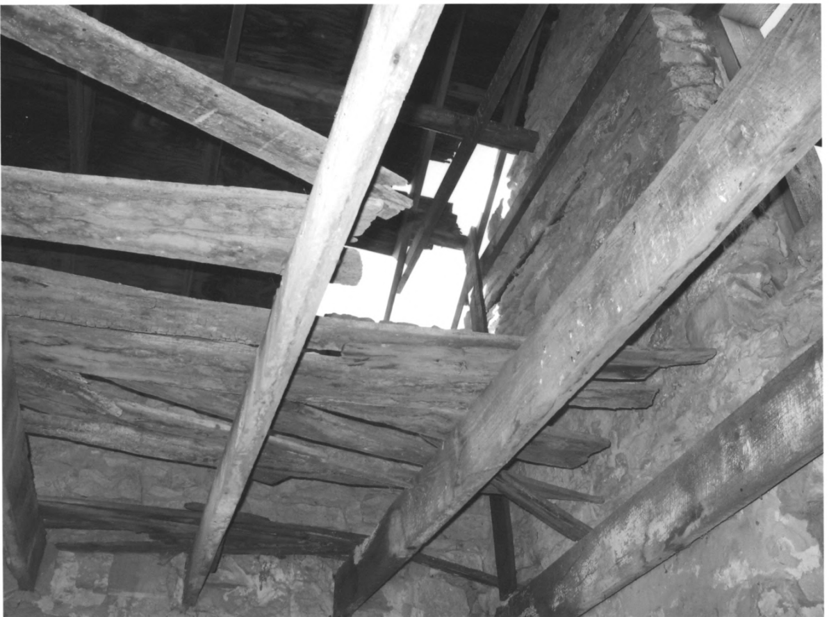
Lockkeeper's House Davis County, IA Photo #0012
