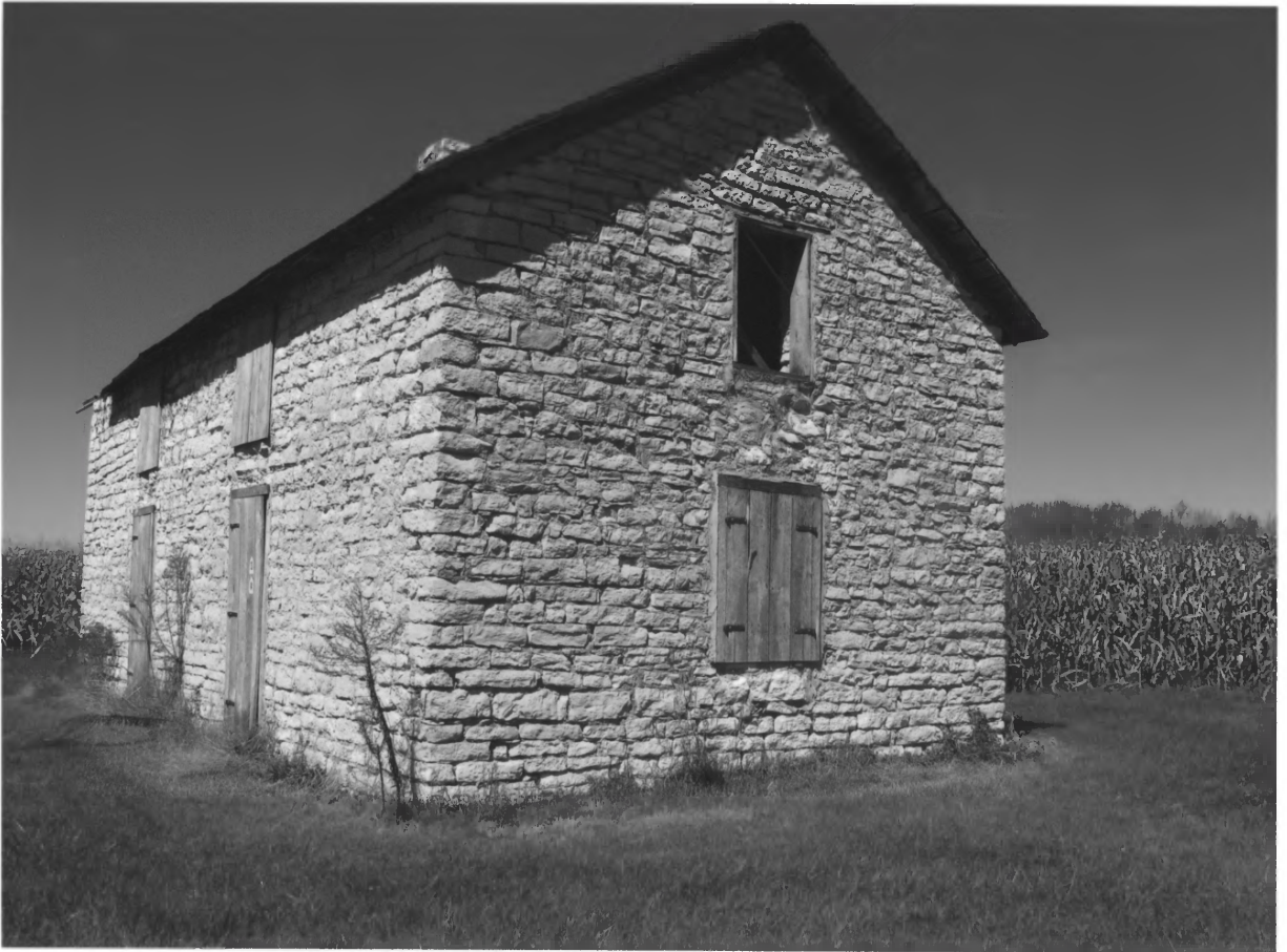
Lockkeeper's House Davis County, IA Photo #0003
