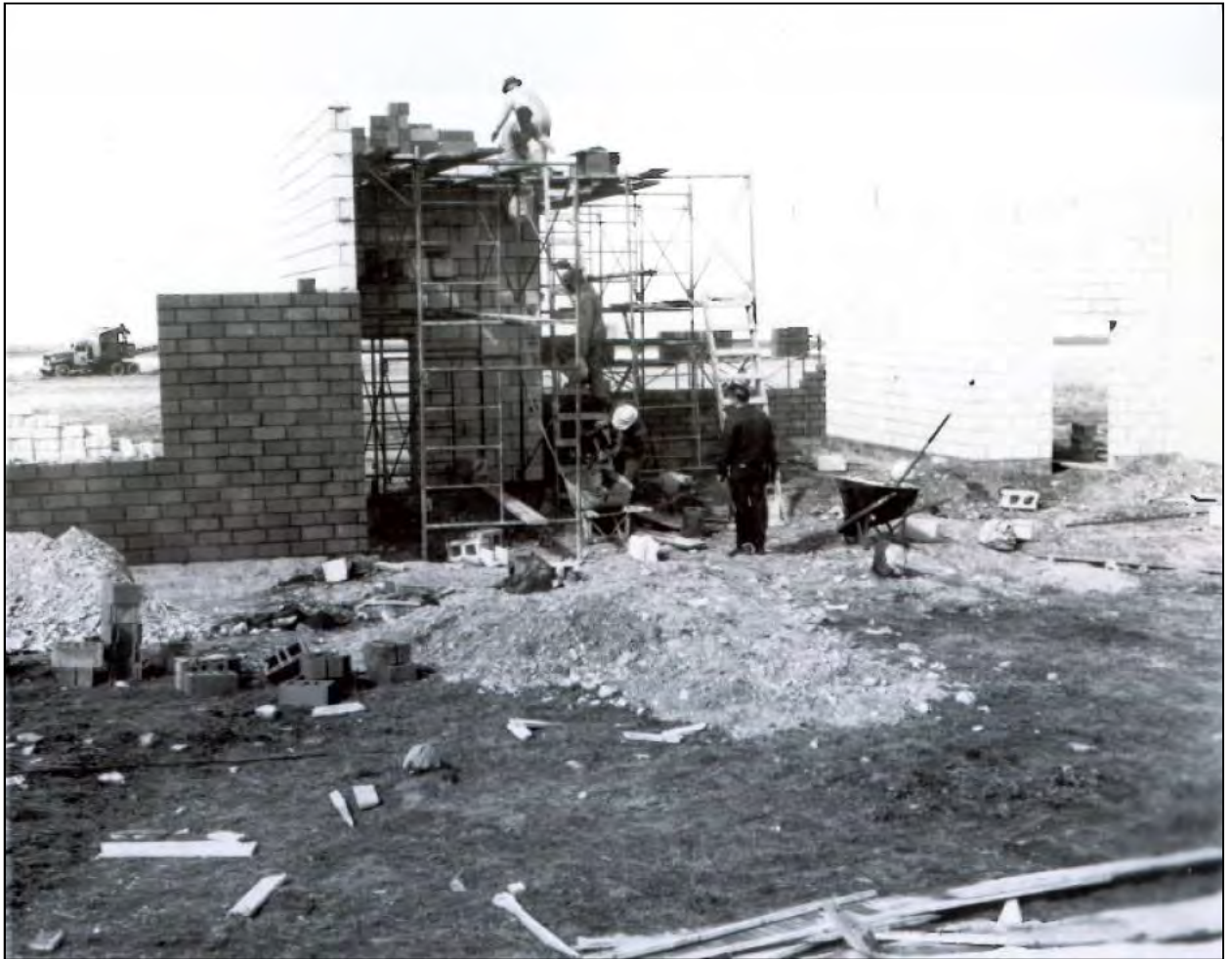
The Montana Aeronautics Commission Operations Building under construction. Spring 1958.
