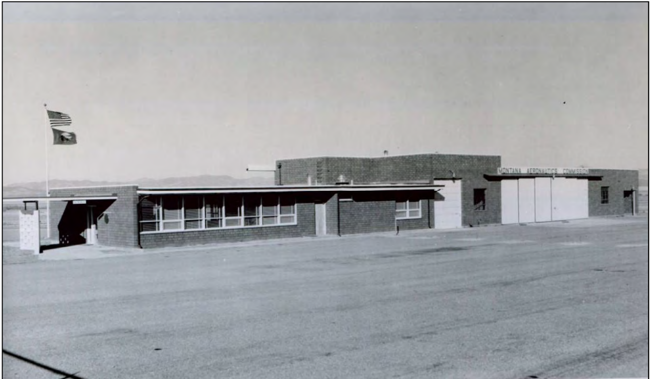
The Montana Aeronautics Commission Operations Building at completion, July 1958. South façade. View to the northeast.
