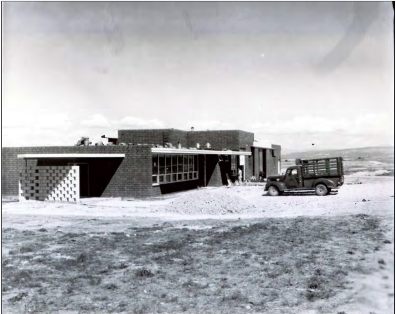
The Montana Aeronautics Commission Operations Building nearing completion. View to the east, 1958.
