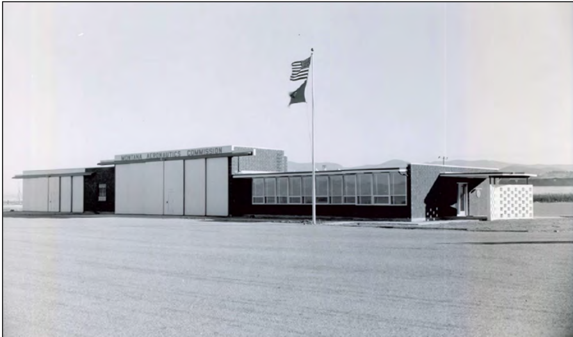
The Montana Aeronautics Commission Operations Building at completion, July 1958. North façade. View to the southeast.
