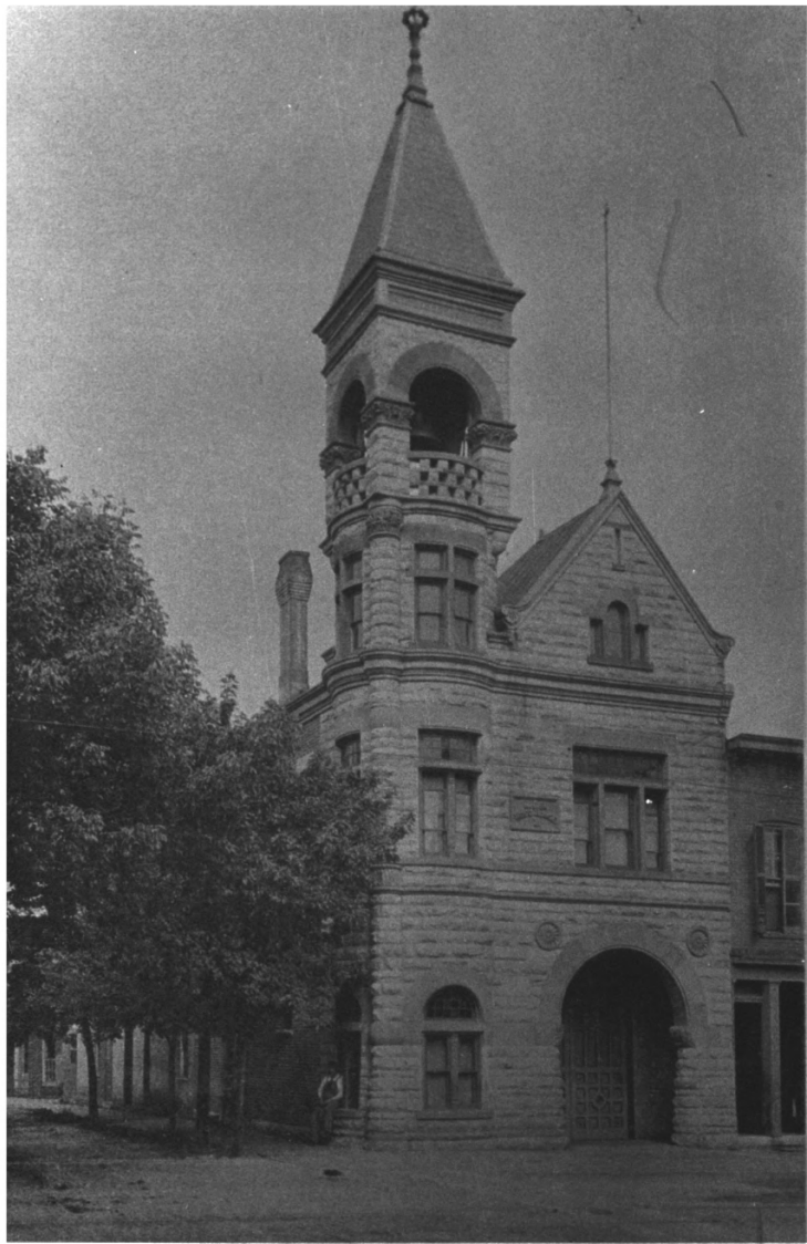
HOSE HOUSE NO. 1.
