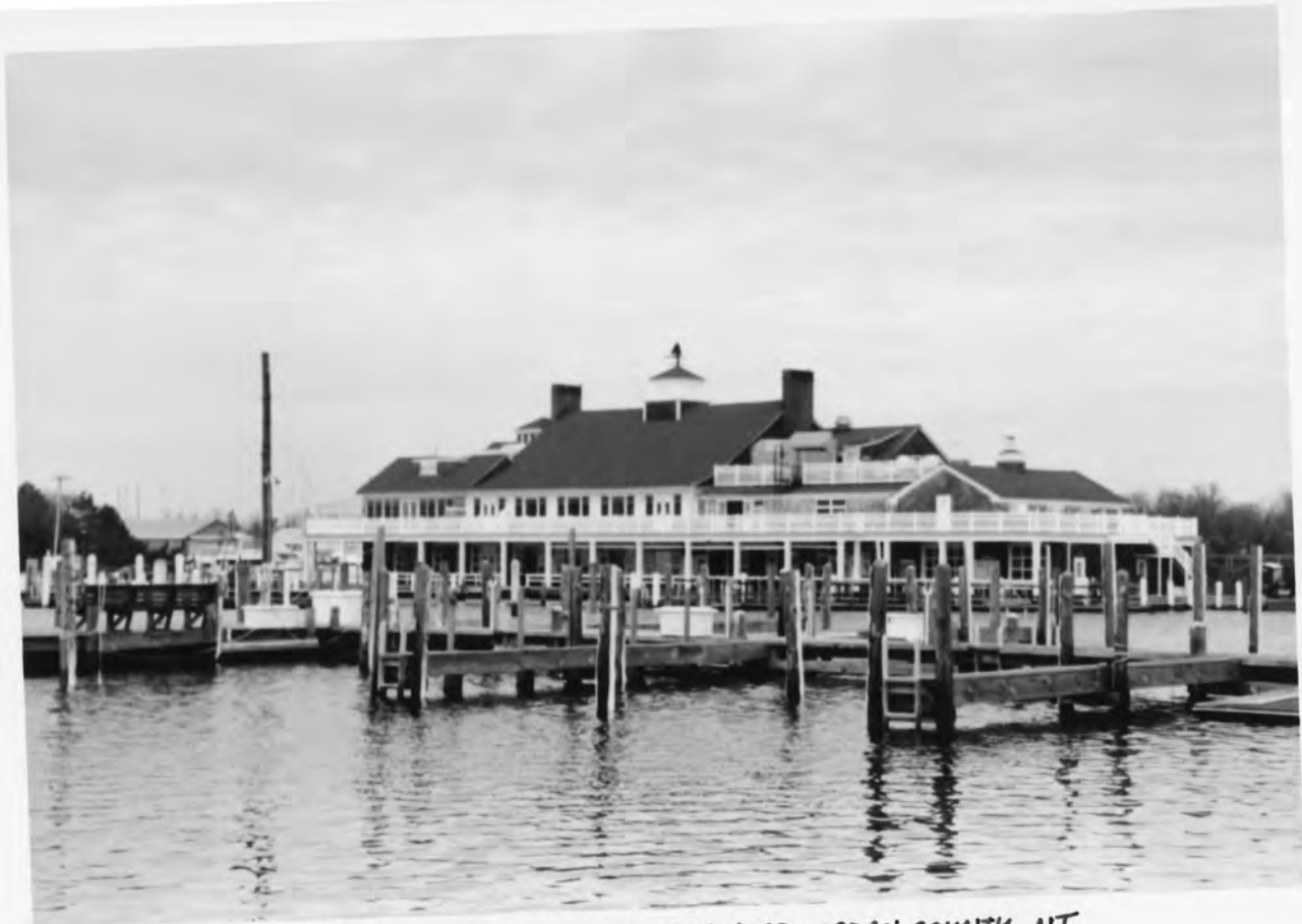
SLIDE 38 OF 75 . BAY HEAD HISTORIC DISTRICT. BAY HEAD, OCEAN COUNTY, NJ
