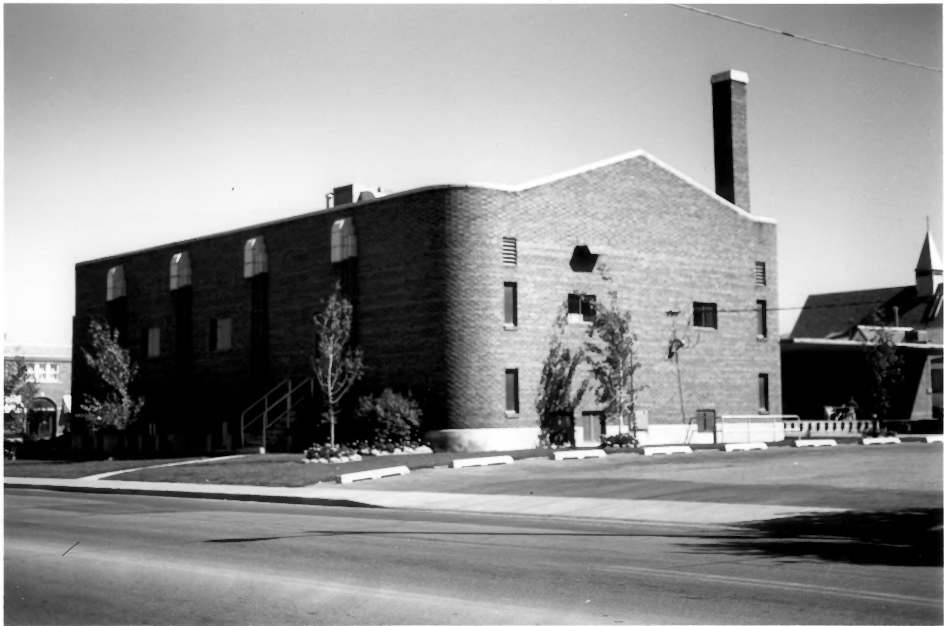
MIDVALE CITY HALL MIDVALE, UTAH (PHOTO #2)
