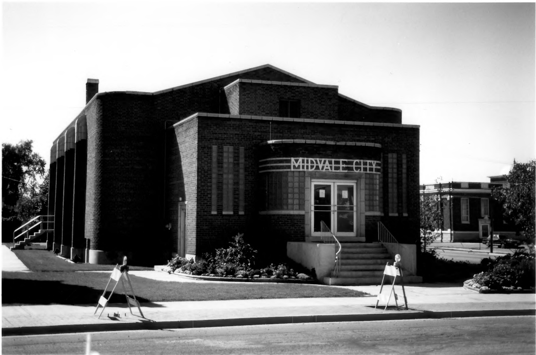
MIDVALE CITY HALL MIDVALE, UTAH (PHOTO #1)
