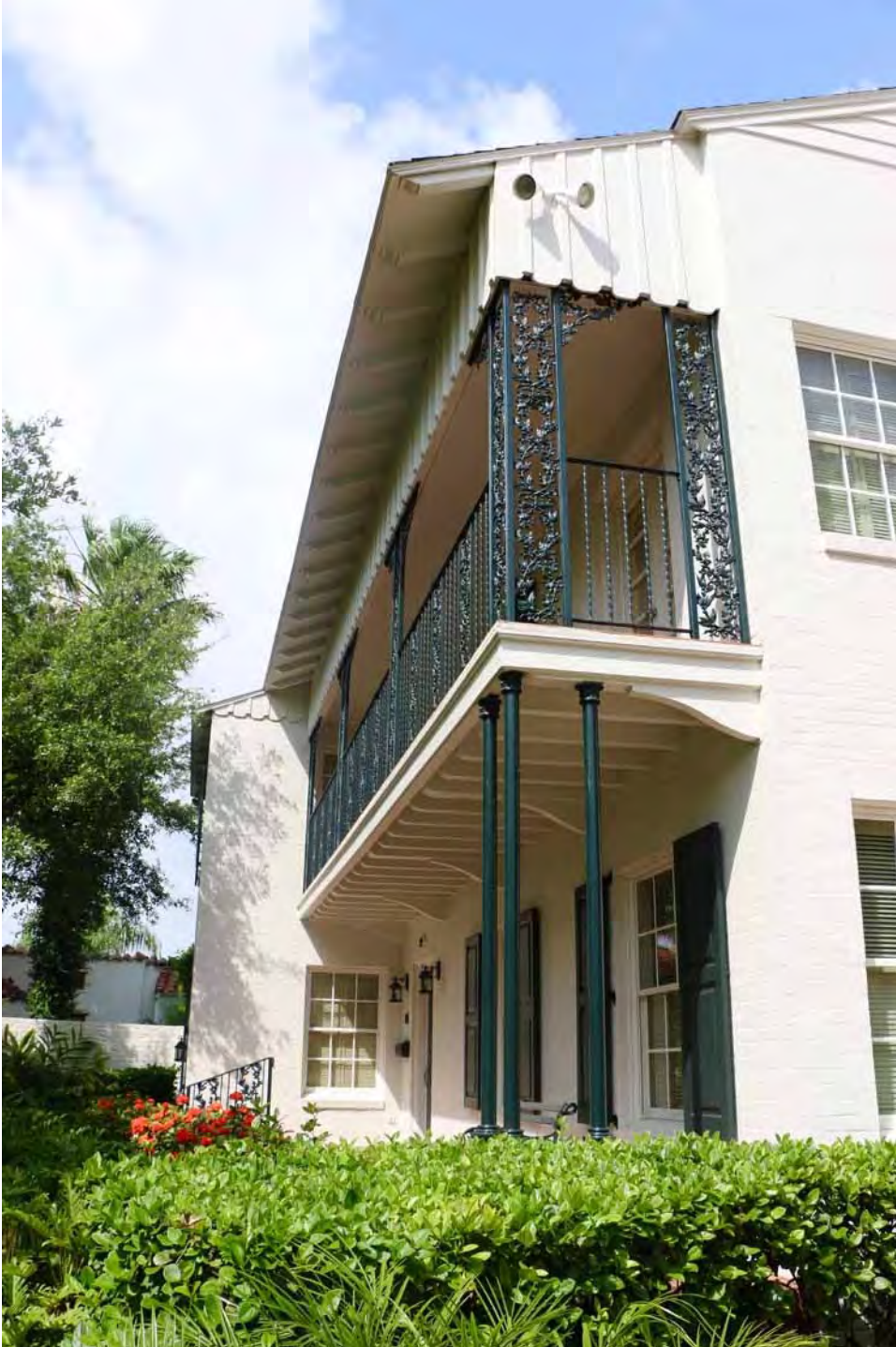
Photo 4: Detail of southeast (primary) elevation, looking approximately west.
