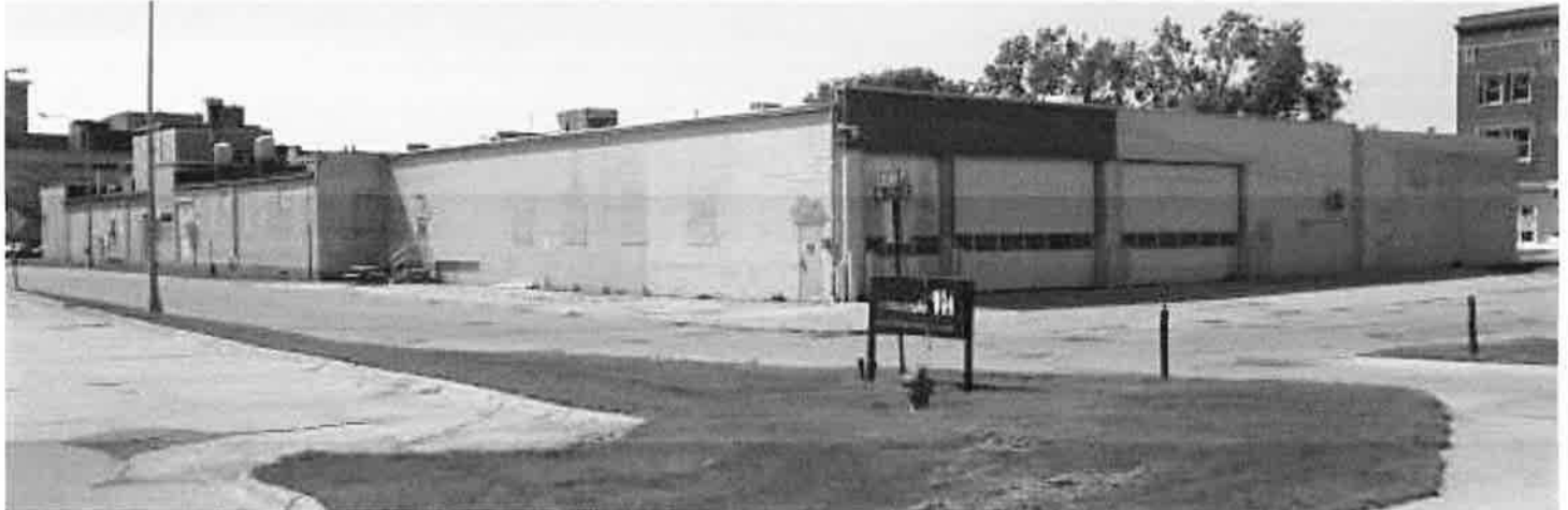
Figure 3 The overhead garage doors are the most notable feature of the northwest of the bakery complex. Tallgrass Historians L.C., 2015
