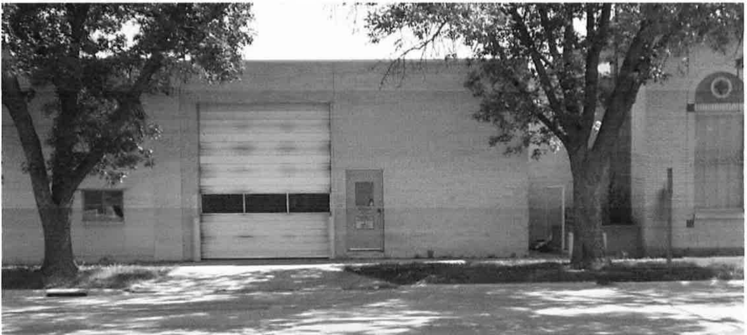
Figure 5 This is the Commercial Street exposure of the 1977 construction project that joined the small older corner brick building (at far left) to the midsection of the bakery building (far right). The inset notch that holds the water meter and piping is seen behind the tree on the right. Tallgrass Historians L.C., 2015
