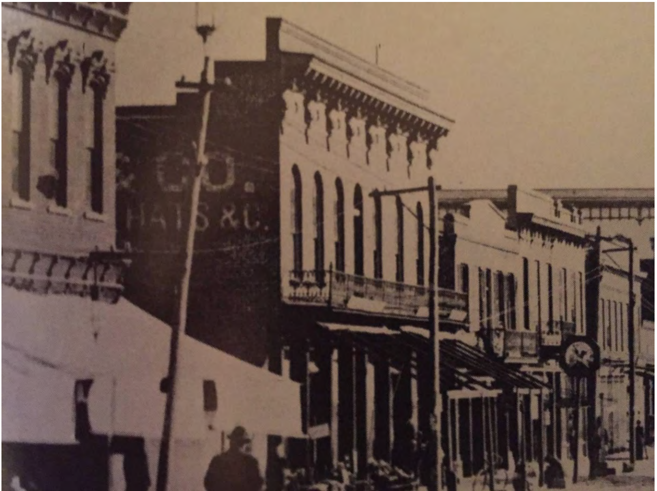
Figure 1. Columbia Commercial Historic District J. C. Penney/Maxwell Furniture Building, 1634 Main Street Columbia, Richland, South Carolina
