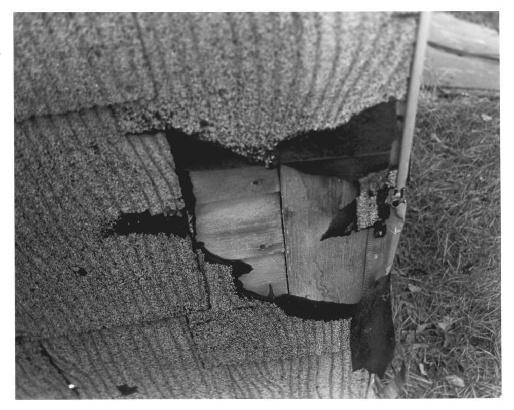
Photograph # 5 Bissell Tavern Windsor, Ct. Oct. 1984 Photo - Gail Nettles/Neg. on file Connecticut Historical Comm. North east corner showing original clapboards under asbestos siding
