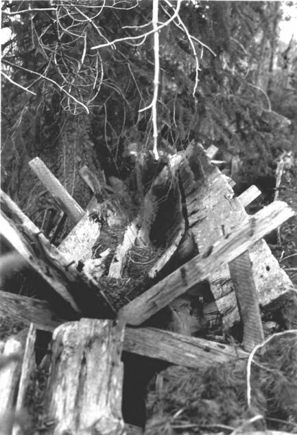
7. Flume remains showing construction detail, trough looking upstream. Located between Camps No.2 and No.3.
