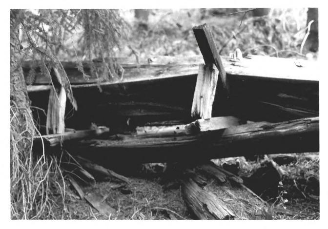
8. Flume remains showing construction detail of trough Located between Camps No.2 and No.3.
