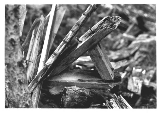
5. Flume remains showing bracing detail. Note cut spikes.
