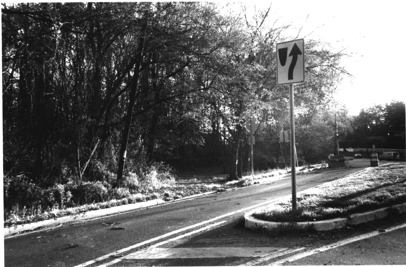
KING'S HIGHWAY (UPPER ROAD, LINCOLN HIGHWAY) NJ MERCER COUNTY 167 of 200
