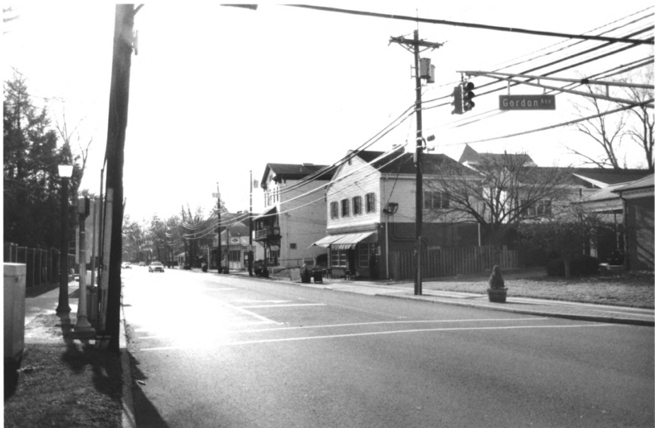
KING'S HIGHWAY (UPPER ROAD, LINCOLN HIGHWAY) NJ MERCER COUNTY 18304200
