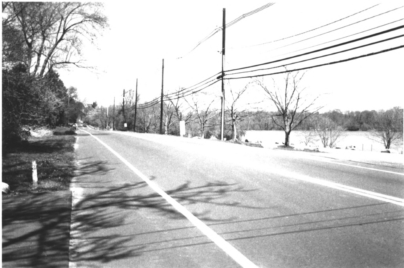
KING'S HIGHWAY (UPPER ROAD, LINCOLN HIGHWAY), NJ MERCER COUNTY 43 of 200
