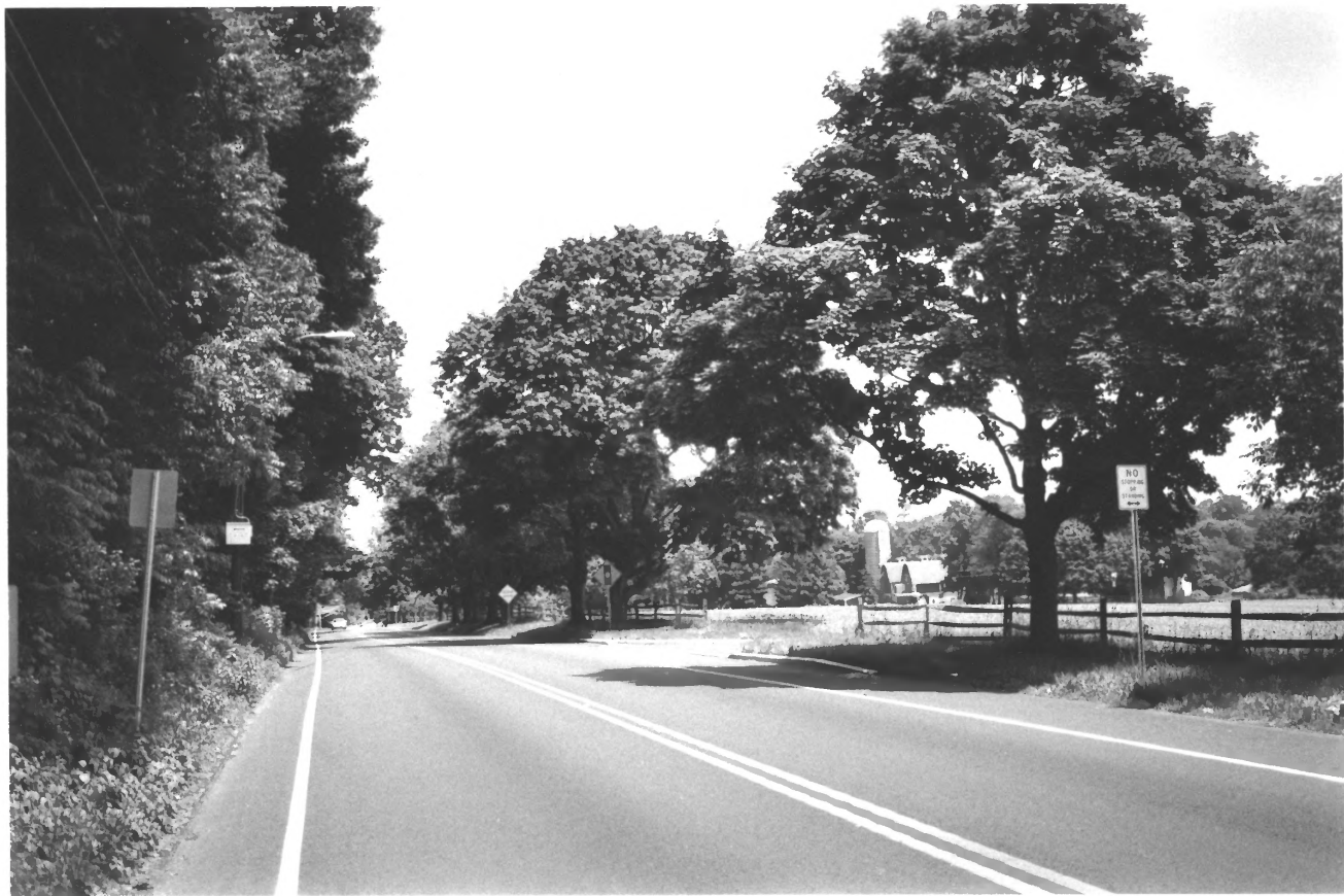
KING'S HIGHWAY (UPPER ROAD, LINCOLN HIGHWAY), NJ MERCER COUNTY 170 of 200
