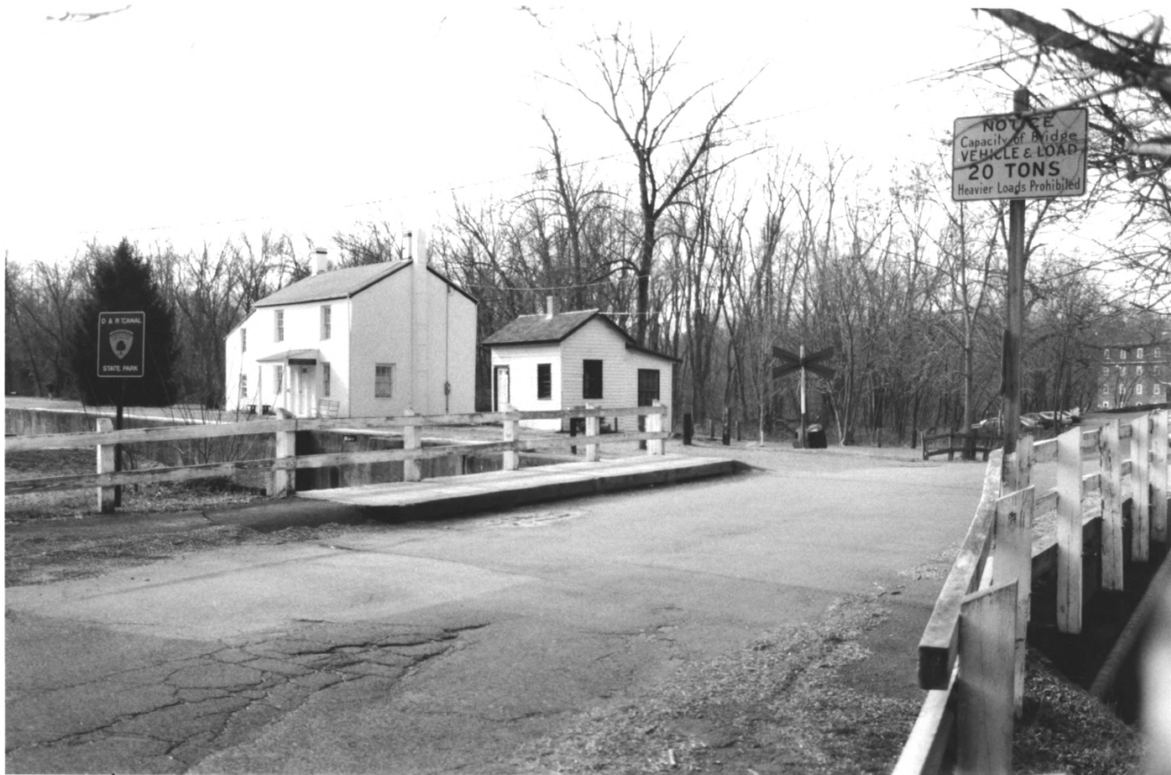
KING'S HIGHWAY (UPPER ROAD, LINCOLN HIGHWAY) NJ MERCER COUNTY 25 of 200
