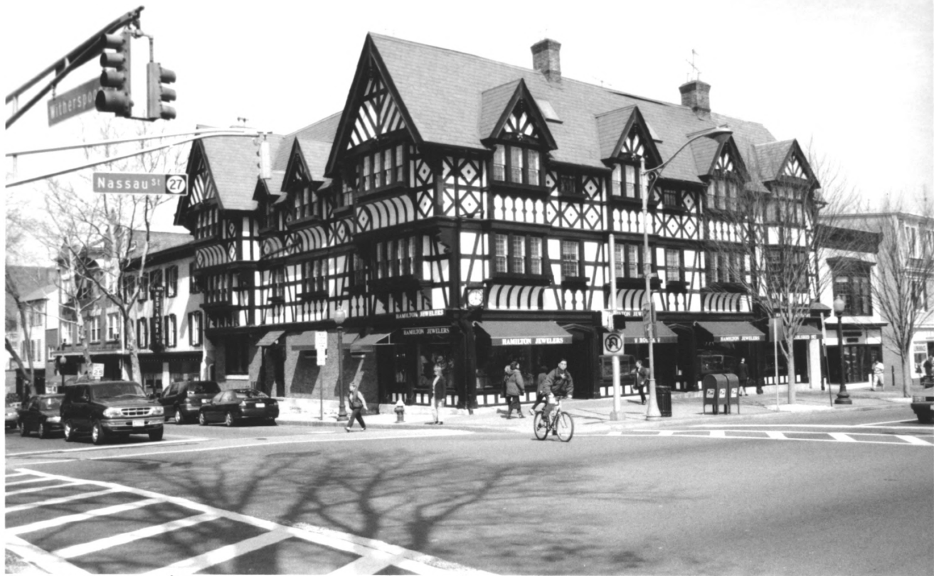
King's Highway (Upper Road, Lincoln Highway), NJ Mercer County
