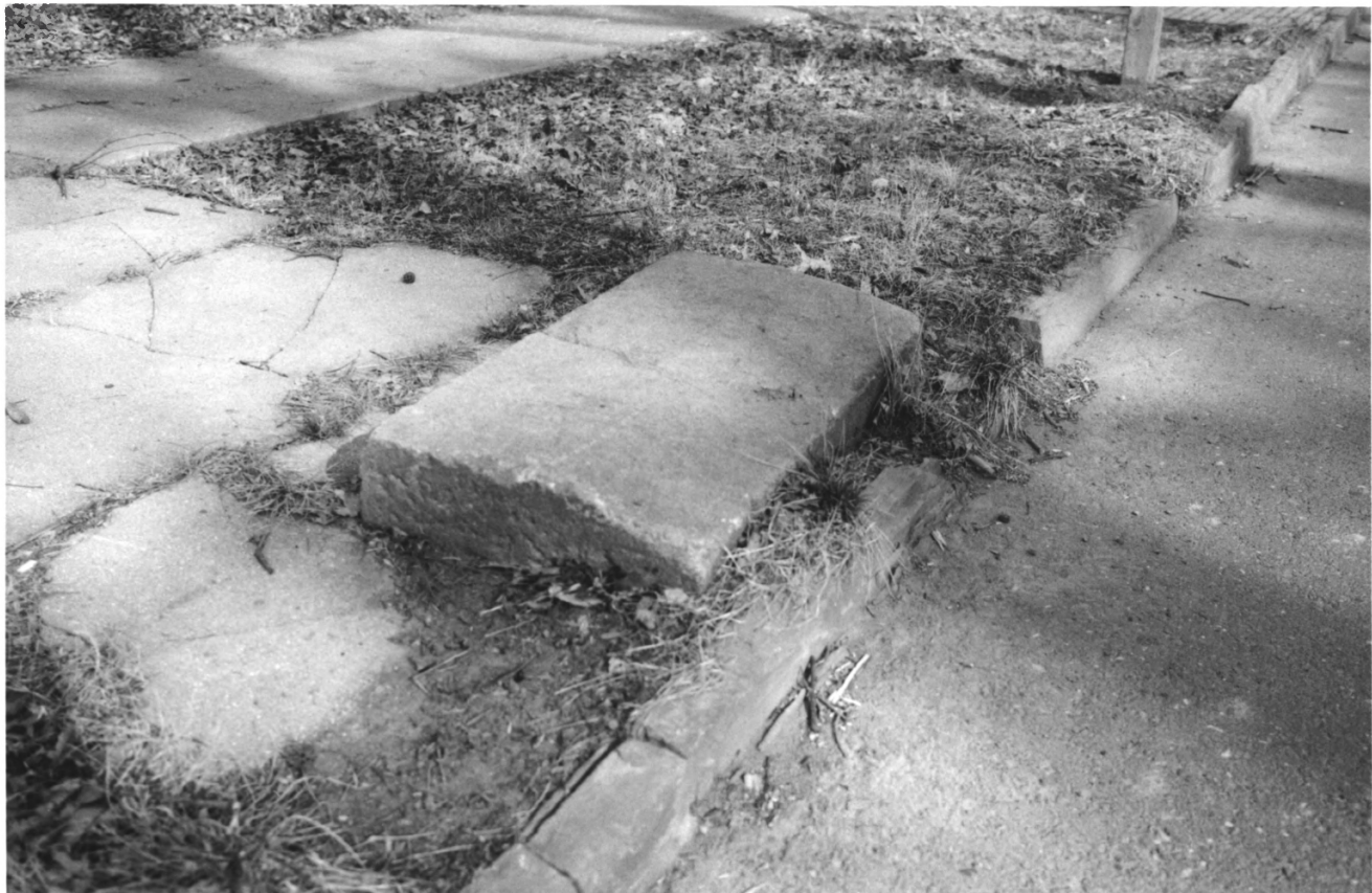
KING'S HIGHWAY (UPPER ROAD), LINCOLN HIGHWAY) NJ MERCER COUNTY 73 of 200
