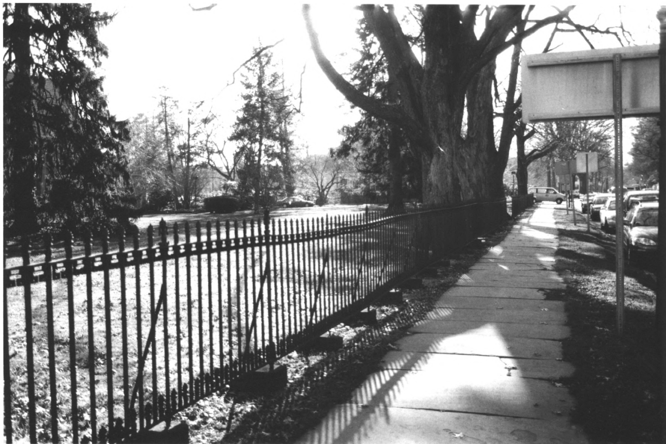
KING'S HIGHWAY (UPPER ROAD, LINCOLN HIGHWAY), NJ MERCER COUNTY 114 of 200
