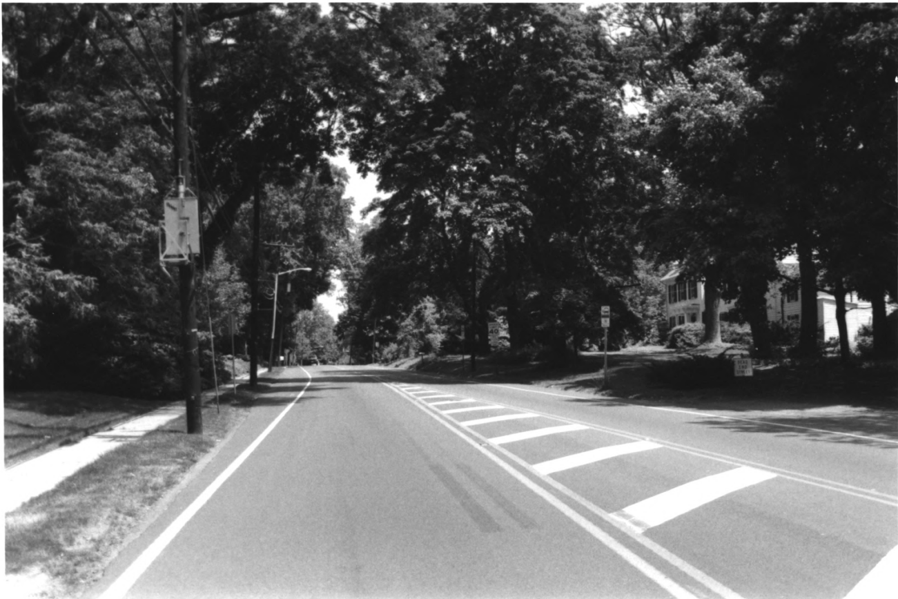
KING'S HIGHWAY (UPPER ROAD, LINCOLN HIGHWAY), NJ MERCER COUNTY 175 of 200
