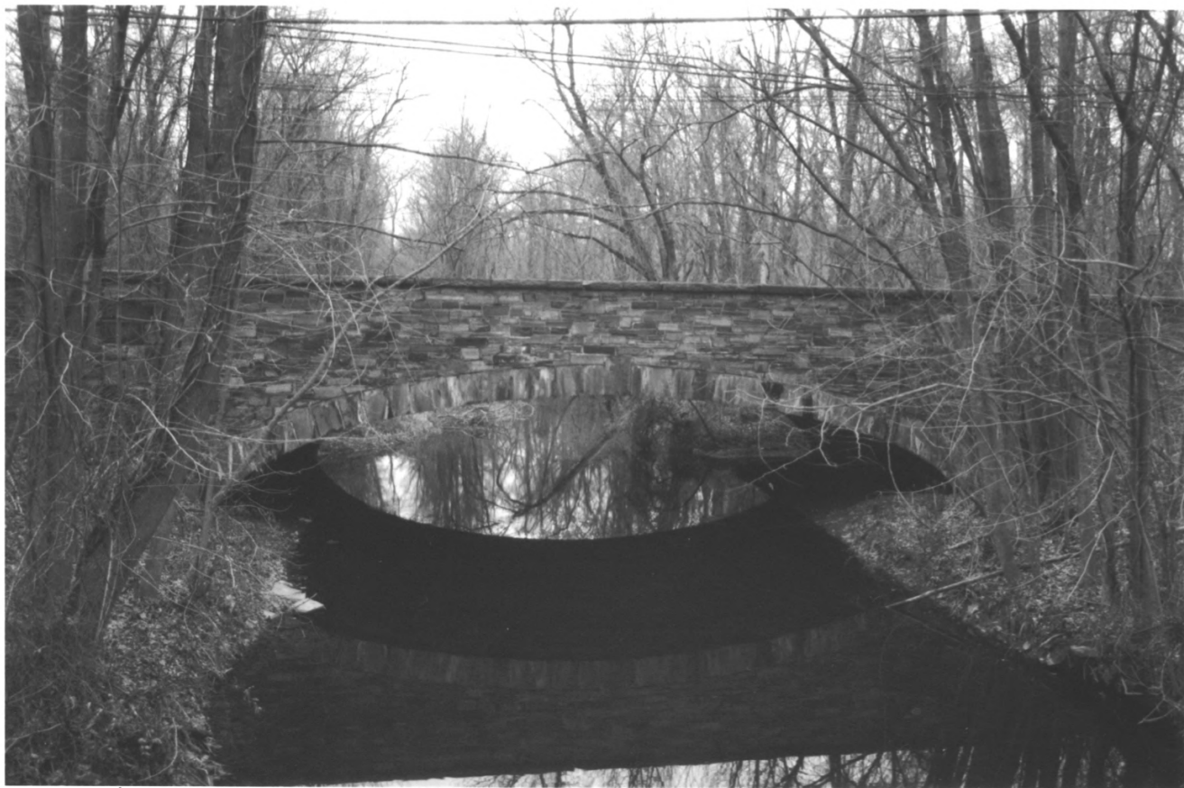
KING'S HIGHWAY (UPPER ROAD, LINCOLN HIGHWAY), NJ MERCER COUNTY 165 of 200
