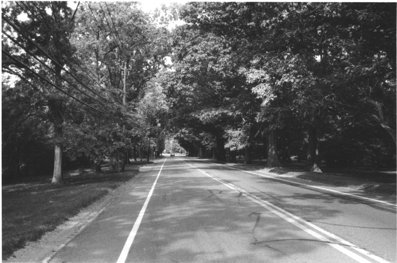
KING'S HIGHWAY (UPPER ROAD, LINCOLN HIGHWAY), NJ MERCER COUNTY 146 of 200
