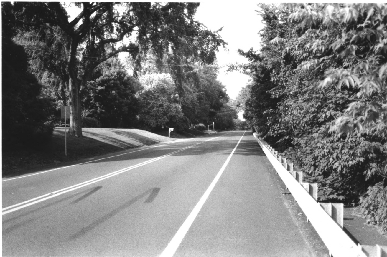
KING'S HIGHWAY (UPPER ROAD), LINCOLN HIGHWAY, NJ MERCER COUNTY 41 of 200
