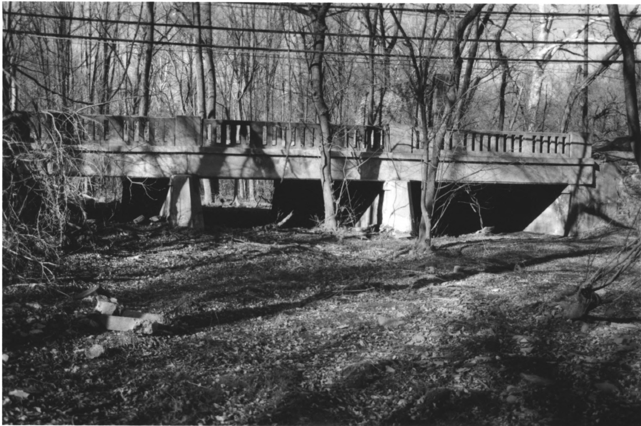
KING'S HIGHWAY (UPPER ROAD, LINCOLN HIGHWAY), NJ MERCER COUNTY 140 of 200
