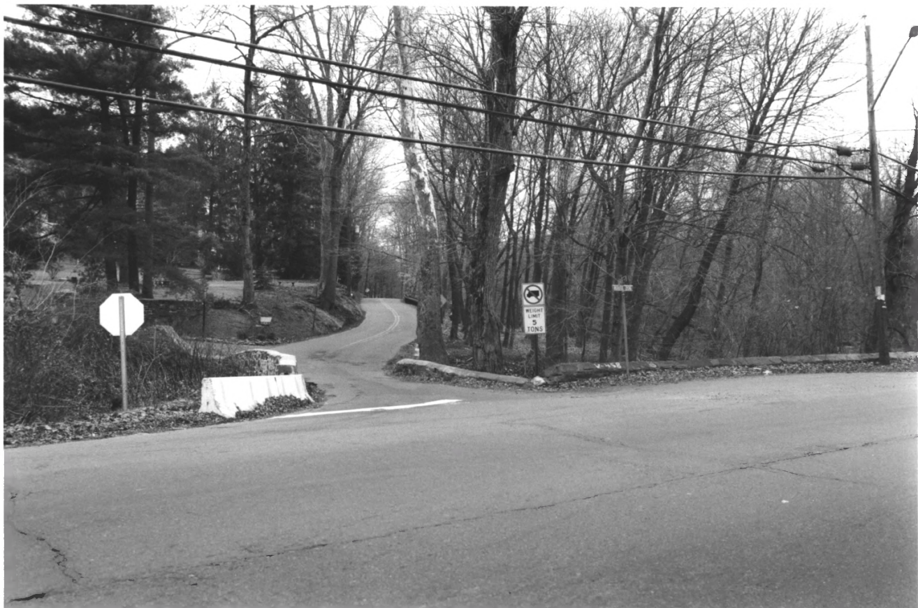
KING'S HIGHWAY (UPPER ROAD, LINCOLN HIGHWAY), NJ MERCER COUNTY, 133 of 200
