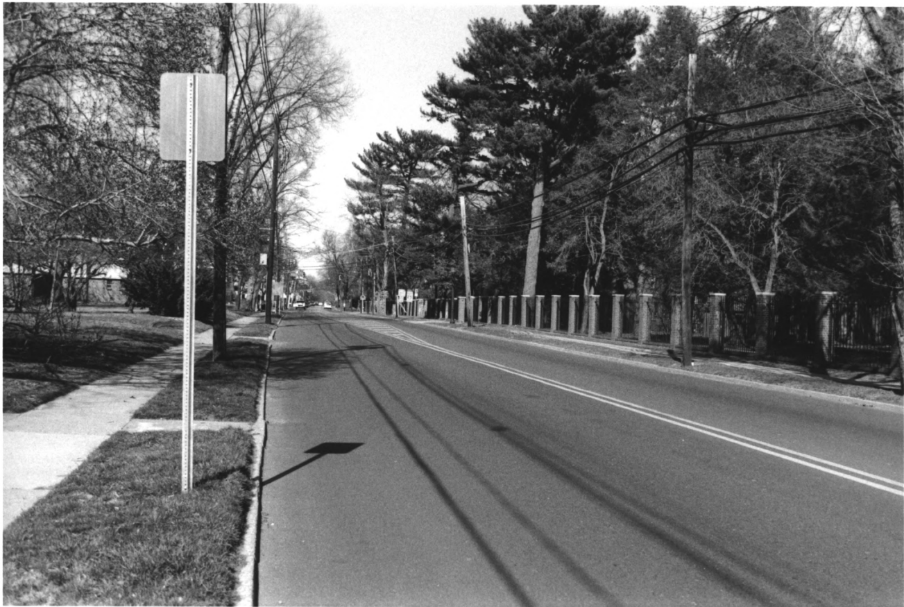
KING'S HIGHWAY (UPPER ROAD, LINCOLN HIGHWAY), NJ MERCER COUNTY 188 of 200
