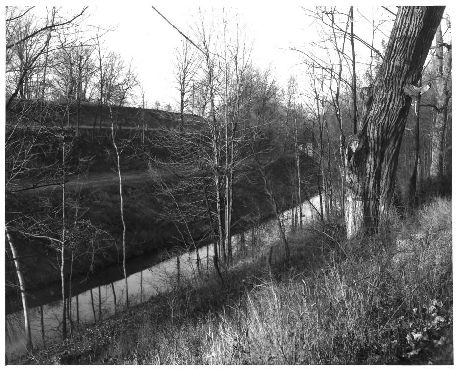
Miami and Erie Canal, "Deep:Cut," Ohio Route 66, south of Spencerville, Ohio. This tremendous cut for the Miami and Erie Canal is over a mile long and fifty-two feet deep at its deepest point.
