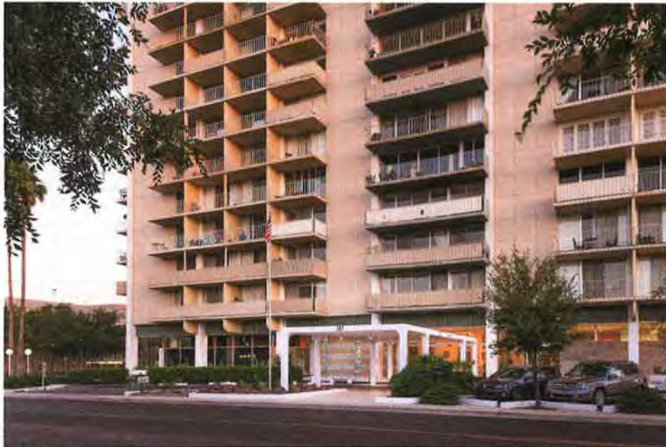
Figure 1: Base of the North elevation (façade) showing the porte-cochere in relation to the central entrance and the base of the building. The circular projection (detailed in Figure 2 below) appears to the left, and the glass wall of the base is visible. On the upper stories, note the cantilevered balconies and metal balustrades and balusters. (This image is also Photo 17, listed below)
