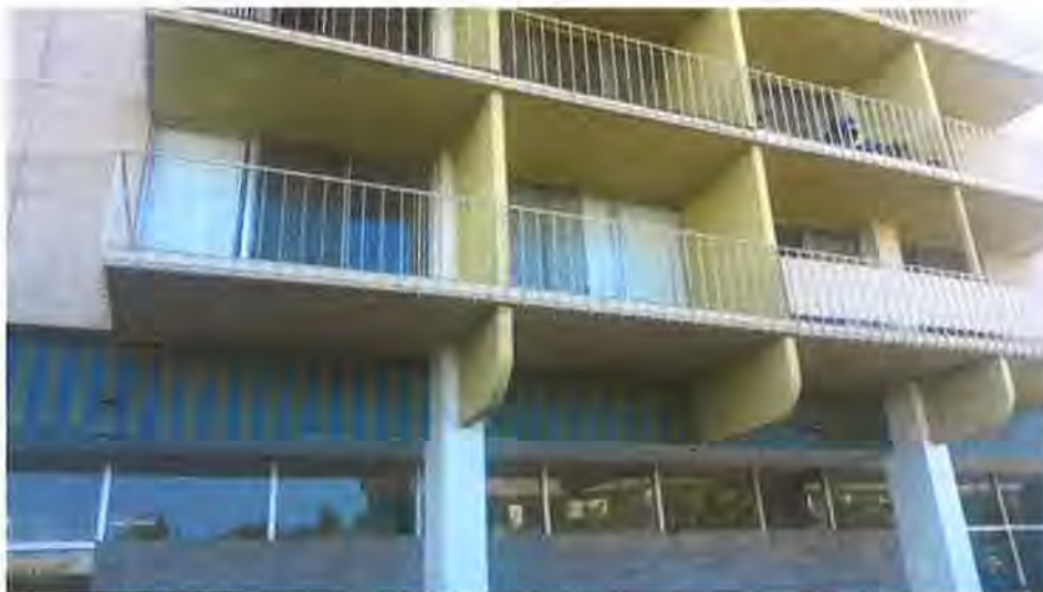
Figure 3: Blue glass mosaic band, situated at top of first story, and curved ends at the base of the vertical panels.
