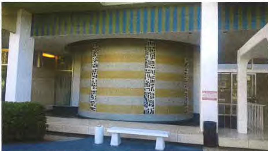
Figure 2: Circular projection from main façade, featuring mosaic tiles, and stained glass. This element, and the mosaic band above indicate the incorporation of art, in contrast to the austere nature of the overall design.
