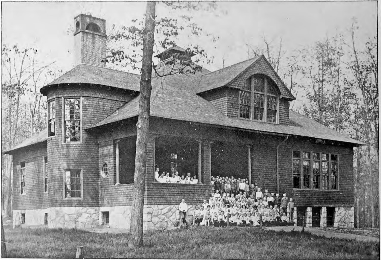
SCHOOL BUILDING: THREE SCHOOL ROOMS. AUDIENCE ROOM ON SECOND FLOOR
