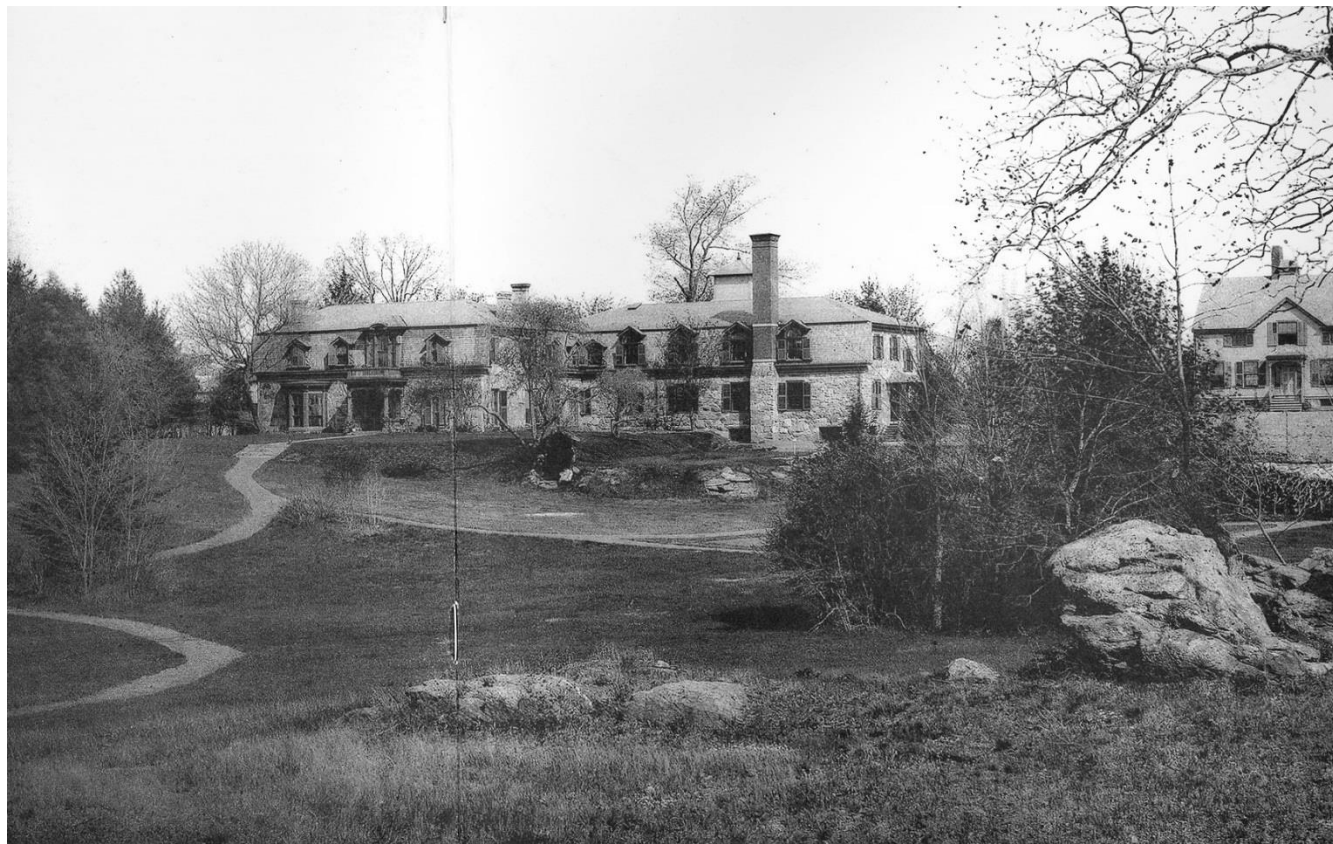
Figure 5 The earliest known photograph (c. 1890) of the State Home and School for Dependent and Neglected Children property showing the George W. Chapin House (left) after its conversion to a superintendent's residence and the completion of a wing addition to house a dining room and multi-purpose space for children. Cottage C (1885), the first wood-frame cottage purpose-built for the State Home and School, is seen to the right. This image also displays pathways and road systems which partially survive today. The boulder in the foreground is extant and provides a placemaker for the property.
