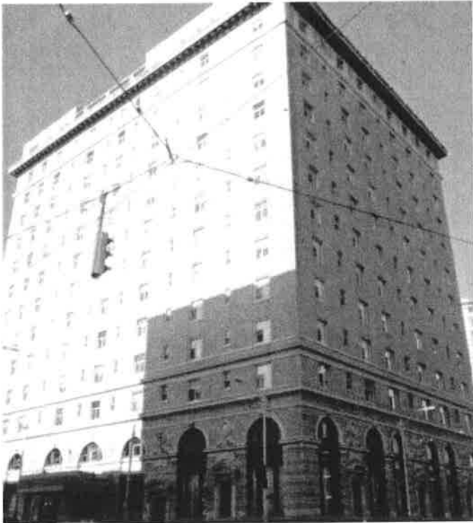
1989 view of the New Washington Hotel (1902 Second Ave, Seattle, WA, 1908), designed by Eames and Young. Source: Washington Information System for Architectural and Archaeological Records Data (WISAARD).
