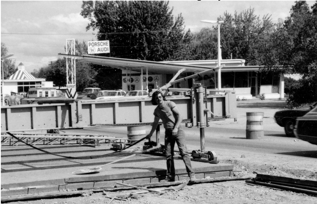
Courtesy Idaho Transportation Department Online Photograph Collection, SH443
