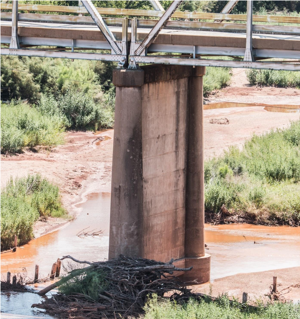
Photo 9 Concrete pier, taken from current U.S. 380 Bridge, facing south.
