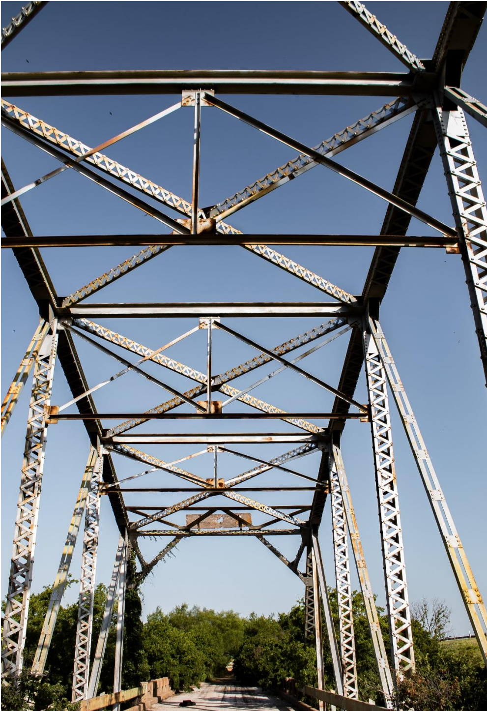
Photo 7 Easternmost span, facing west towards approach spans
