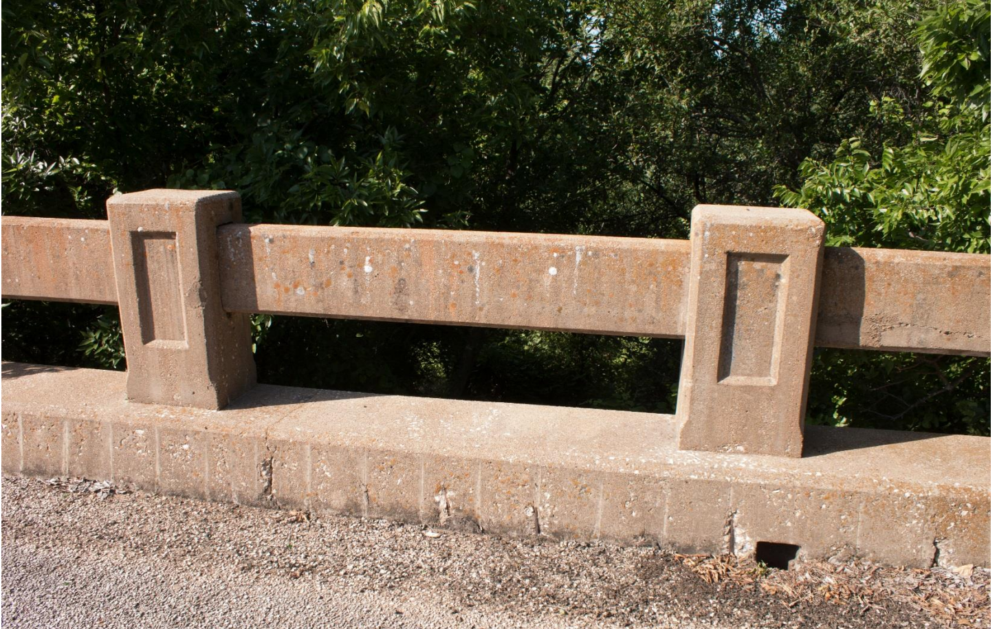
Photo 8 Typical approach span railing Camera facing south
