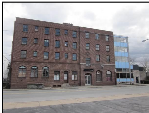
Figure 11. Hotel Oneida. Note 1960s addition on right.
