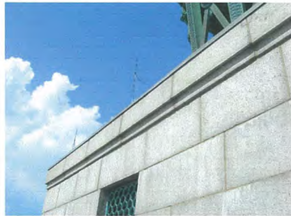
Fig. 64 – Lightning arresters on top of penthouse wall, looking northeast.
