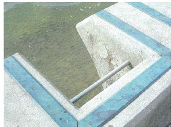
Fig. 21 – Access ladder built into south seawall, looking south
