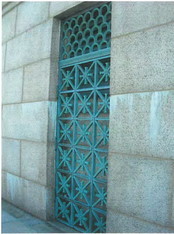
Fig. 61 – Typical vent opening and grillwork of exterior penthouse walls, looking southwest.
