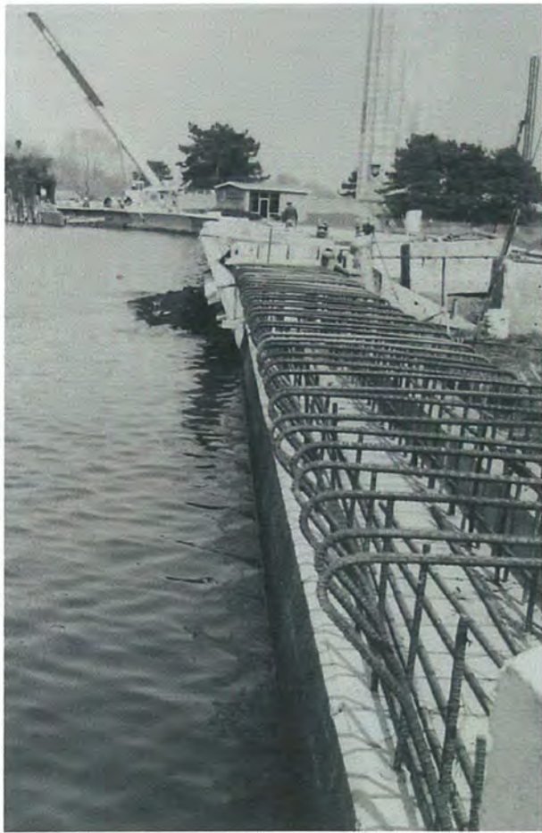
Fig. 136 – North seawall reconstruction, c. 1978, looking southeast. Photo courtesy of the Perry's Victory and International Peace Memorial archives.
