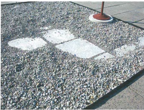
Fig. 41 – Ongoing rehabilitation of granite pavers on upper plaza, looking southwest. Note hard black plastic borders and pebbled surface.
