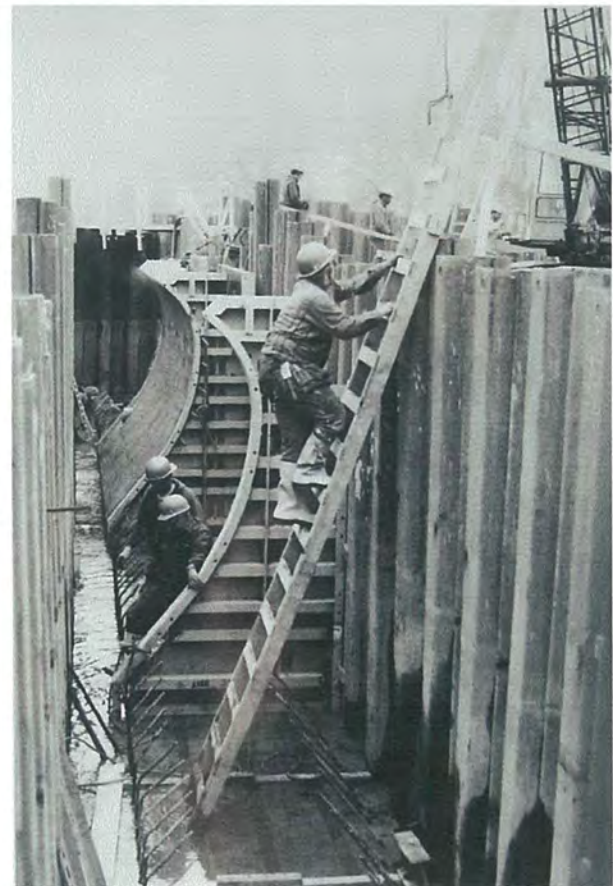
Fig. 139 – Placing forms for south seawall reconstruction, c. 1977-78. Photo courtesy of the Perry's Victory and International Peace Memorial archives.
