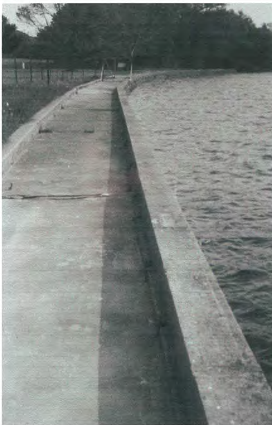
Fig. 19 – South seawall, c. 1977, before reconfiguration and reconstruction, looking northeast. Note that a wall has been added on the water side of the sidewalk. Photo courtesy of Perry's Victory and International Peace Memorial archives.
