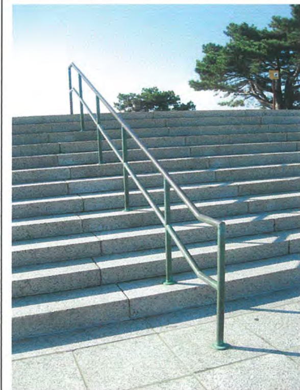
Fig. 36 – Typical brass pipe handrails on plaza stairways, looking south.
