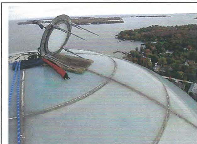
Fig. 140 – View of exterior of lantern roof, c. 2007, looking northeast. Shows original plate glass panels and access hatch. Photo from Wiss, Janney, Elstner Associates, Exterior Conditions Assessment , p. 43.
