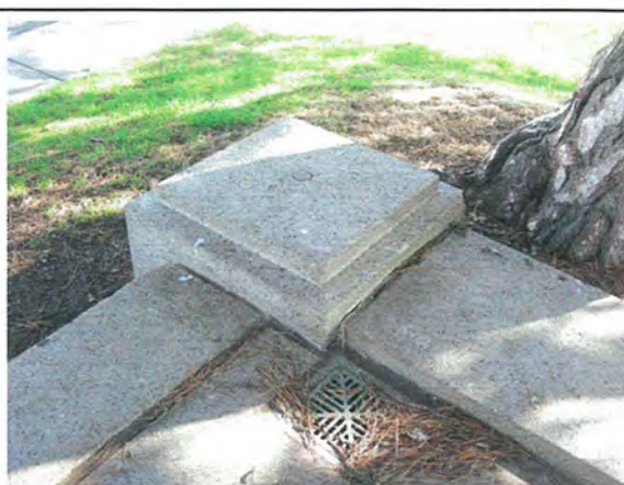
Fig. 37 – Granite curbing and brass drain cover in north corner of lower plaza, looking north.
