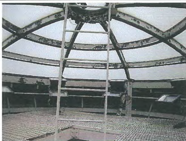
Fig. 141 – Interior view of lantern roof, c. 2007, before replacement of damaged panels. Photo from Wiss, Janney, Elstner Associates, Exterior Conditions Assessment , p. 42.
