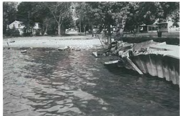
Fig. 132 – Damage to south seawall from 1972-73 storms, looking west. Delaware Avenue at end of seawall. Photo courtesy of the Perry's Victory and International Peace Memorial archives.
