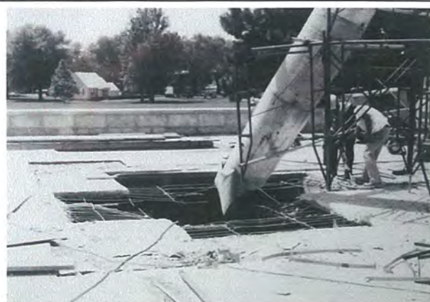
Fig. 142 – Repairing formed reinforced concrete of upper plaza, c. 1982. Photo courtesy of the Perry's Victory and International Peace Memorial archives.
