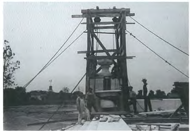
Fig. 109 – Mounting granite urn, c. 1915. Photo courtesy of the Perry's Victory and International Peace Memorial archives.
