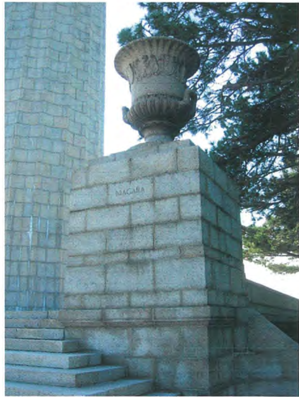
Fig. 43 – Typical granite-faced pedestal supporting granite urn, looking east.
