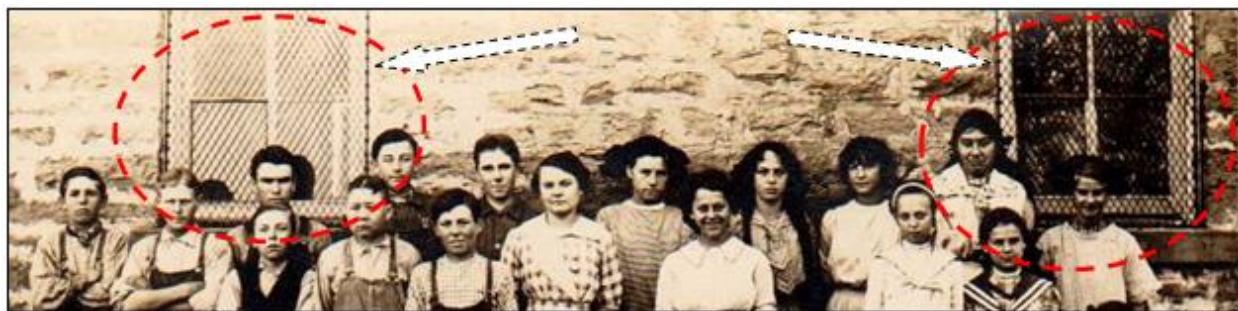
Figure 4: Oak Grove School 1912. Arrows point to window screens.
