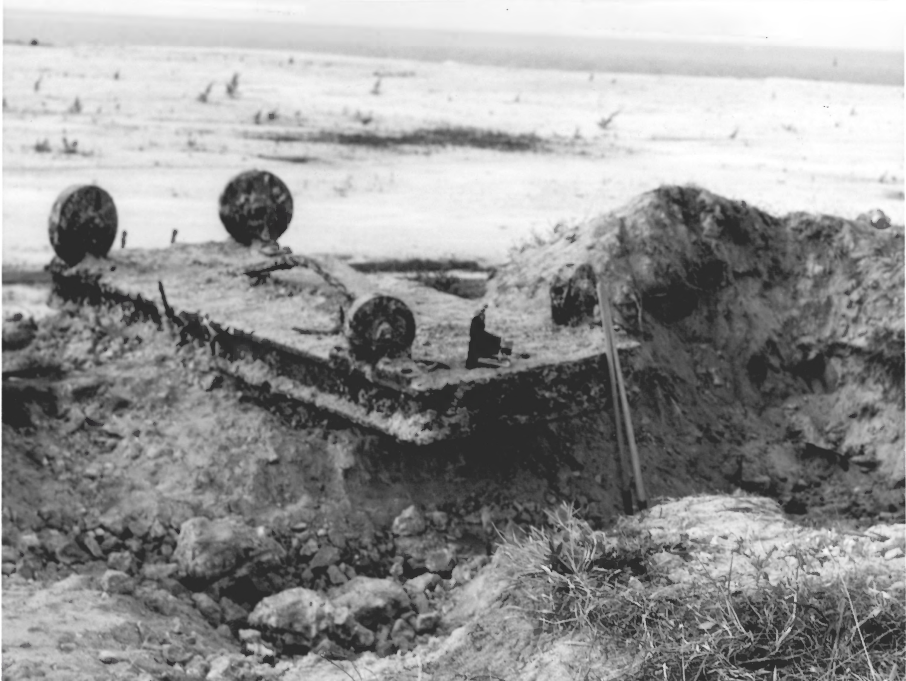
FIRST BARBETTER GUN CARRIAGE TO BE BROUGHT TO LIGHT IN SOUTH CHANNEL WALL EXCAVATION ---OCEAN IS IN BACKGROUND
