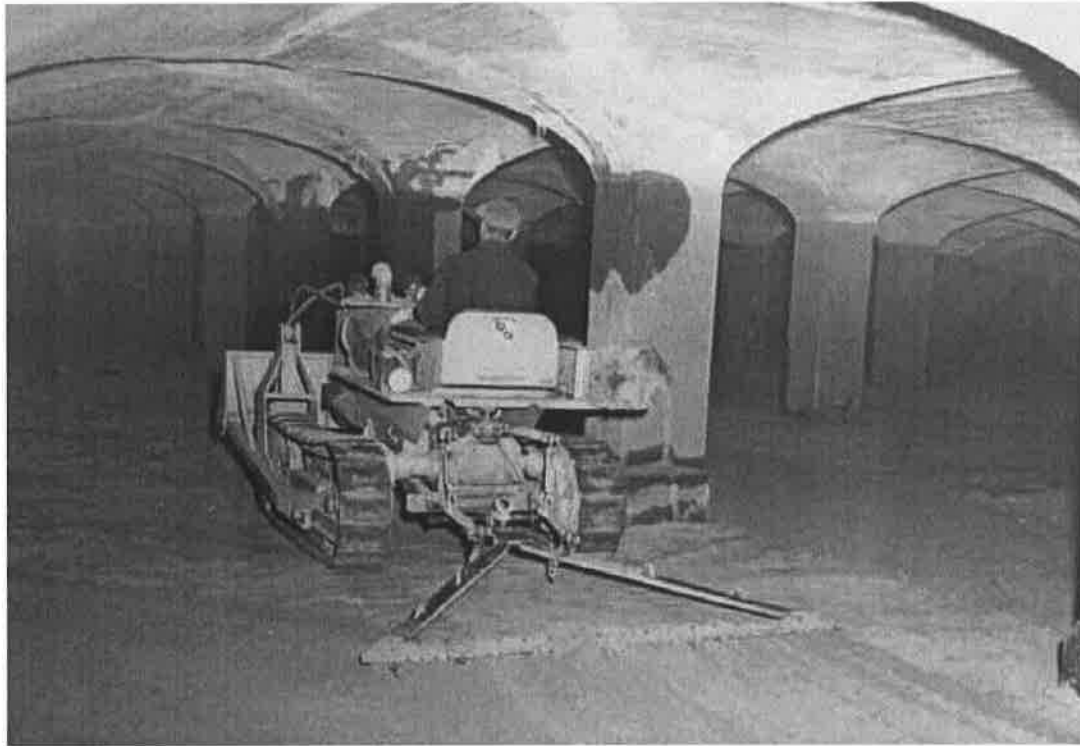
Tractor and filter rake pulverizing the filter sand surface and filter operation (c. 1944) Courtesy of the Archives of the Washington Aqueduct
