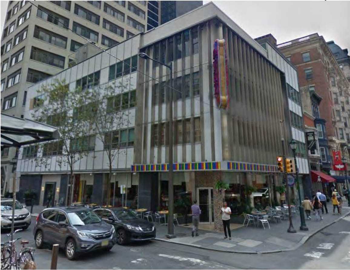
Figure 22 – Cayuga Federal Savings & Loan Building, Philadelphia, PA (Philip Mastrin, 1960).
