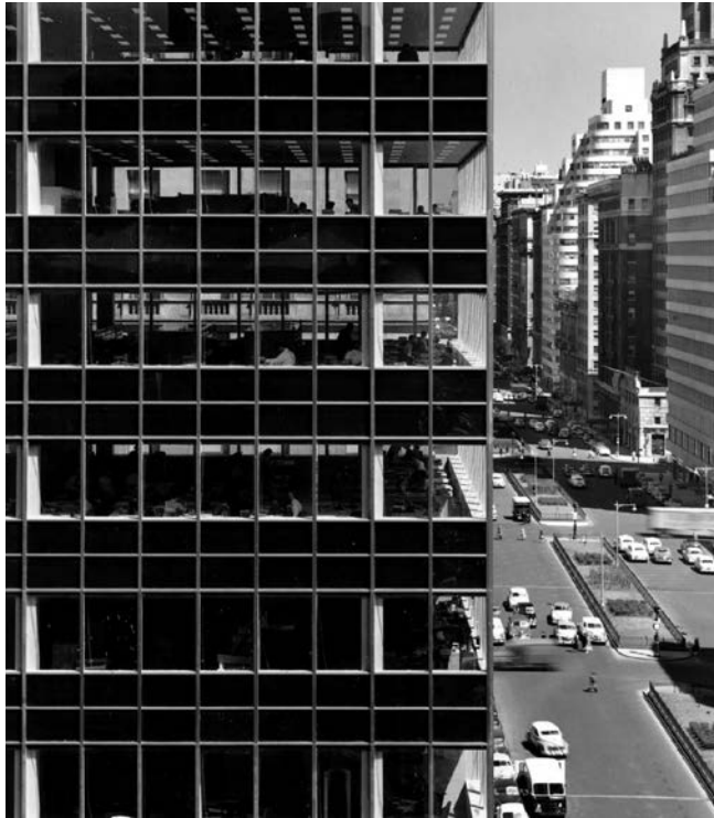
Figure 20 – Detail of the façade of Lever House, New York City (Skidmore, Owings and Merrill, 1952).
