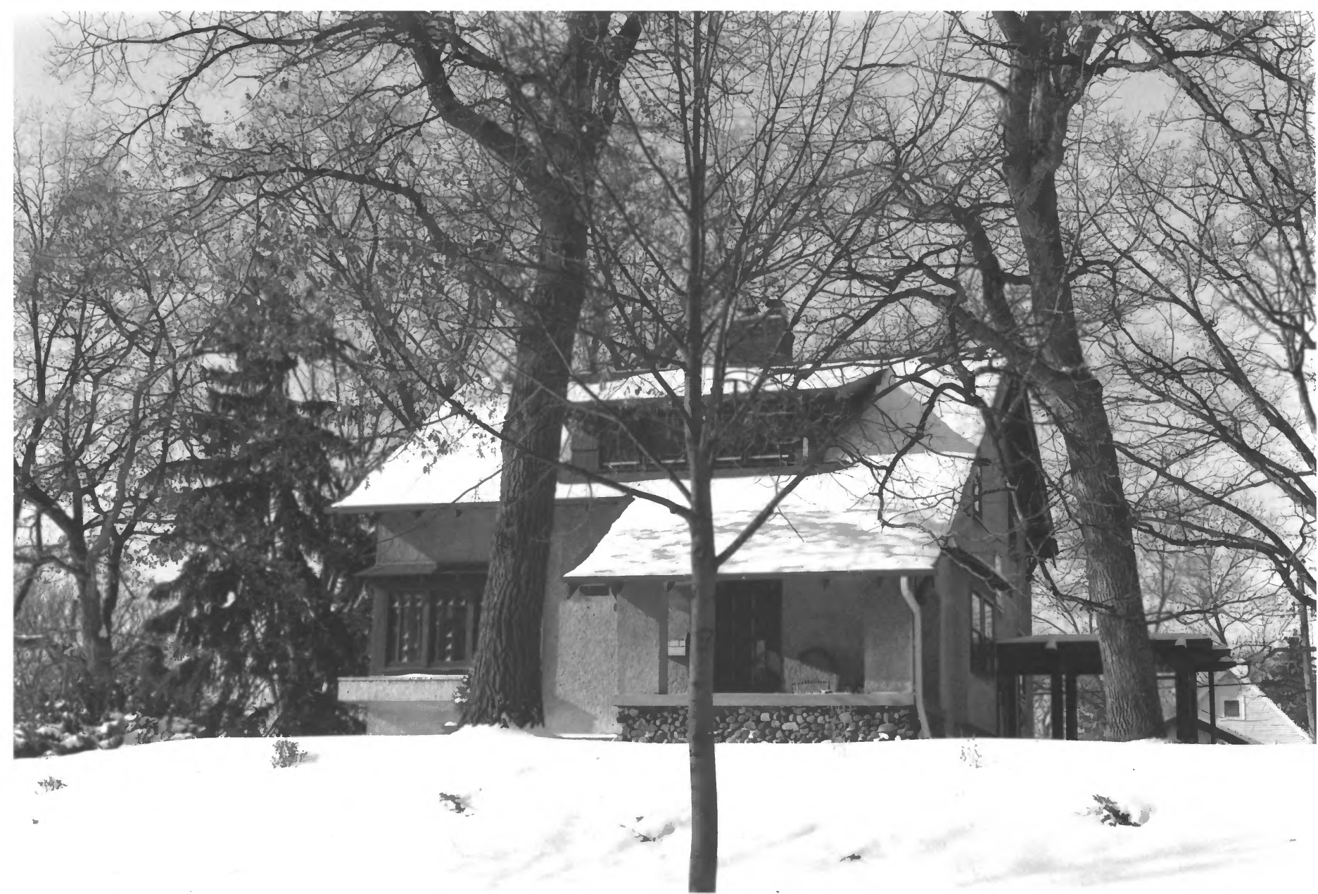
Fournier, Lawrence A. and Mary, House 3505 Sheridan Avenue North Minneapolis, Hennepin Co. 012214-9A/10
